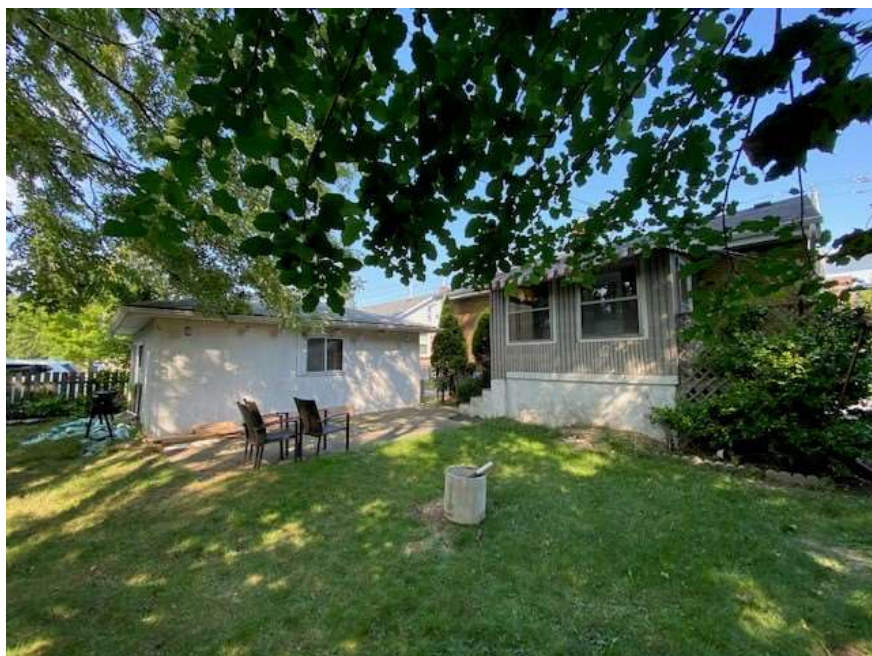
Image 3: 1455 Oxford Street East – rear view of residence, garage and yard (August 24, 2020)
