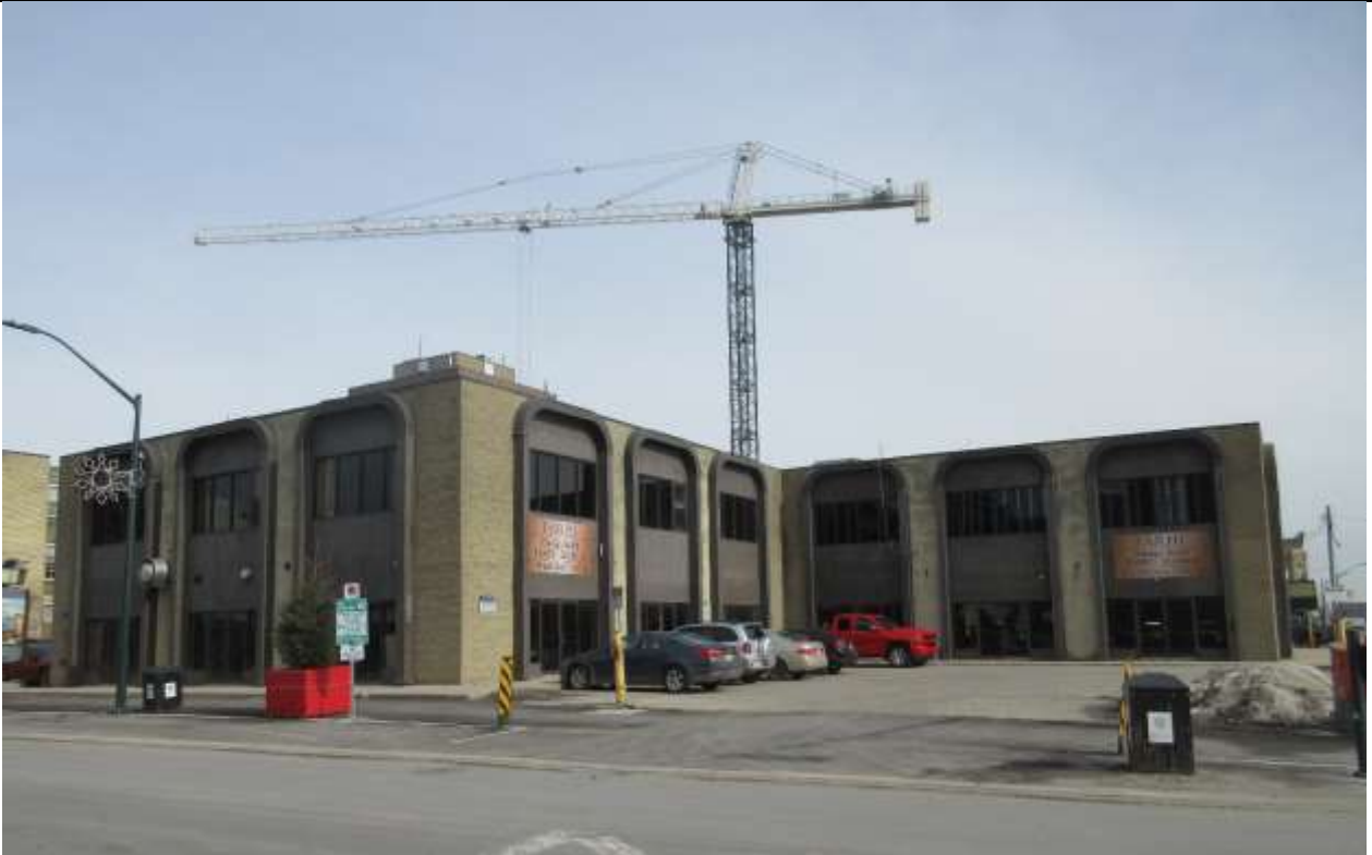
Image 1: North east view of existing building and parking on the property as seen from intersection of Talbot and York Streets (2019-02-14)
