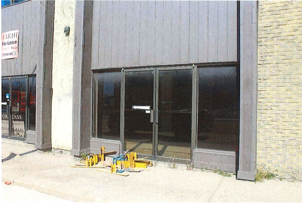
Image 7: Storefront view showing 120 York Street from the south, September 2019
