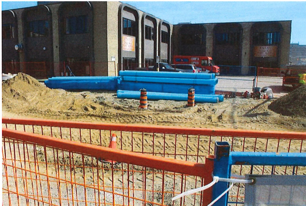
Image 4: View showing 120 York Street from the West, September 2019
