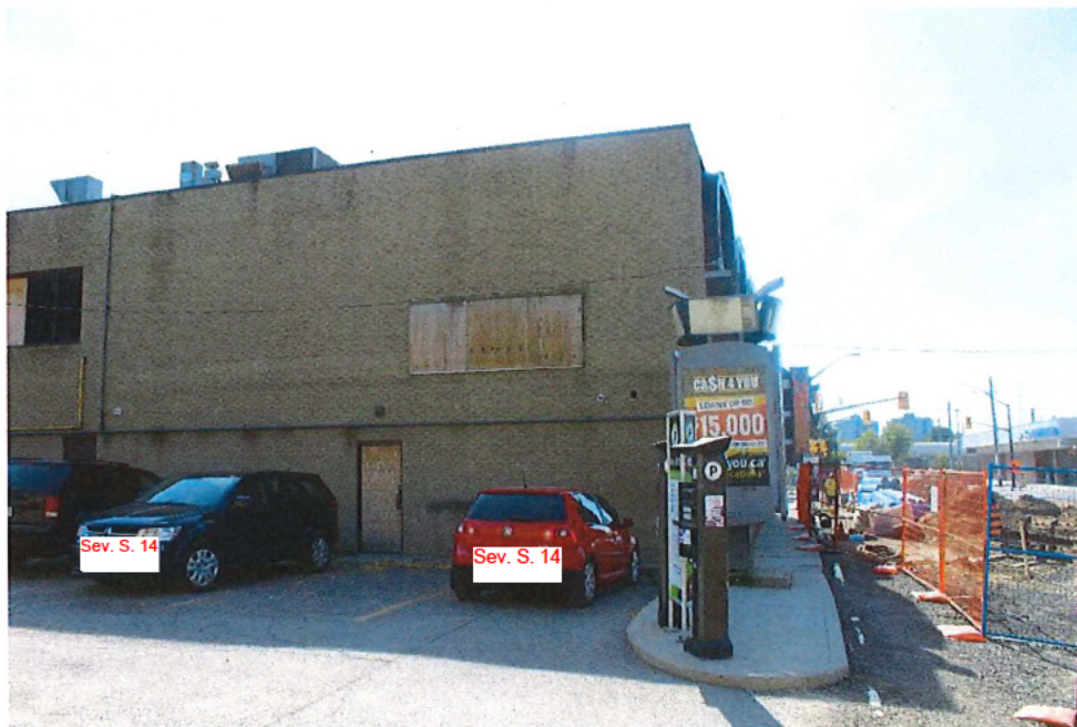
Image 2: View showing 120 York Street from the north, September 2019
