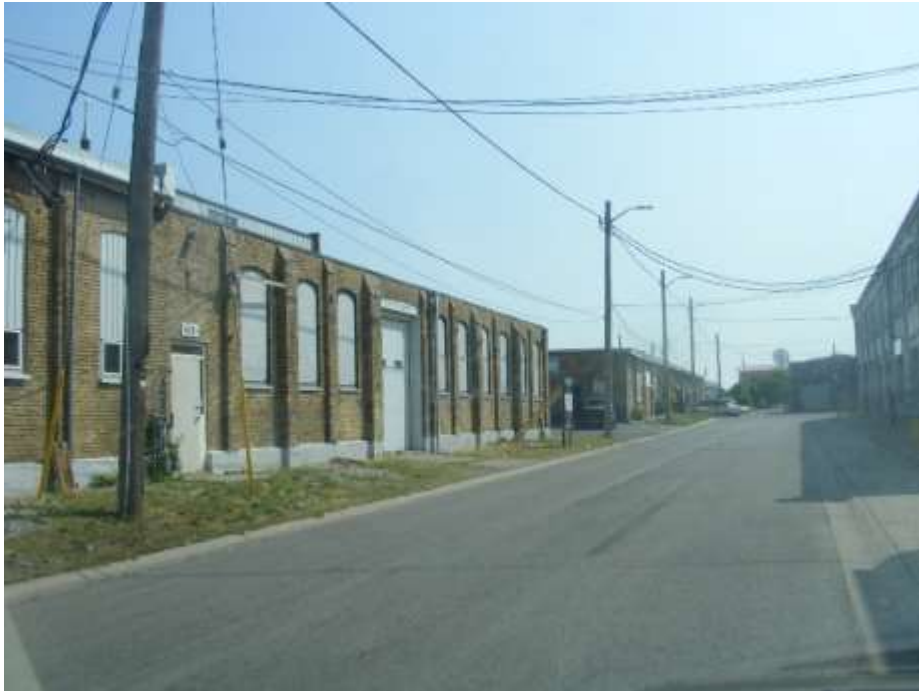
Photo 3 – Door on Cabell Street
