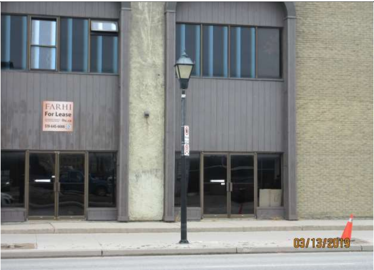
Image 2: Detail of Talbot Street façade of building on the property, view facing east (2019-03-13)
