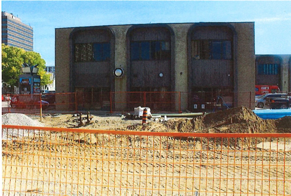
Image 3: View showing 120 York Street from the West, September 2019
