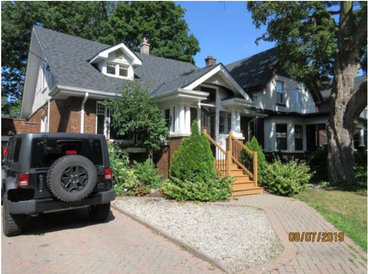
Image 2: Photograph of the property at 59 Wortley Road, showing the altered front steps.
