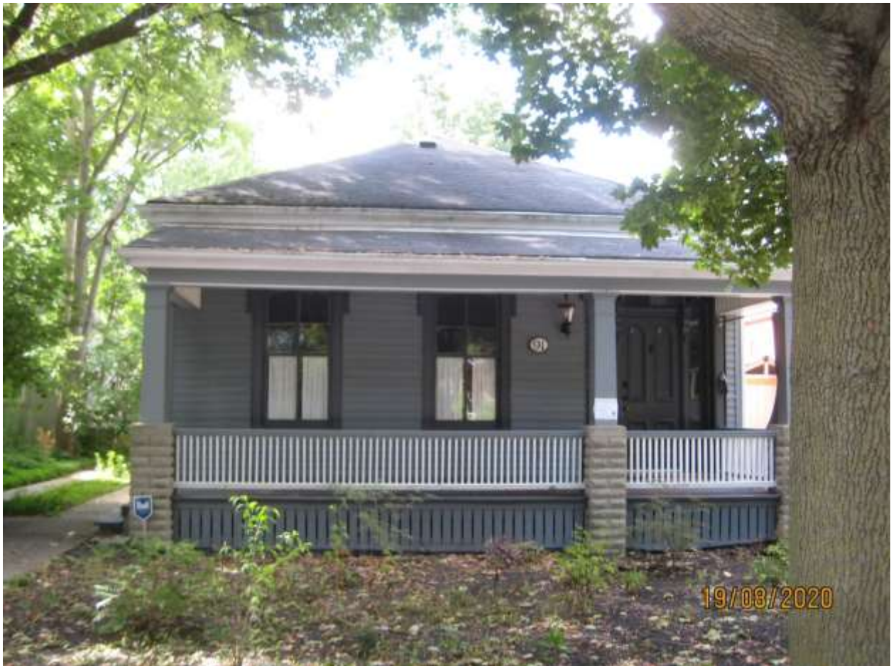
Image 4: Photograph showing the existing conditions of the dwelling at 91 Bruce Street in the Wortley Village-Old South Heritage Conservation District. Note, the railing on the right side of the photograph is proposed to be removed as a part of the proposed porch restoration.
