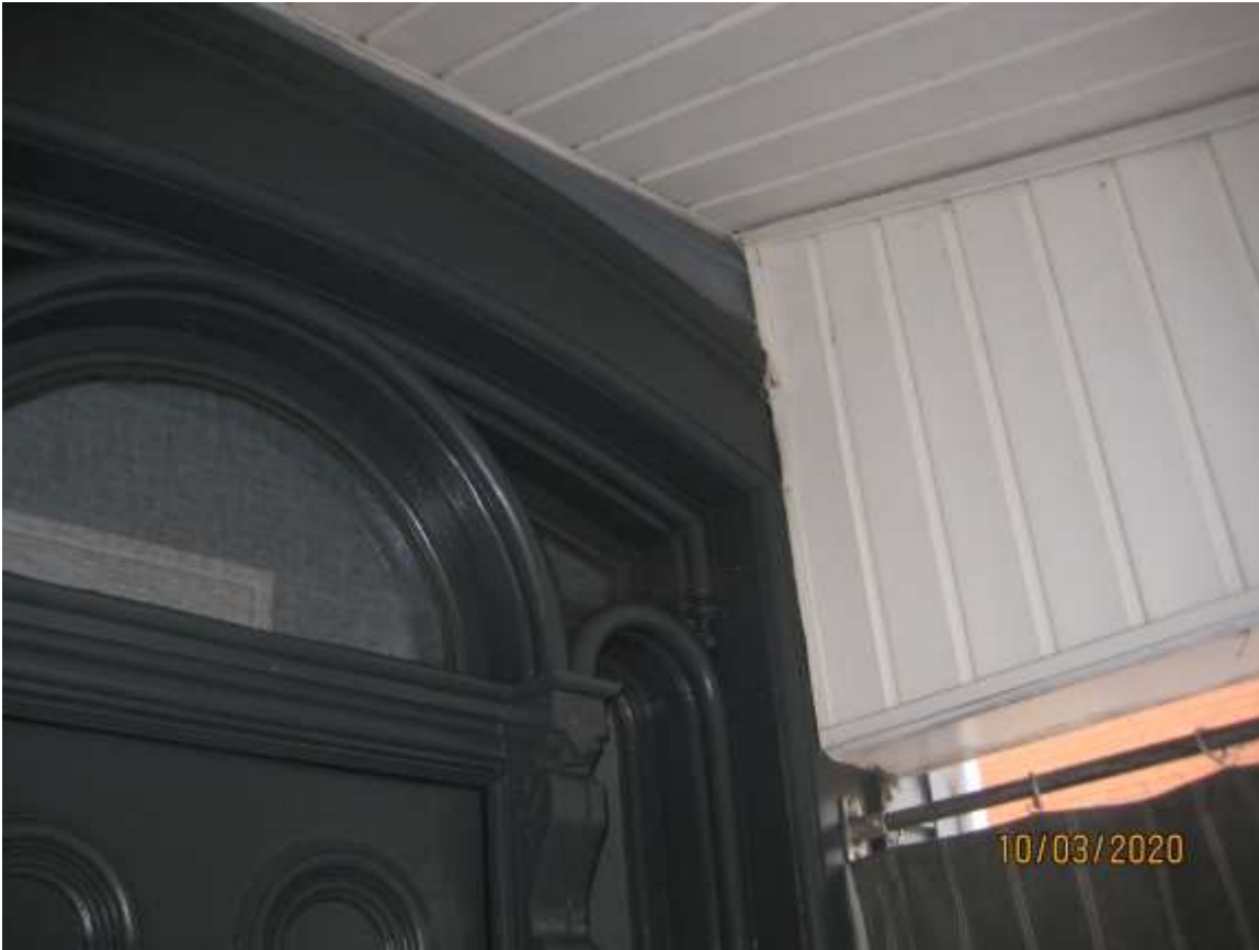
Image 9: Detail showing the existing conditions of the London Doorway. Note, the trim of the doorway has been previously altered with the installation of the porch ends. The Heritage Alteration Permit application seeks to restore the porch ends and porch ceiling in a manner that exposes the trim of the doorway and allows for the future restoration of the London Doorway.
