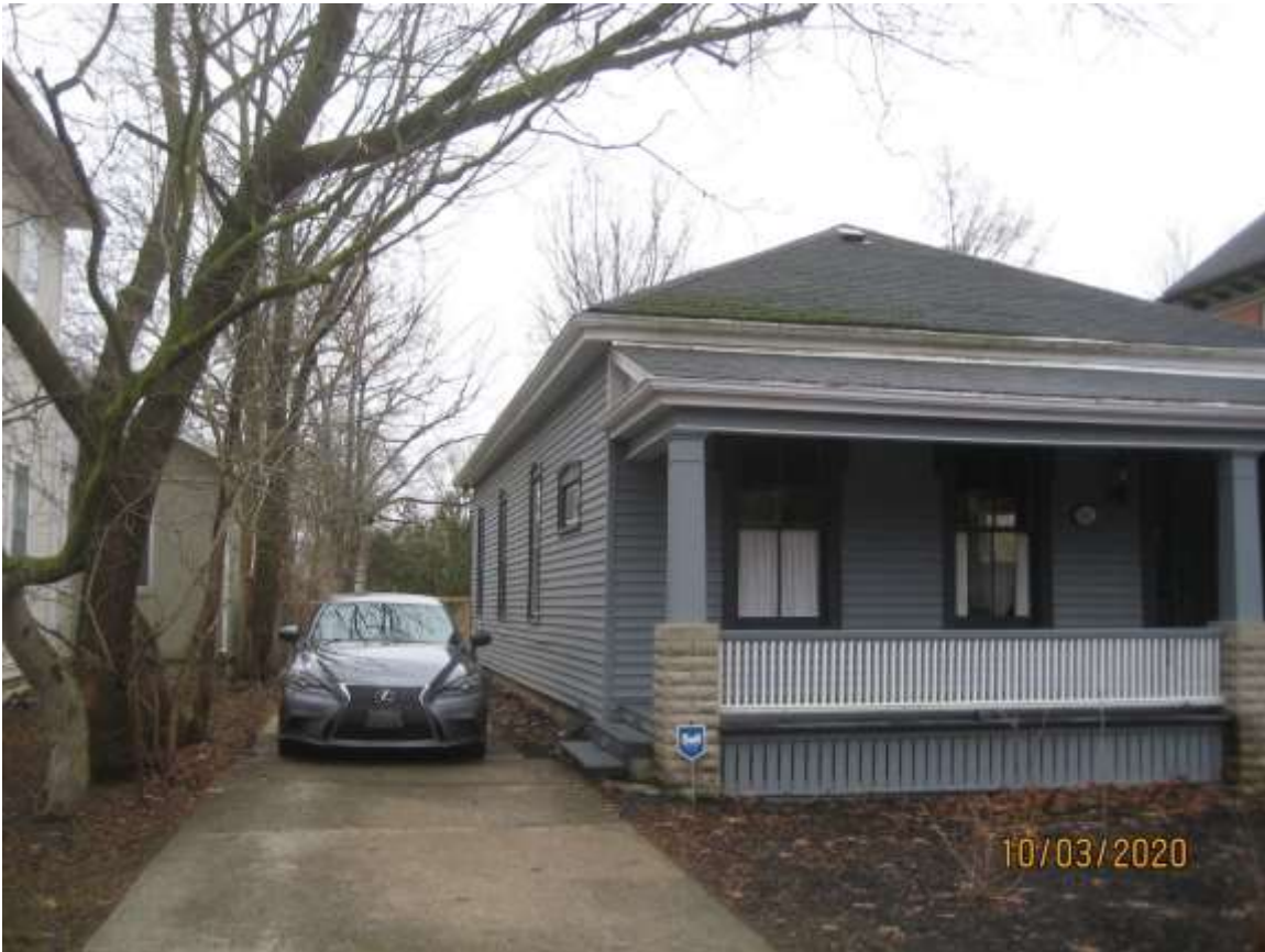
Image 8: Photograph showing the front (north) and side (east) facades of the dwelling as visible from the sidewalk on the south side of Bruce Street.
