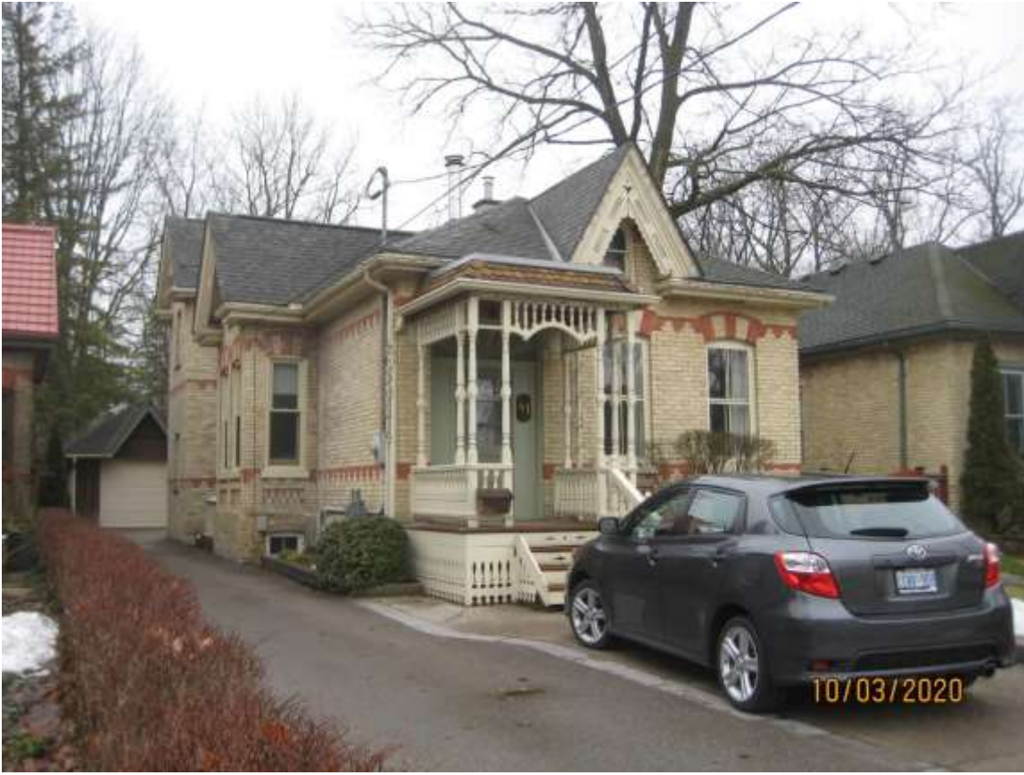
Image 11: Photograph of the dwelling located at 41 Bruce Street in the Wortley Village-Old South Heritage Conservation District, showing an example of a rear addition on single storey cottage.
