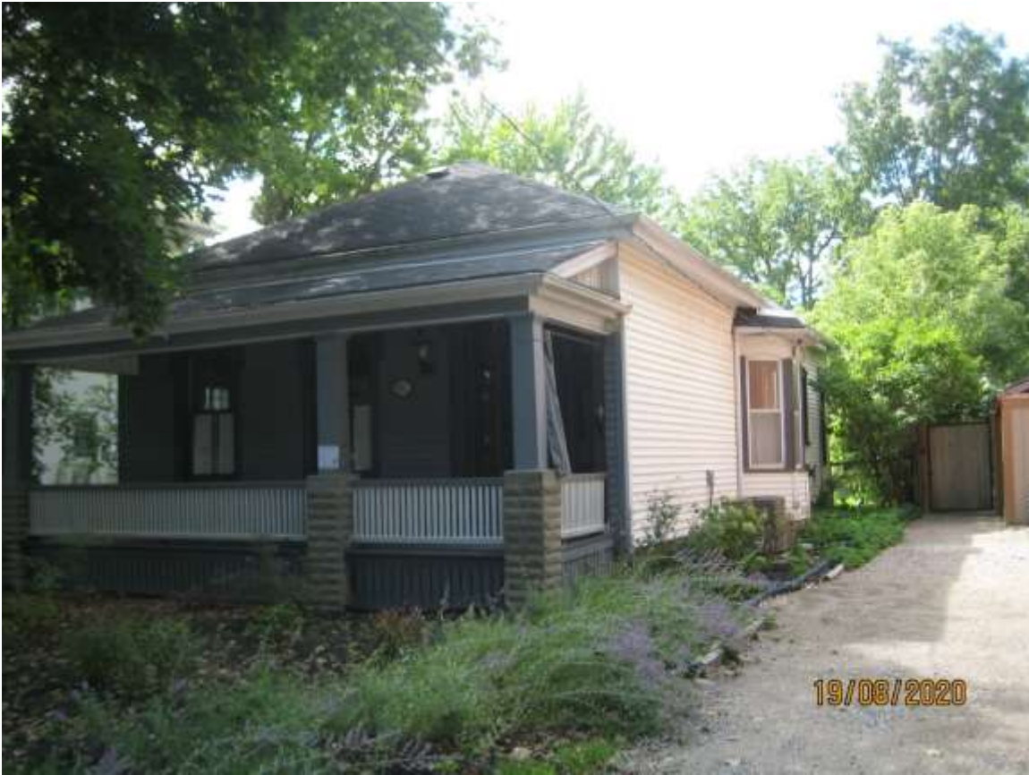
Image 5: Photograph showing the front (north) and side (west) facades of the dwelling, showing its existing conditions and various vinyl siding.
