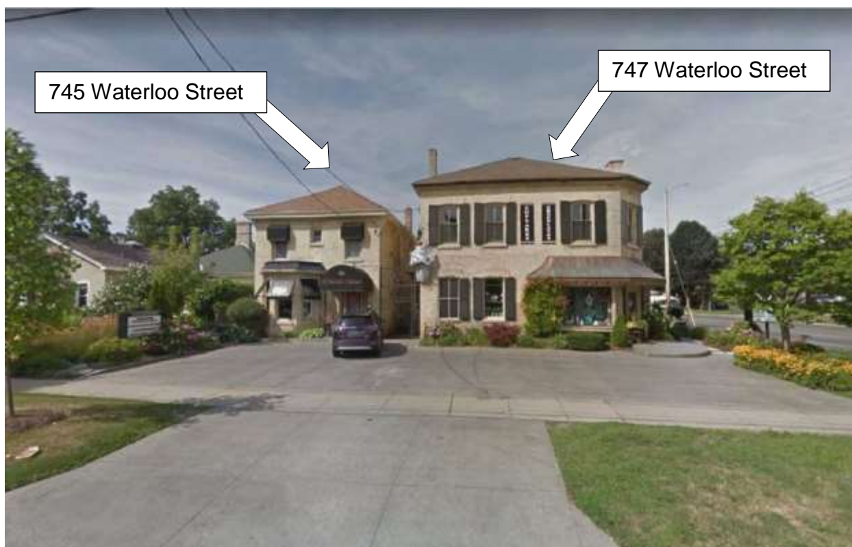
Photo of subject site as shown in September 24, 2018 Staff report to PEC
