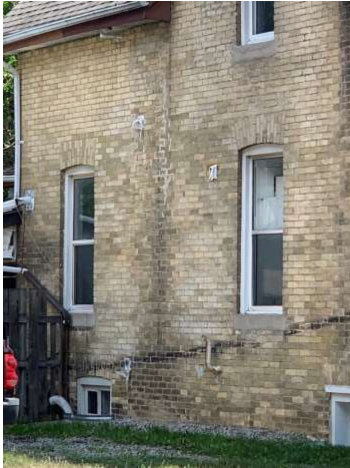
Image 7: Photograph submitted as a part of the Heritage Alteration Permit application for the property at 512 English Street, showing voussoir and sill details on the north façade that will be installed on the west façade.
