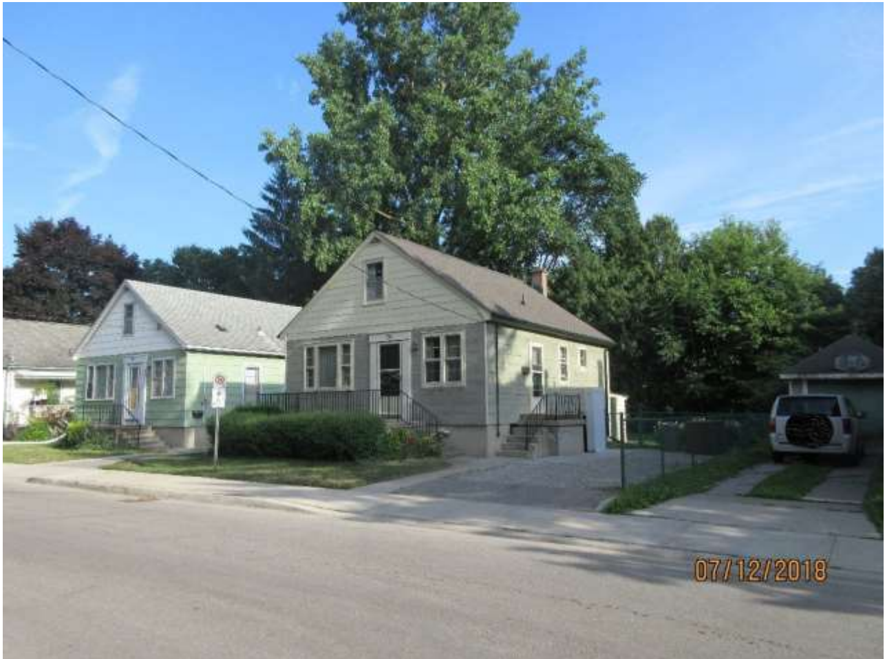
Image 1: View of the north (main) and west elevations of the dwelling located at 70 Rogers Avenue on July 12, 2018 (prior to alterations).
