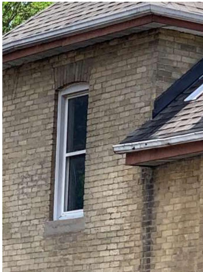
Image 6: Photograph submitted as a part of the Heritage Alteration Permit application for 512 English Street, showing windows on the north façade of the dwelling. The voussiors on this façade will be replicated on the west façade of the dwelling.
