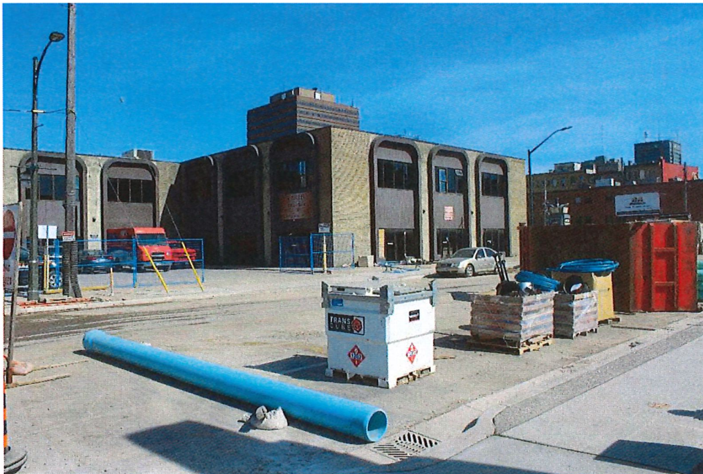
Image 6: View showing 120 York Street from the south, September 2019
