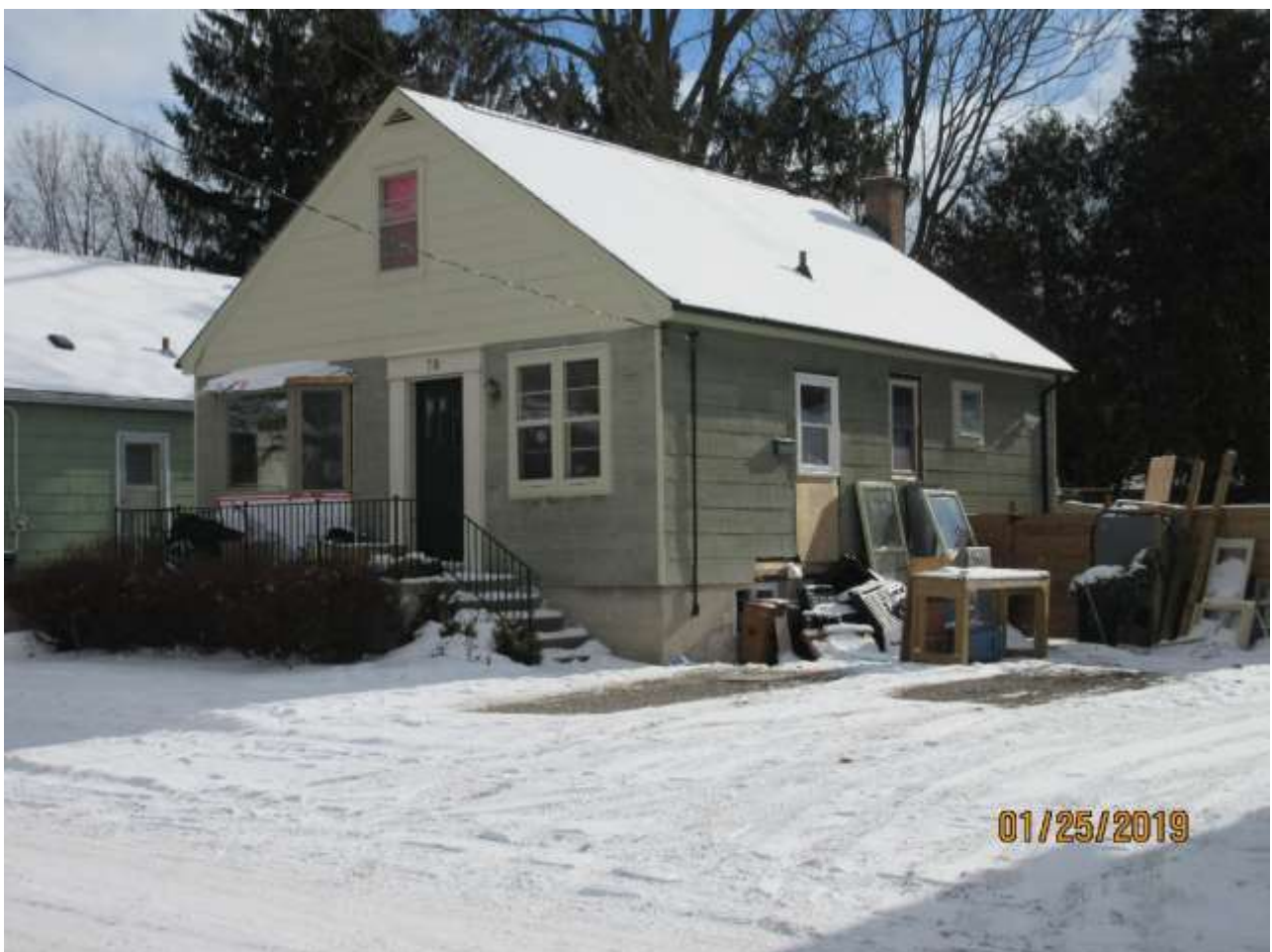
Image 2: Photograph showing the unapproved alterations to the property at 70 Rogers Avenue underway on January 25, 2019.
