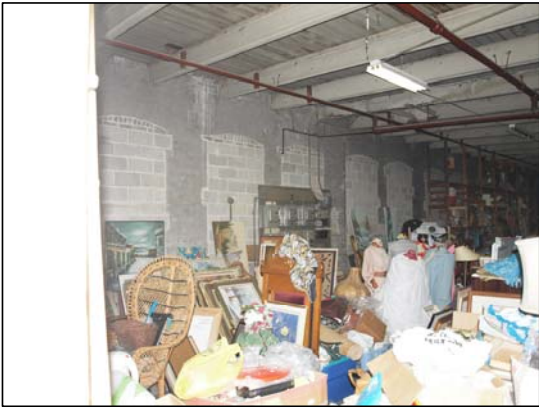
Former exterior wall - 1920's portion
