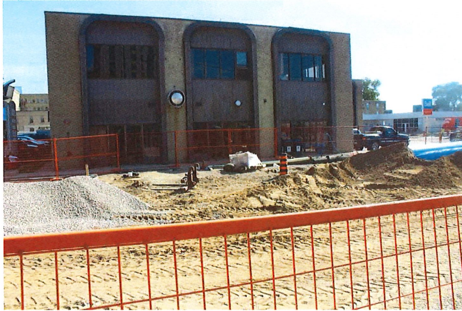
Image 1: View showing 120 York Street from the West, September 2019
