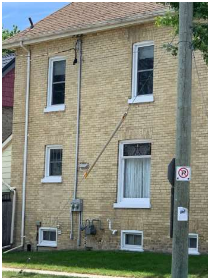
Image 8: Photograph submitted as a part of the Heritage Alteration Permit application for the property at 512 English Street, showing the property located at 519 English Street, within the Old East Heritage Conservation District. The property was cited in the Heritage Alteration Permit application as an example of a similar property demonstrating the voussoirs and sills to be installed at 512 English Street.
