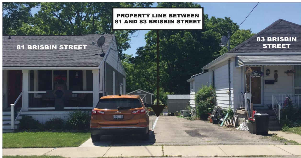
Figure 4: The existing shared driveway, looking west toward 81 and 83 Brisbin Street. The residents have painted a white line on the driveway demarcating ownership.
