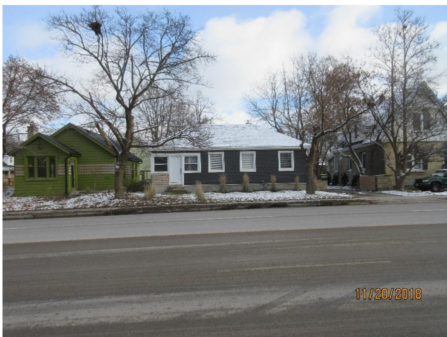
Image 3: Photograph of the property at 78 Wellington Road.
