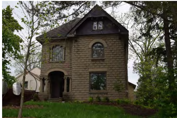
Plate 22: North façade, looking south
