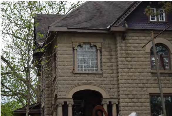
Plate 25: Second storey opaque glass block window, looking south
