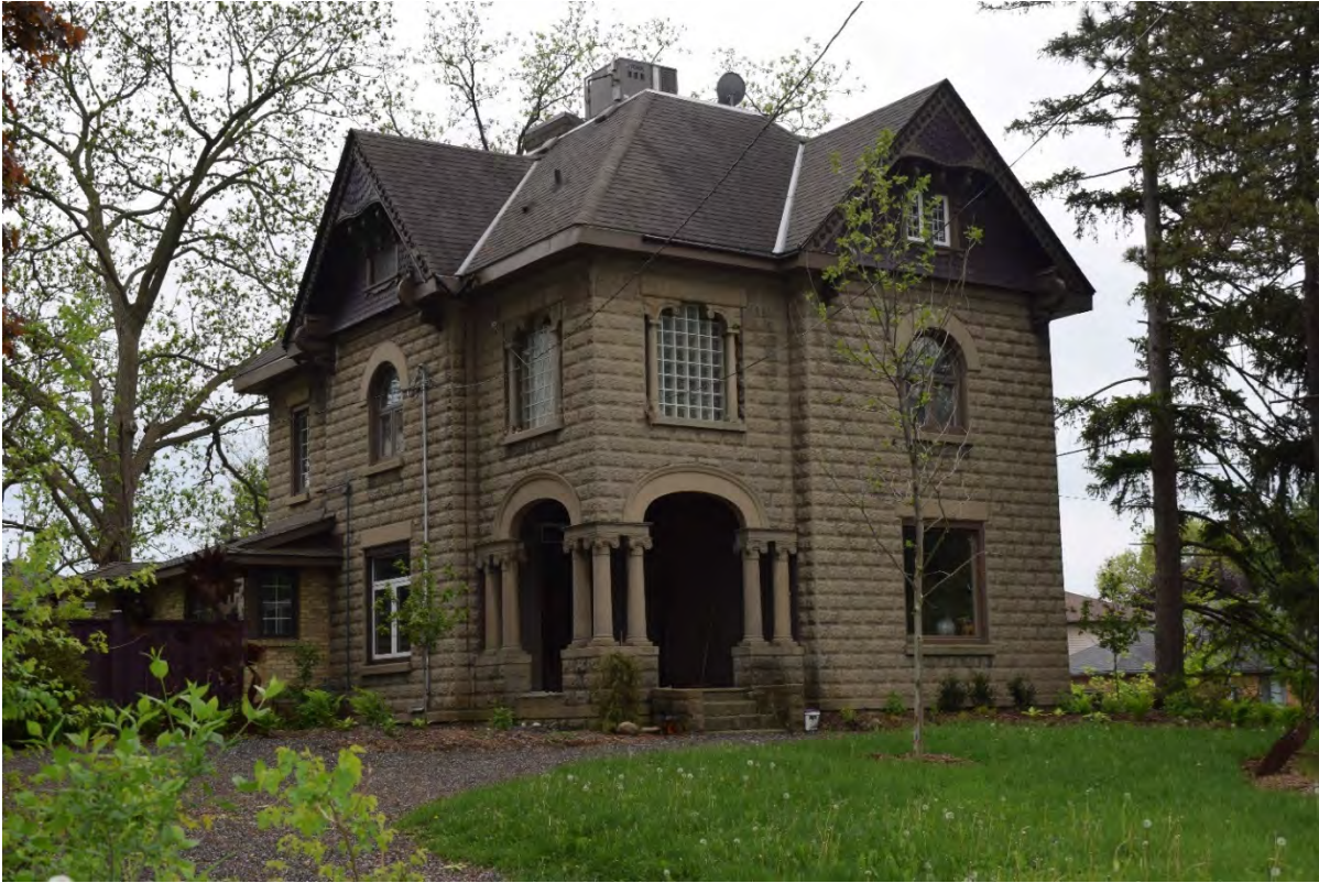
Plate 20: North (front) and east façades of 1158 Byron Baseline Road, looking south
