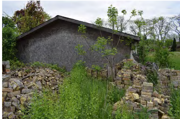
Plate 9: Buff brick piles, looking north
