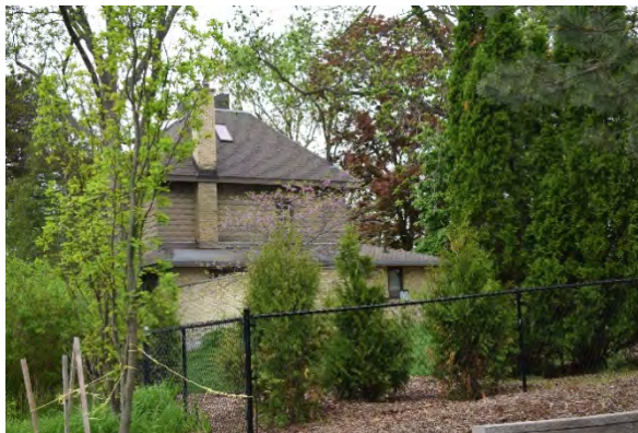
Plate 30: South façade of residence, looking north
