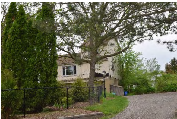
Plate 31: Outbuilding, looking east
