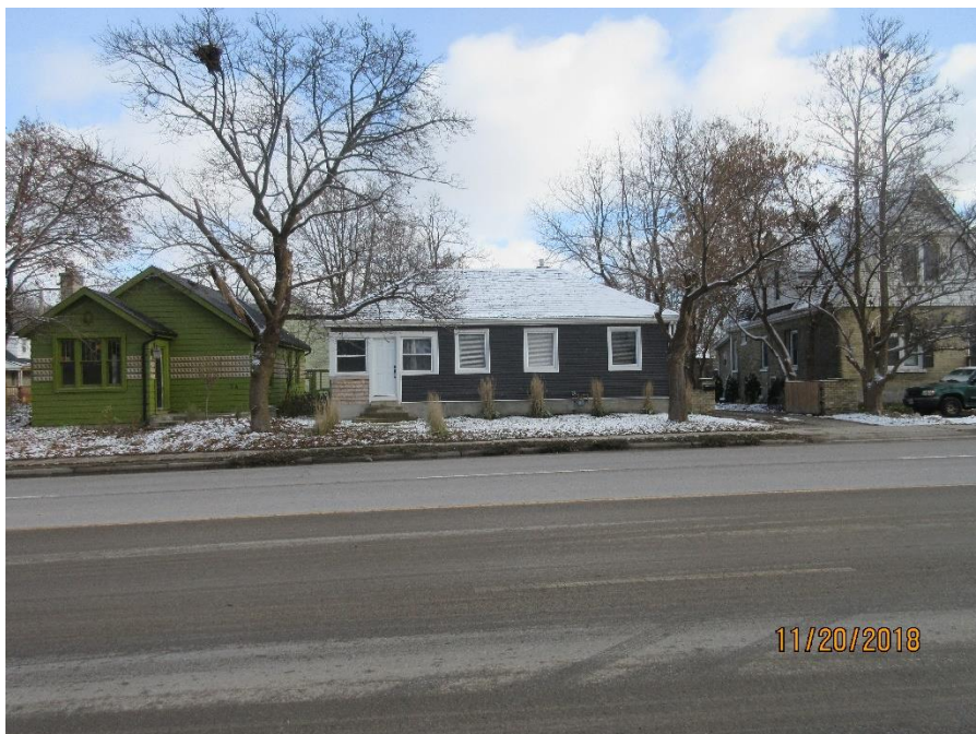
Image 3: Photograph of the property at 78 Wellington Road.
