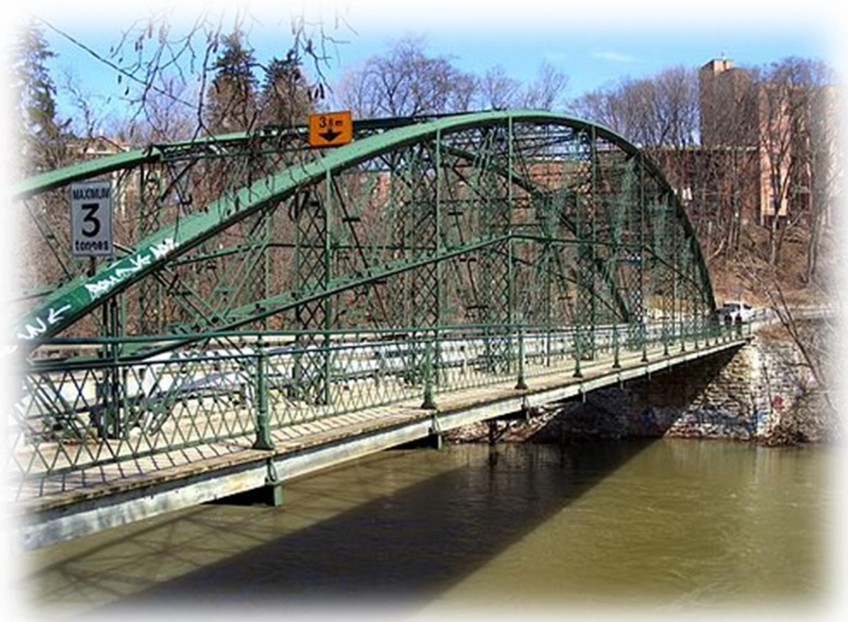
Blackfriars Bridge (photo credit: Canadian Consulting Engineer)
