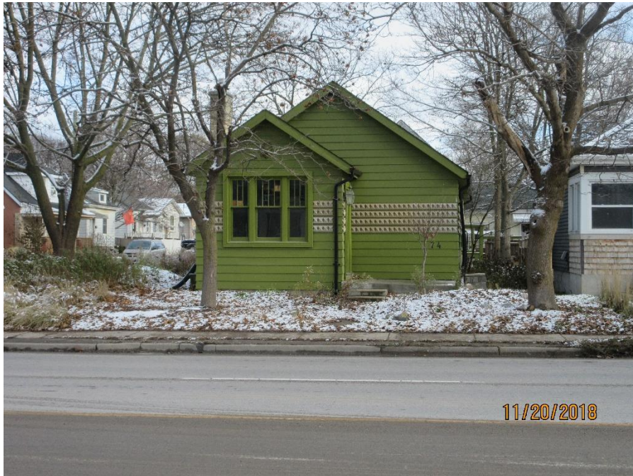
Image 2: Photograph of the property at 74 Wellington Road.
