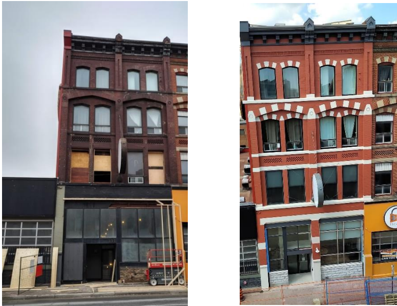
Figure 1: Joan's Place Phase 1 - Before & After of 333 Richmond St.
