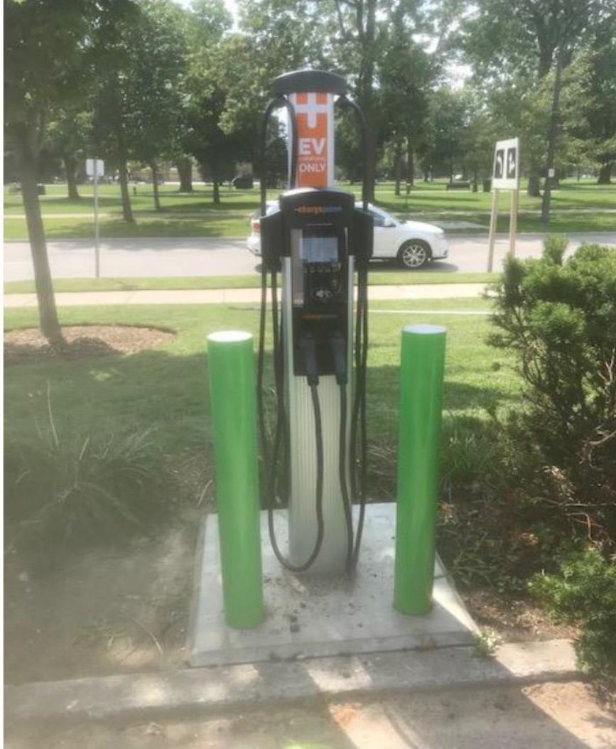
Sample of a Level 2, Dual EV Charger mounted on a precast concrete base. (located at London life)
