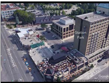
The Station Park development added density while incorporating the 1892/93 CPR railway station.
