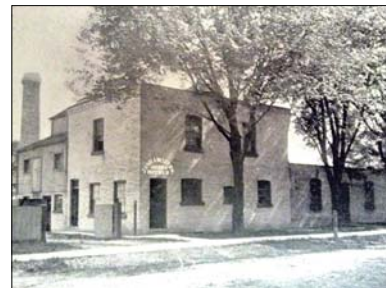
One re-use for the Kent Brewery building could be a pub, perhaps even a brew-pub.
