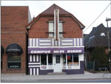
This first example shows that buildings don't have to be grand to be adaptively re-used. Humble structures can lend charm and variety to their surroundings. This building, which now houses the iconic Campus Hi-Fi, was built and used as a brick stable in the 1880s.
