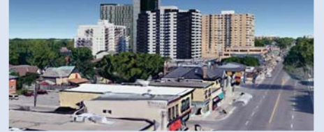
Looking North along Richmond Street
