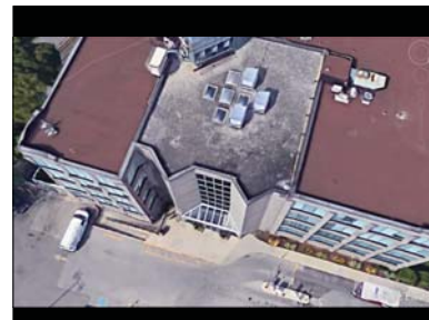
Another example is the filling-in of the courtyard of the 1909 Murray-Selby Shoe factory building at Piccadilly and Richmond Streets. The industrial feel of the factory was preserved while creating an airy modern atrium.
