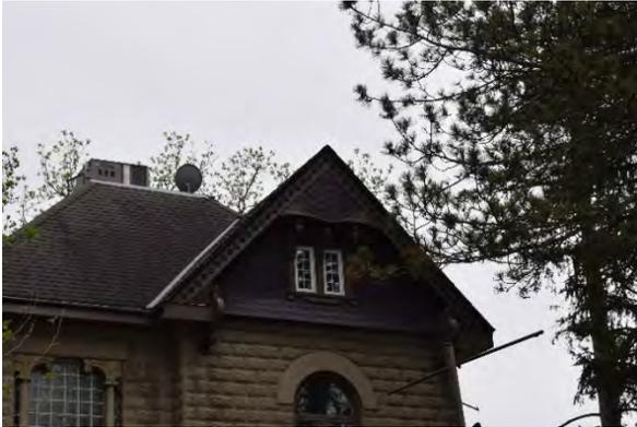
**Plate 23: Bargeboard, brackets, and fish scales, looking south**
