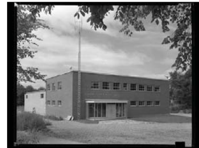
The Frank Gerry Warehouse at 50 Piccadilly Street (13 September 1954, London Free Press Collection of Photographic Negatives, Western Archives, Western University) now houses a nightclub.
