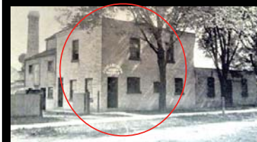
Main building of Kent Brewery post alterations and additions
