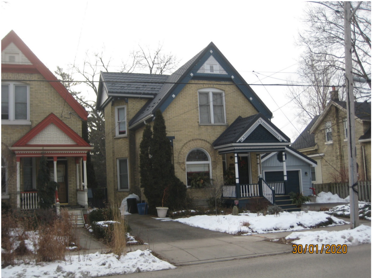
Image 17: Photograph showing unapproved roofing material alterations at 949 Lorne Avenue in January 2020
