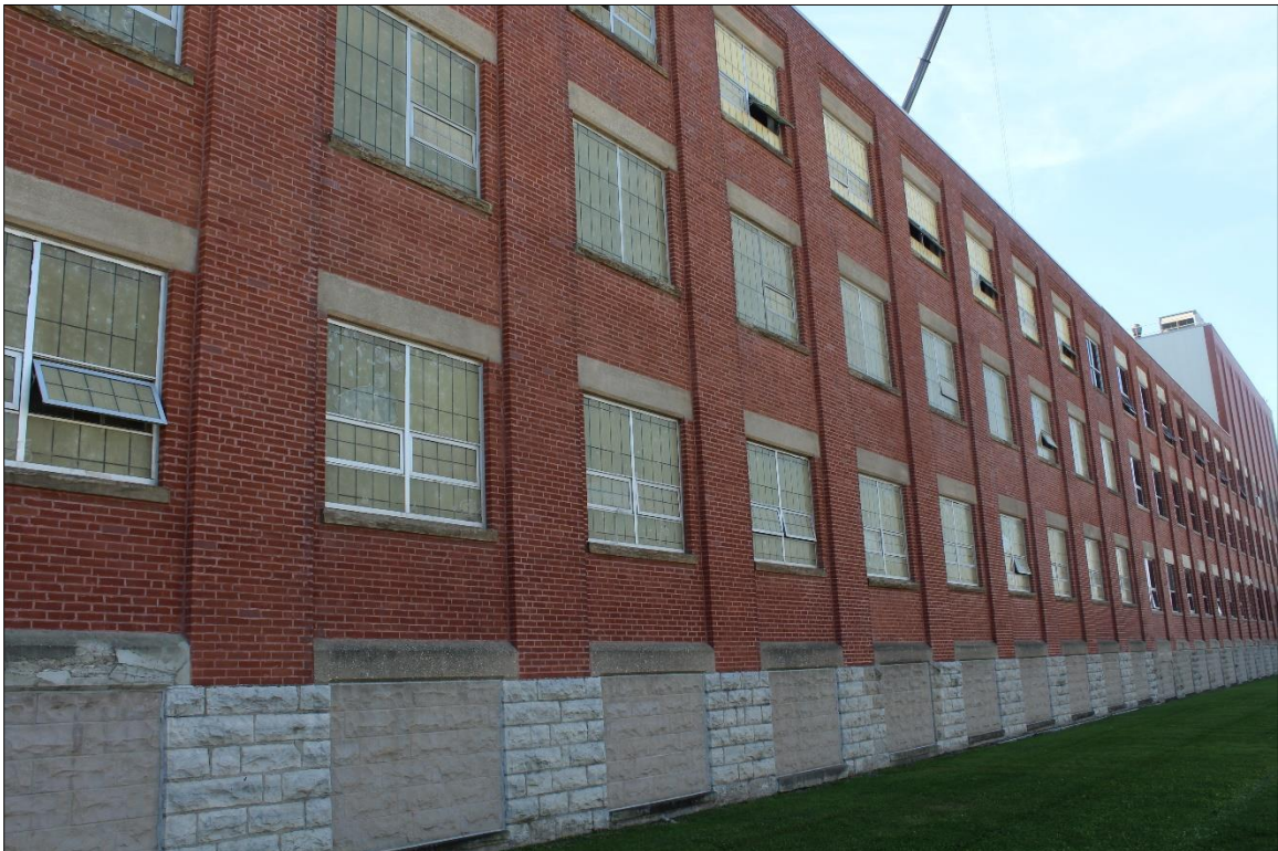
Image 5: Detail of window treatment (AECOM, 2019)
