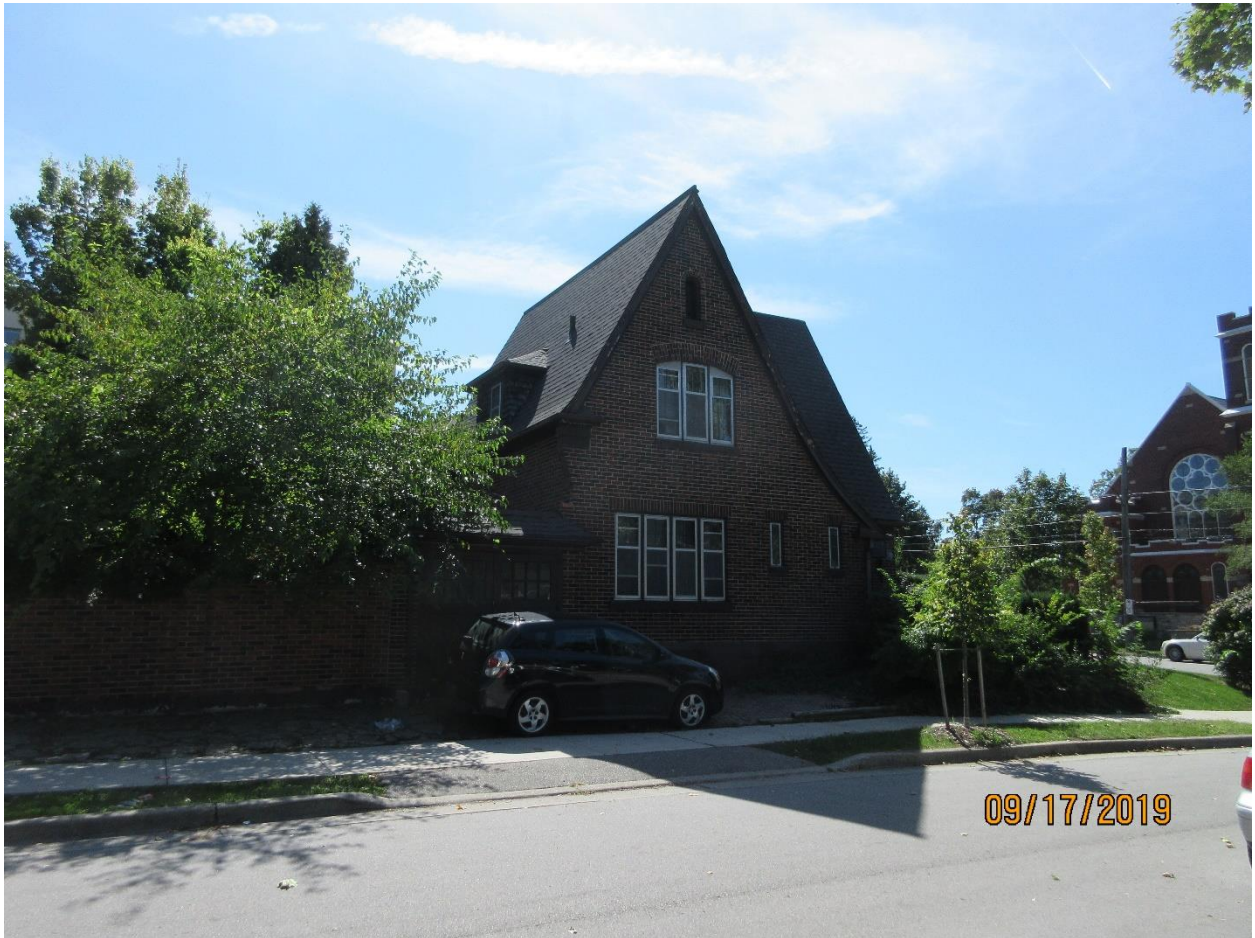
Image 9: Photograph showing the completed roofing replacement with asphalt shingles on the property at 1058 Richmond Street (east and north elevations) on September 17, 2019.
