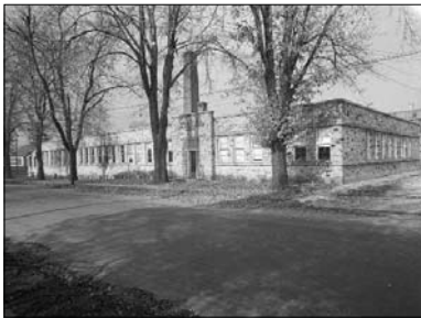
Other nearby industrial buildings have been adaptively reused. The Webster Air Equipment Ltd building at 140 Ann Street (London Free Press Collection of Photographic Negatives, 29 October 1948, Western Archives, Western University), is now home to Hutton House.
