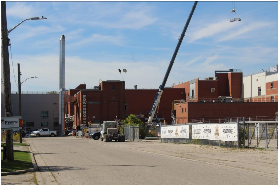
Image 11: Looking west along King Street towards powerhouse (AECOM, 2019)
