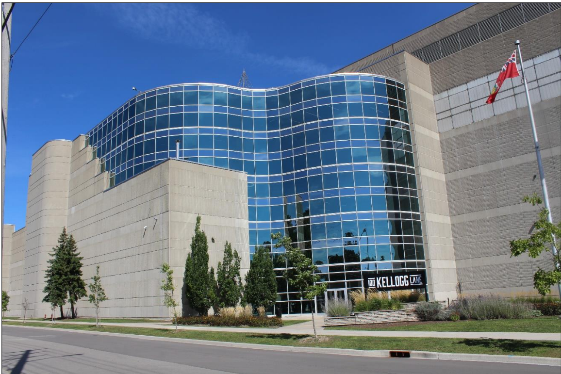
Image 9: 1982-86 addition, looking northeast from Kellogg Lane (AECOM, 2019)
