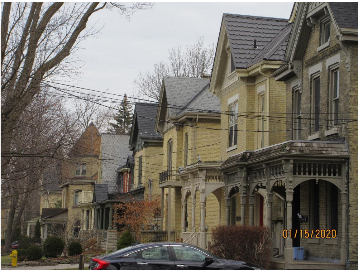
Image 17: Showing the streetscape of the south side of Wolfe Street, a variety of roofing materials can be seen. From right to left: asphalt shingles, metal roof, asphalt shingles, composite shingles, slate, and asphalt shingles. Some roofing materials are clearly more compatible with the heritage character of the West Woodfield Heritage Conservation District and the individual cultural heritage resources.
