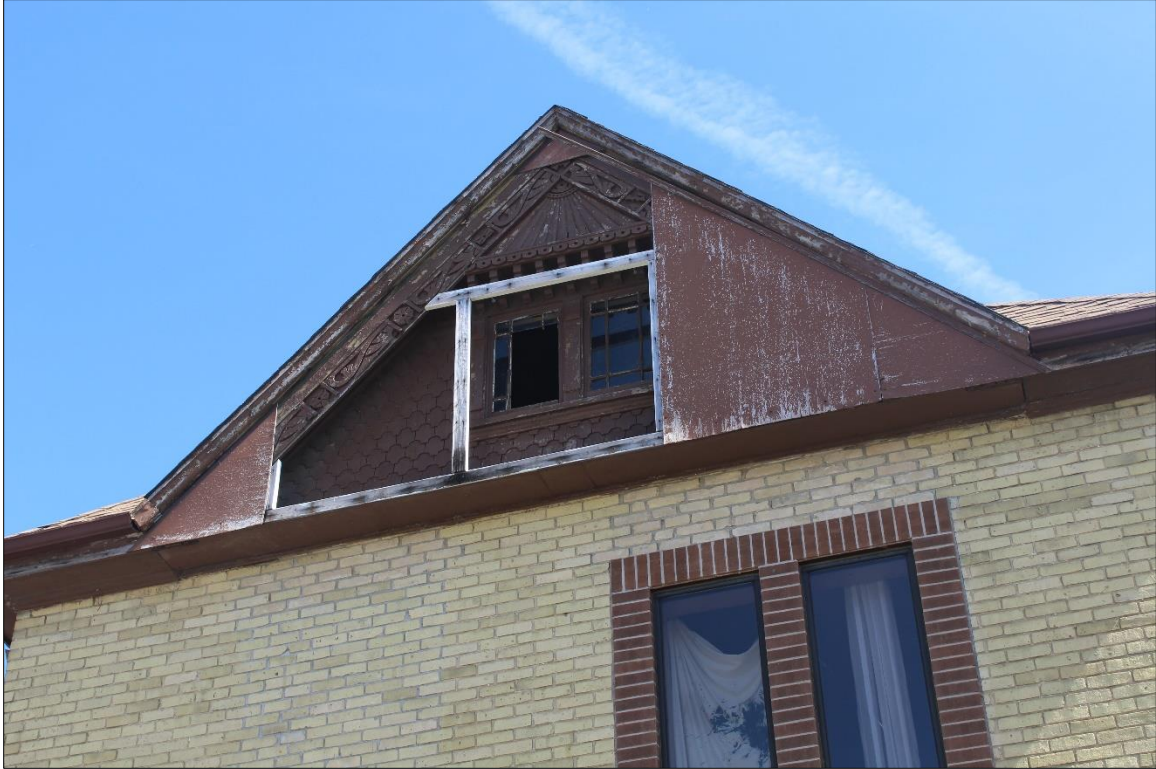
Image 4: Detail of bargeboard and shingle cladding in front gable (AECOM, 2019)
