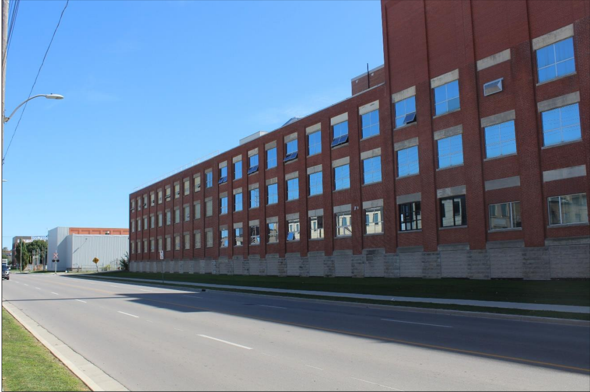
Image 4: Detail of window treatment (AECOM, 2019)
