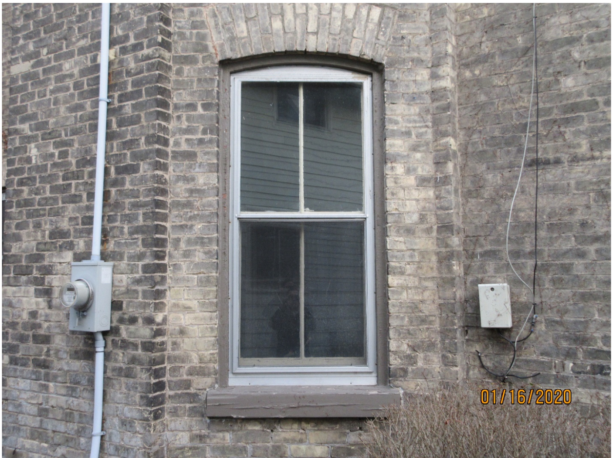
Image 6: Detail photograph of the exterior of the window on the easterly bay on the property at 40 Askin Street.
