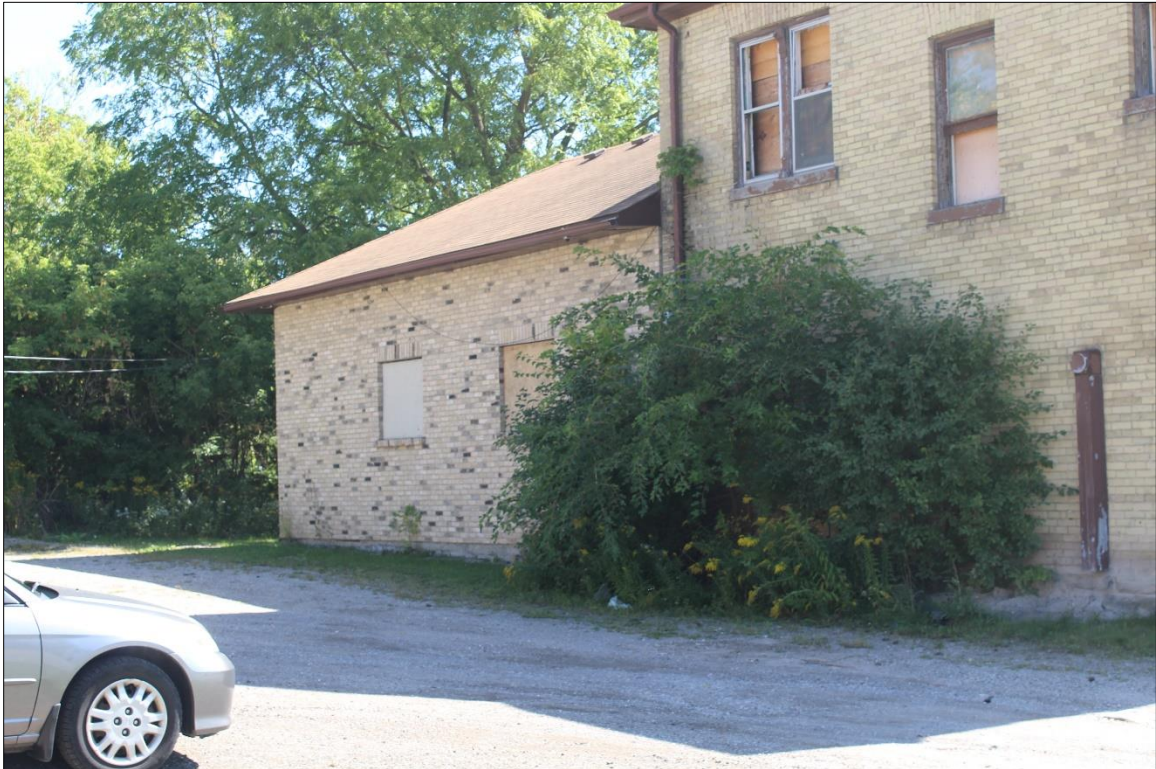
Image 3: Single-storey extension at rear of building (AECOM, 2019)
