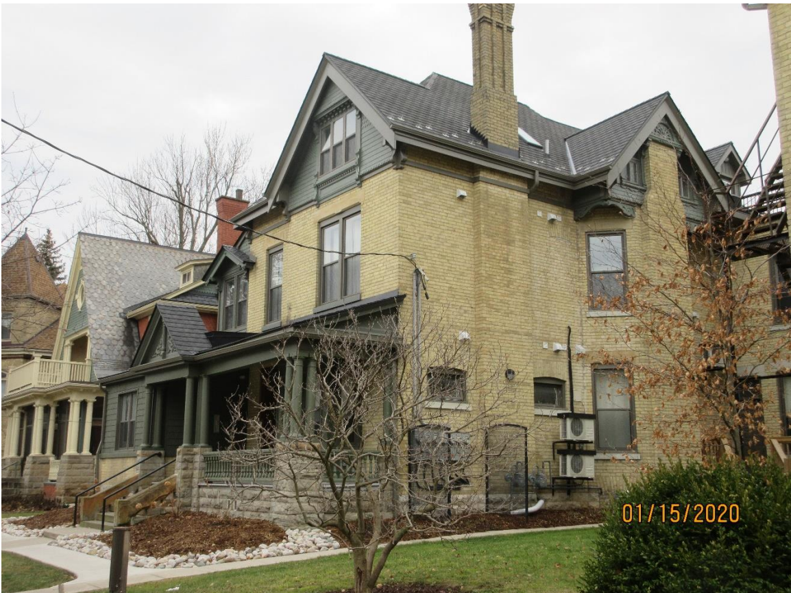
Image 15: Photograph of the property at 309-311 Wolfe Street following roofing replacement with a rubber composite product on January 15, 2020.
