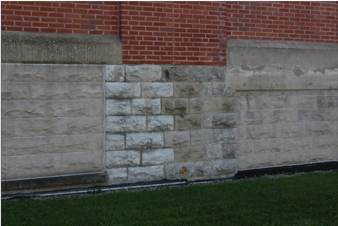
Image 6: Detail of foundation and joint between 1914 and 1933 structures (AECOM, 2019)
