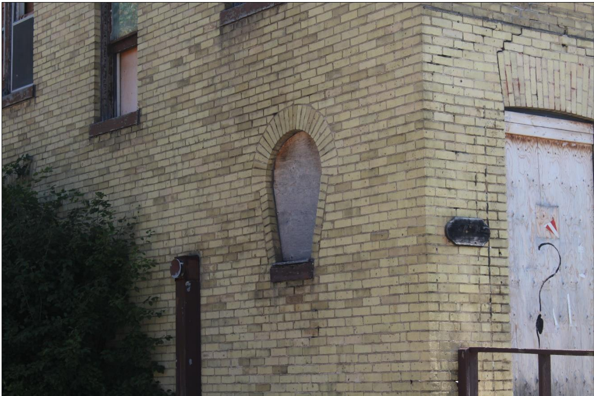
Image 5: Detail of Keyhole window on north façade (AECOM, 2019)
