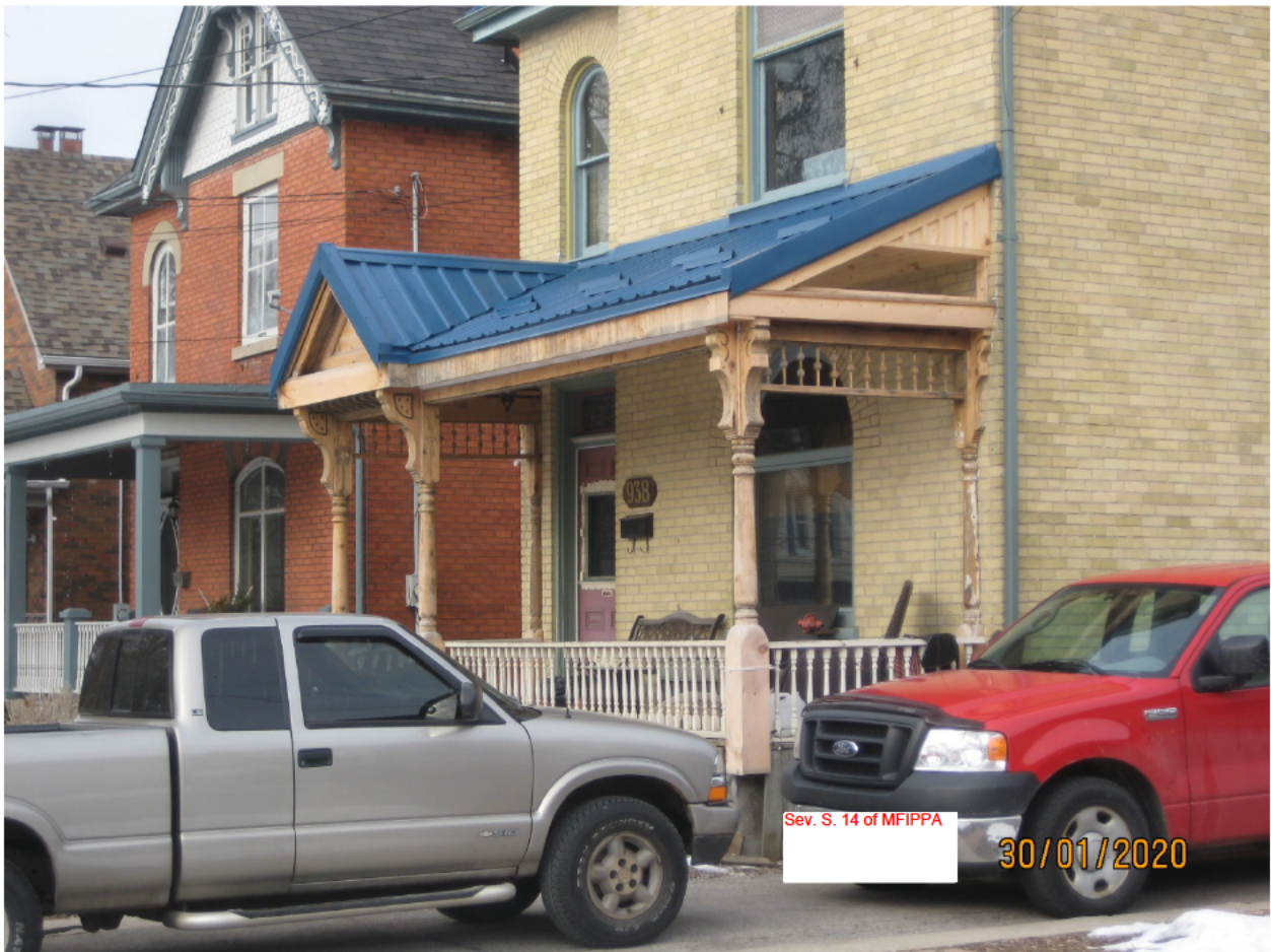
Image 12: Photograph showing porch alterations completed to date, in January 2020
