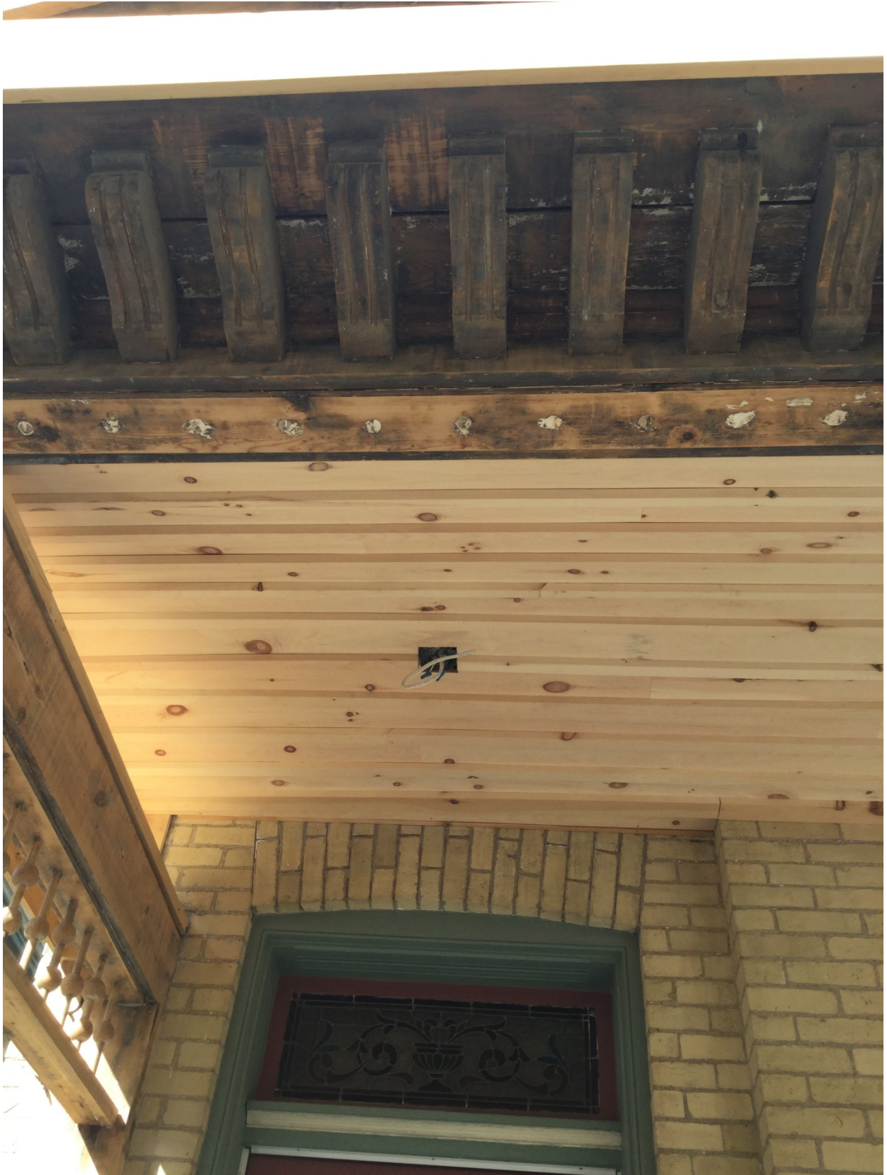
Image 8: Photograph submitted as a part of the Heritage Alteration Permit application for 938 Lorne Avenue showing the alterations to the verandah ceiling and evidence of removed spandrels exposed during alterations to the porch
