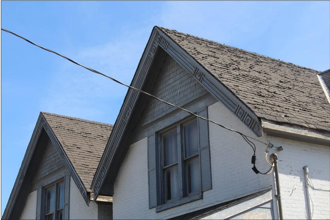
Image 5: Detail of shingles and decorative bargeboards (AECOM, 2019)
