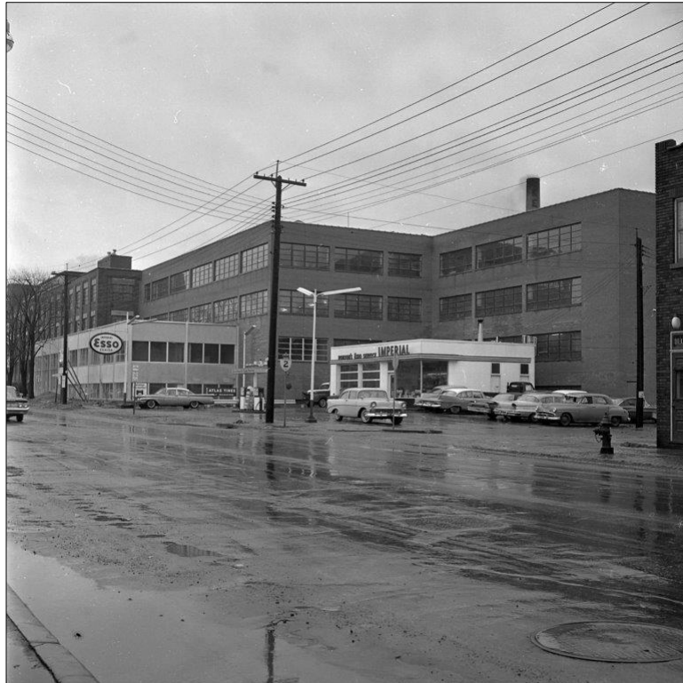
Image 3: Looking east along Dundas at Kellogg Lane (then Eva Street), showing new plant addition, 1961 (London Public Library - London Room)
