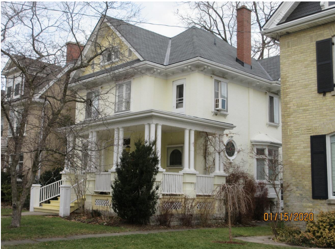
Image 13: Photograph of the property at 836 Wellington Street, following the replacement of the slate roof with an asphalt shingle ("slateline" faux slate).
