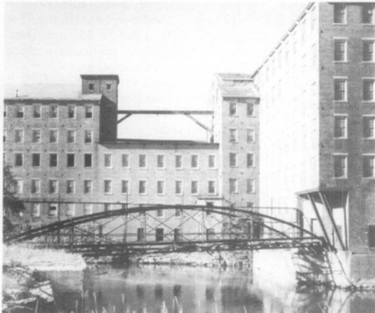
Figure 1. Windows are frequently important visual focal points, especially on simple facades such as this mill building. Replacement of the multi-pane windows here with larger panes could dramatically change the appearance of the building. The areas of missing windows convey the impression of such a change. Photo: John T. Lowe
