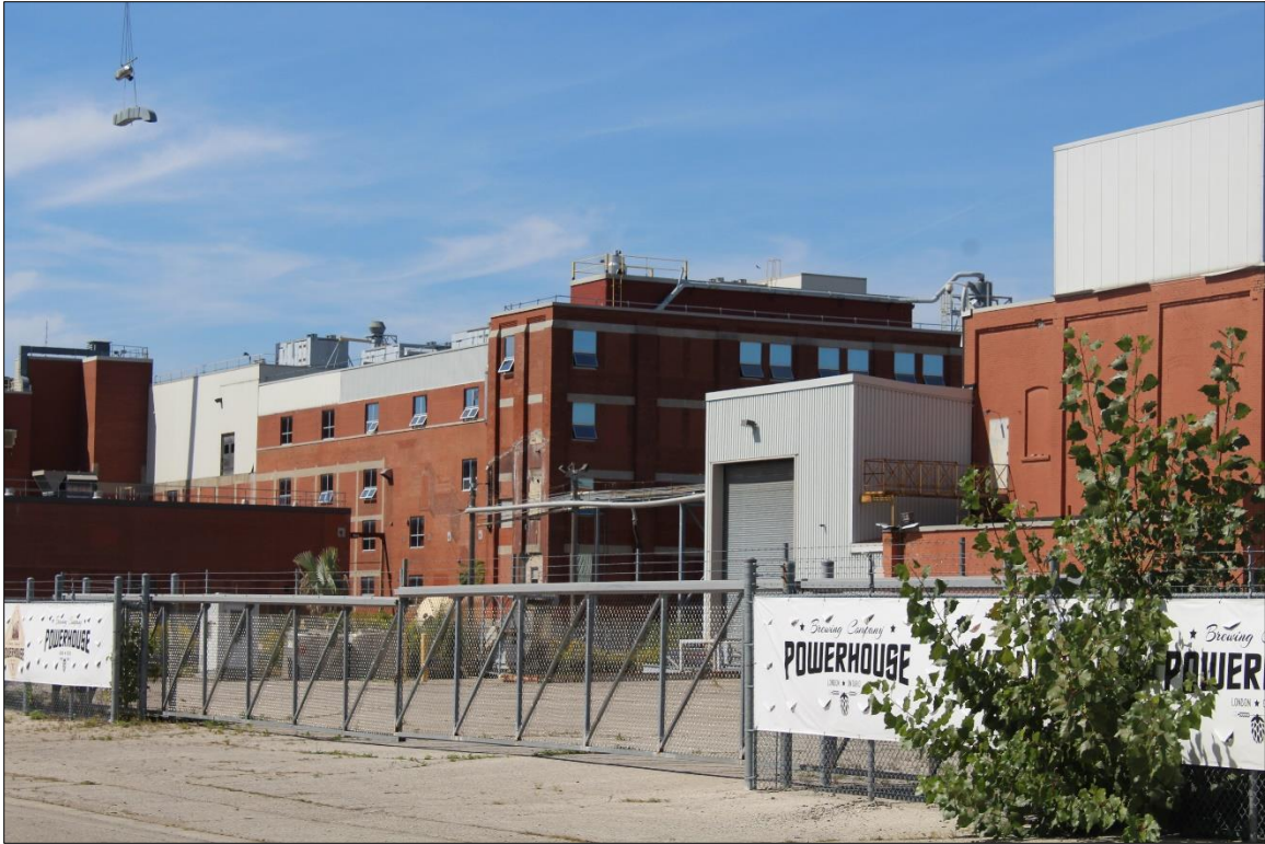
Image 10: Rear of property looking northwest from King Street (AECOM, 2019)
