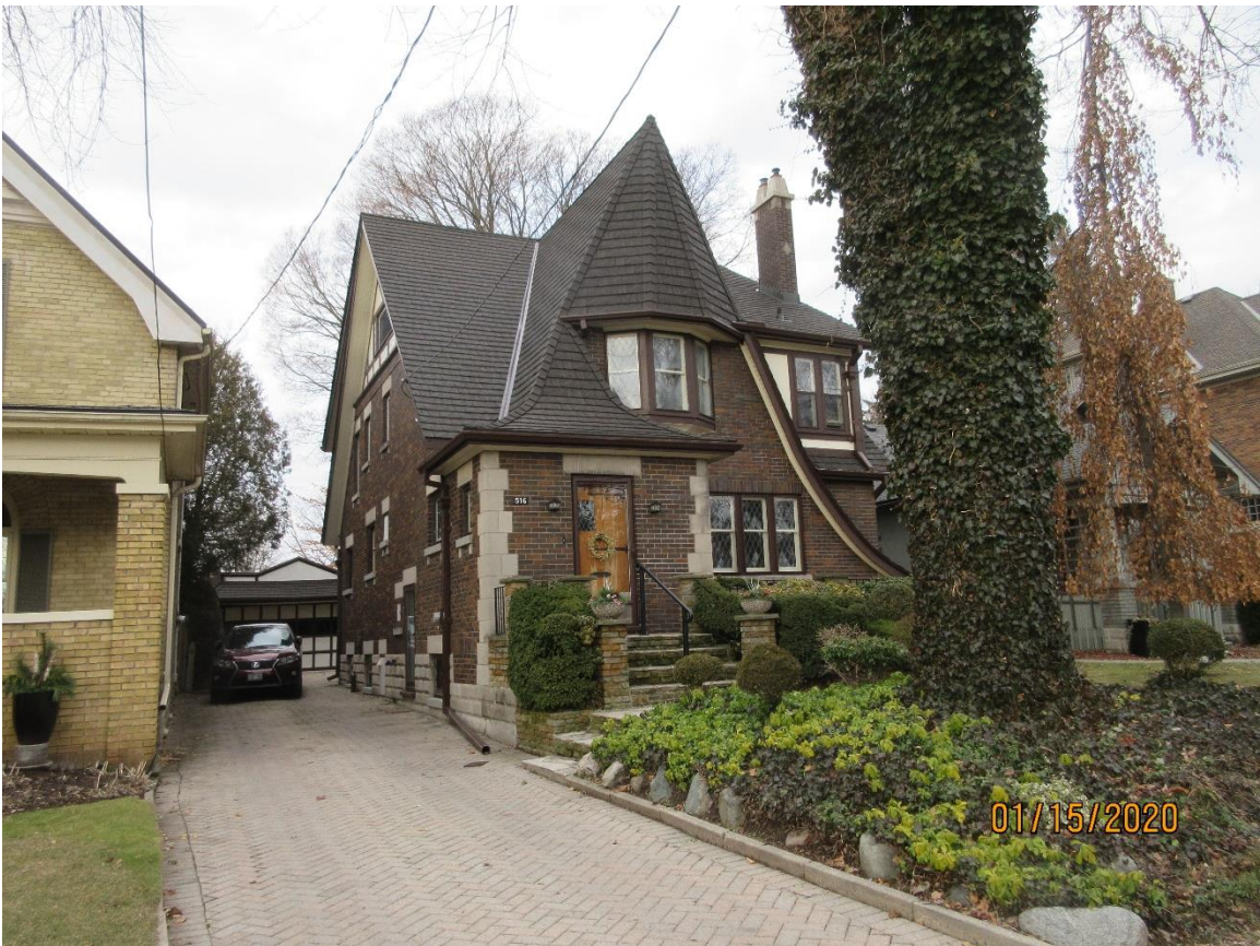
Image 19: Photograph of the property at 516 Grosvenor Street on January 15, 2020, following replacement of the wood shingle roofing with a composite rubber roofing product.
