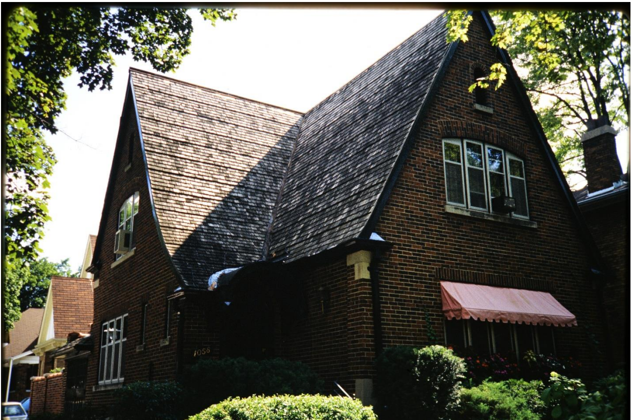
Image 2: Detail photograph of the property at 1058 Richmond Street, emphasizing the wood shingle roof (c.1990).
