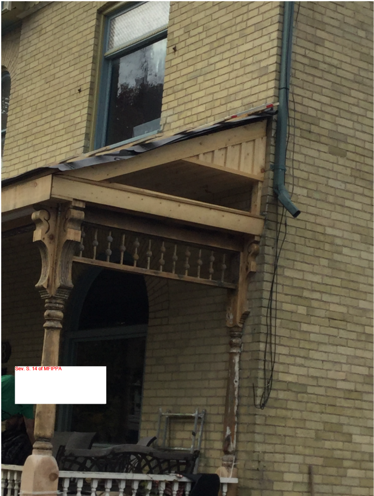
Image 7: Photograph submitted as a part of the Heritage Alteration Permit application for 938 Lorne Avenue showing detail of the porch design and existing spandrel details
