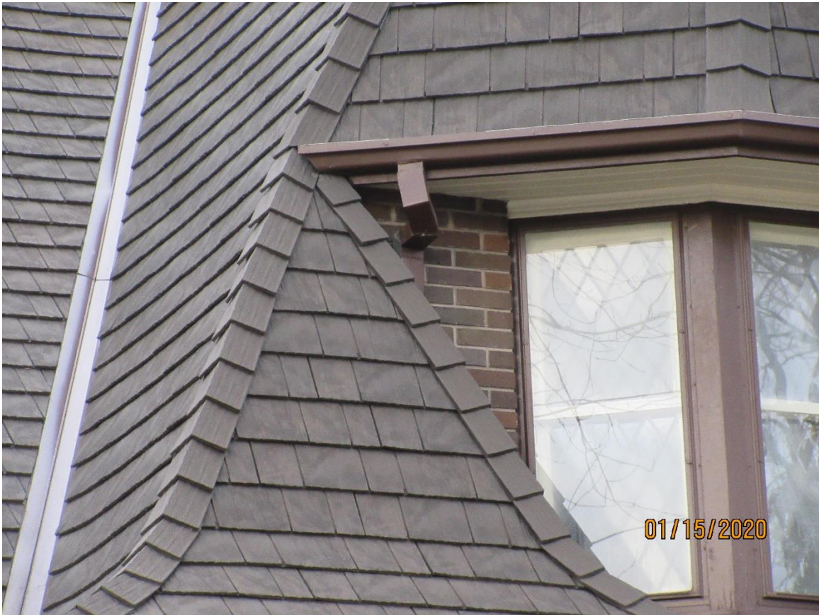
Image 20: Detail photograph of the composite roof product used on the property at 516 Grosvenor Street to replace the wood shingle roof.
