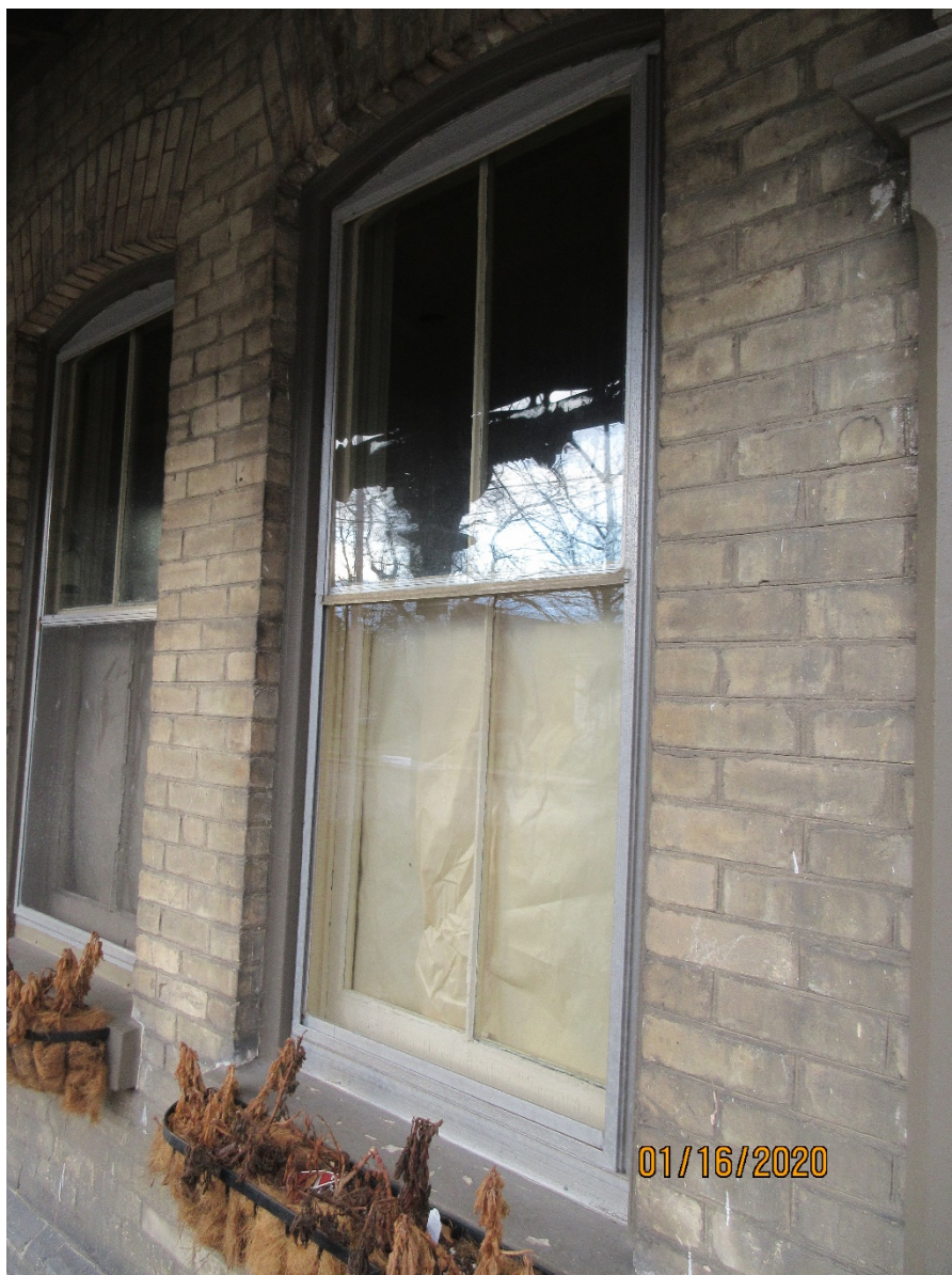
Image 4: Detail photograph of the windows under the porch on the property at 42 Askin Street. Note that the window openings are topped by a segmented arch brick voussoir; the wood windows feature a segmented arch top sash which is obscured by the rectangular aluminum storm window applied over top.
