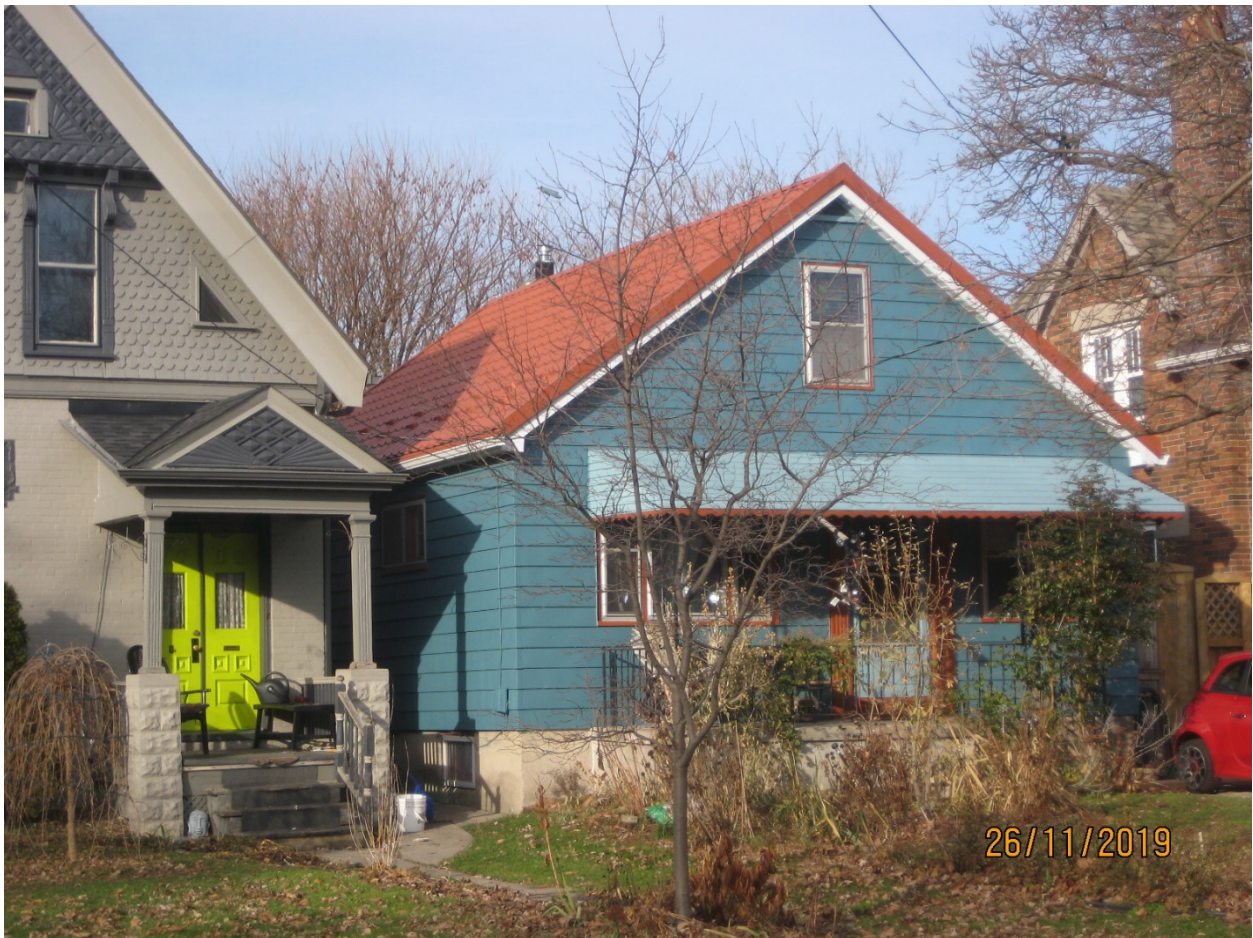
Image 16: Photograph showing unapproved roofing material alteration at 932 Lorne Avenue in November 2019
