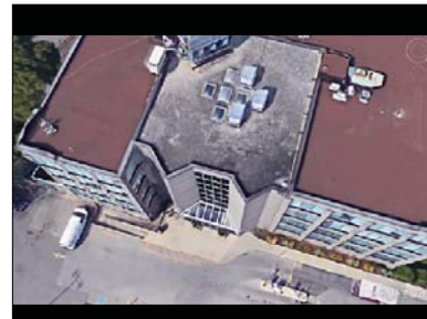
By filling in the courtyard of the 1909 Murray-Selby Shoe factory building at Piccadilly and Richmond Streets, the industrial feel was preserved while creating an airy modern atrium.
