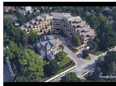
The Sir Adam Beck house was rebuilt with modern materials after an attempt was made to rebuild it with the original materials. Lessons were learned, but the intent was there to incorporate the historic fabric and simultaneously intensify.
