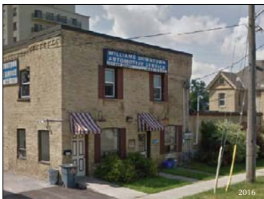
Apart from a new door in the centre, the main Kent Brewery building (left) and its washhouse (right) still look much as they did in their heyday, when the c. 1905 photograph was taken. The building is currently the Williams Downtown Automotive Service at 197 Ann Street. The building today is the "largest surviving brewery artifact from Victorian London Middlesex". (Phillips, 155). The Brewery was already considered old in the 19th Century. In 1889, Goodspeed's History of the County of Middlesex said of the Kent Brewery: "The premises form one of the oldest landmarks in the city, and are located on Ann Street." (Goodspeed, p. 373)
