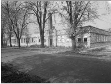
Other nearby industrial buildings have been adaptively reused. The Webster Air Equipment Ltd building at 140 Ann Street (London Free Press Collection of Photographic Negatives, 29 October 1948, Western Archives, Western University), is now home to Hutton House.
