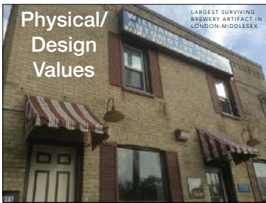
This section summarizes research conducted towards evaluating physical design values for a potential statement of designation for 197 Ann Street.
