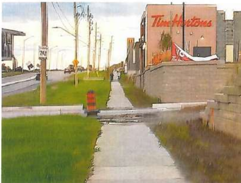
Image 5 – Driveways limiting direct access to Oxford Street to drive through restaurants, and median separating west bound traffic from entering the restaurants.
