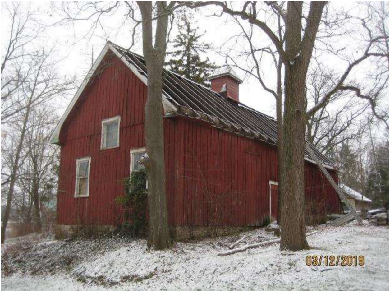
Image 23: Photograph of the west side of the accessory building, showing the removed roof sheathing, December 3, 2019.
