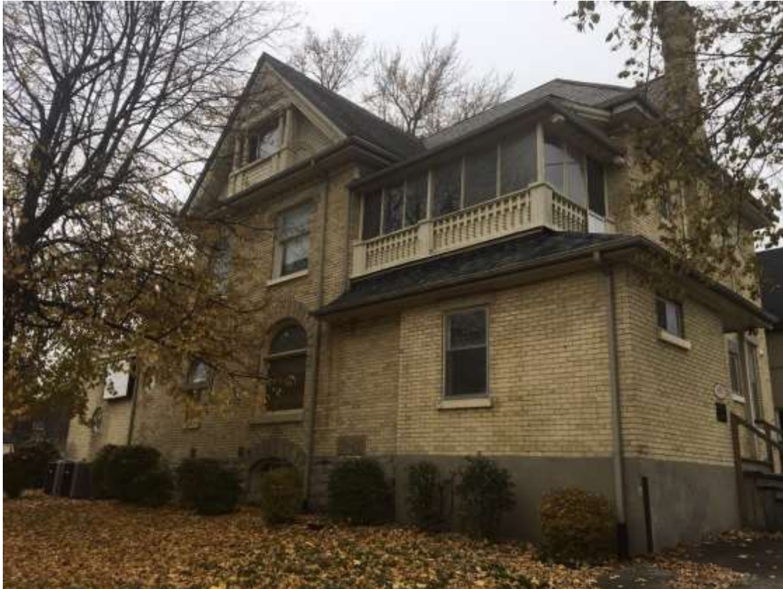
Figure 1: Subject site (view off of Central Avenue).
