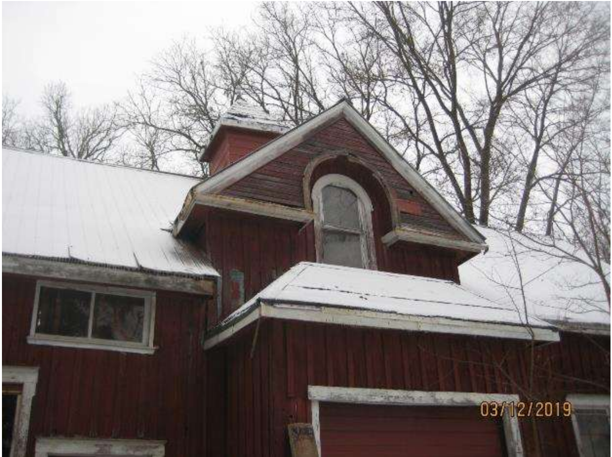
Image 25: Detail of the central projecting gable peak, round-headed window, and hipped roof covering the bay entrance to the accessory building. The ventilator can be seen rising above the centre of the peak, December 3, 2019.
