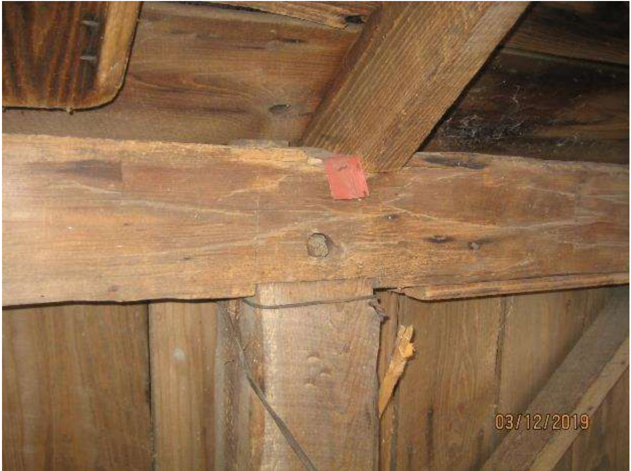
Image 29: Interior detail showing traditional mortise and tenon timber frame connections used throughout the accessory building, December 3, 2019.
