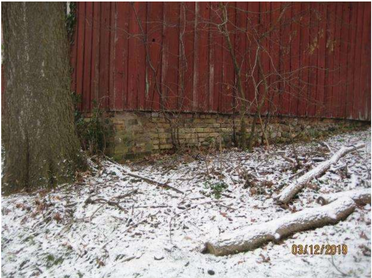
Image 24: Photograph of the foundation on the west side of the accessory building showing a mix of buff brick and field stone materials, December 3, 2019.
