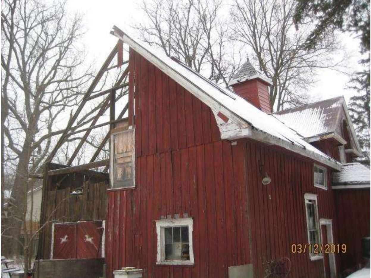
Image 22: Photograph of the south side of the accessory building. Note the portions of the exterior cladding and roof had been removed by the property owner the in the fall of 2019, December 3, 2019.
