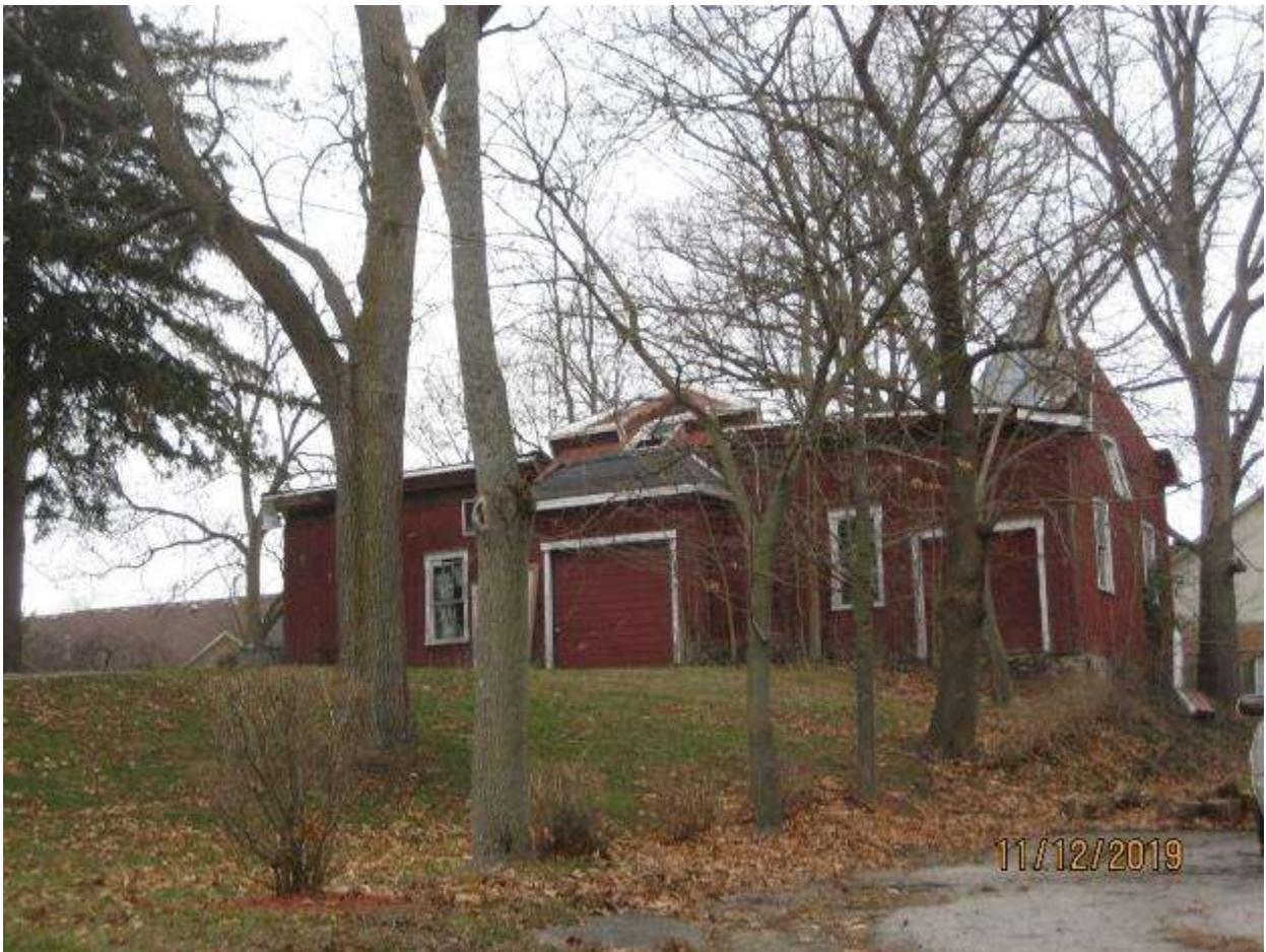
*Image 32: Photograph showing the east side of the accessory building as viewed from Halls Mill Road, showing the collapse of the roof framing, December 11, 2019.*
