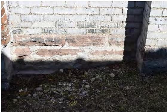
**Plate 13: Rusticated concrete block foundation, looking east**
