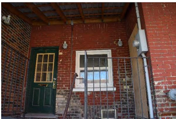
**Plate 14: Replacement window and door openings, looking west**
