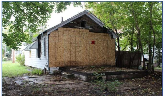
Clockwise from top Left 24. North elevation of 88 Blackfriars Street. 25. Interior view of the gutted interior of 88 Blackfriars, with the partially demolished rear exterior walls and roof. 26. View of the south elevation with temporary plywood sheeting as per City of London unsafe building order. 27. View of crawl space and mud sill floor framing and opening from collapsed foundation.
