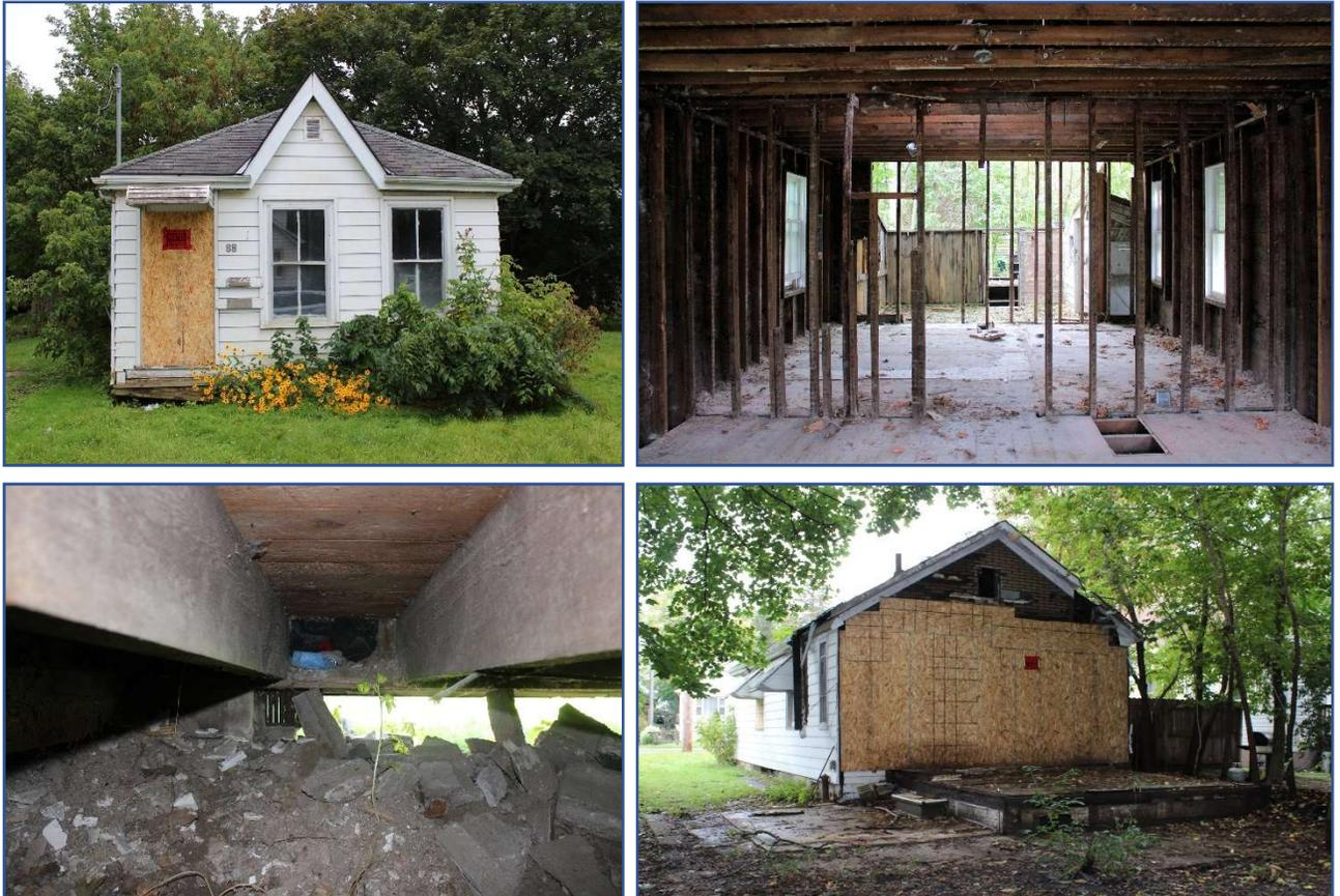
Clockwise from top Left 24. North elevation of 88 Blackfriars Street. 25. Interior view of the gutted interior of 88 Blackfriars, with the partially demolished rear exterior walls and roof. 26. View of the south elevation with temporary plywood sheathing as per City of London unsafe building order. 27. View of crawl space and mud sill floor framing and opening from collapsed foundation.
