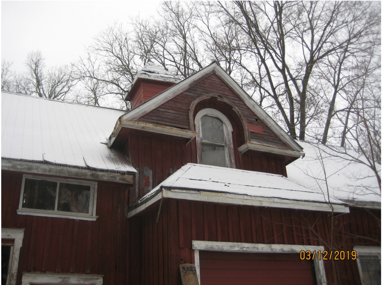
Image 25: Detail of the central projecting gable peak, round-headed window, and hipped roof covering the bay entrance to the accessory building. The ventilator can be seen rising above the centre of the peak, December 3, 2019.
