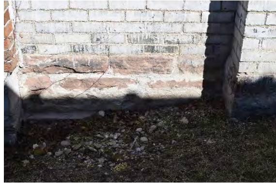
Plate 13: Rusticated concrete block foundation, looking east
