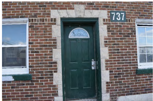
Plate 17: Stone door surround, looking south
