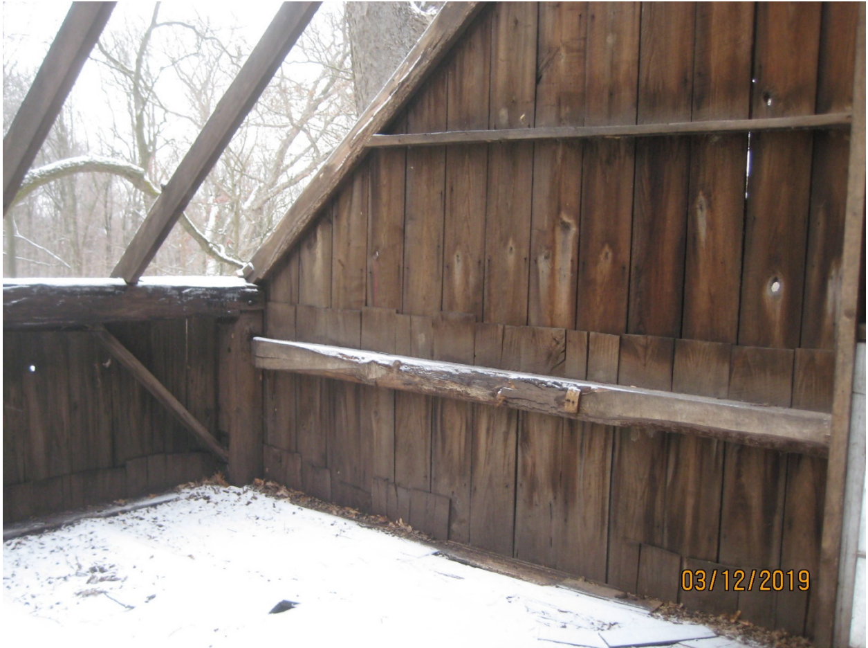
Image 27: Interior detail of the mortise and tenon timber frame construction of the accessory building, December 3, 2019.
