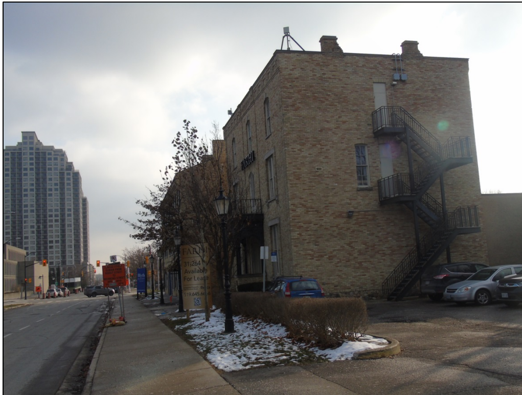
Image 9: View showing rear of the three heritage buildings from the surface parking lot accessed from Queens Avenue
