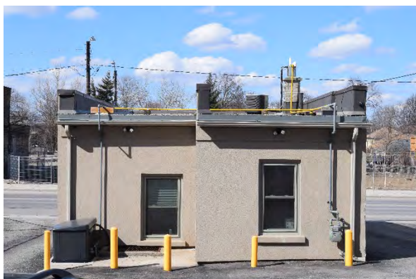
Plate 32: Rear (south) façade of 729 Dundas Street, looking north
