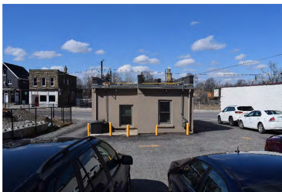
Plate 33: Asphalt parking lot, looking north
