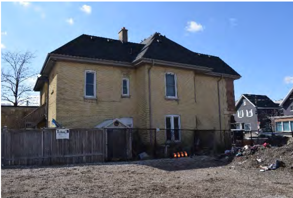
Plate 35: East façade, looking west
