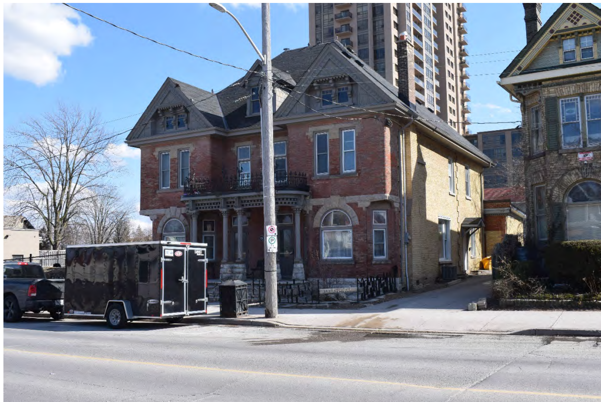
Plate 34: 719-721 Dundas Street, front façade and west façade, looking south
