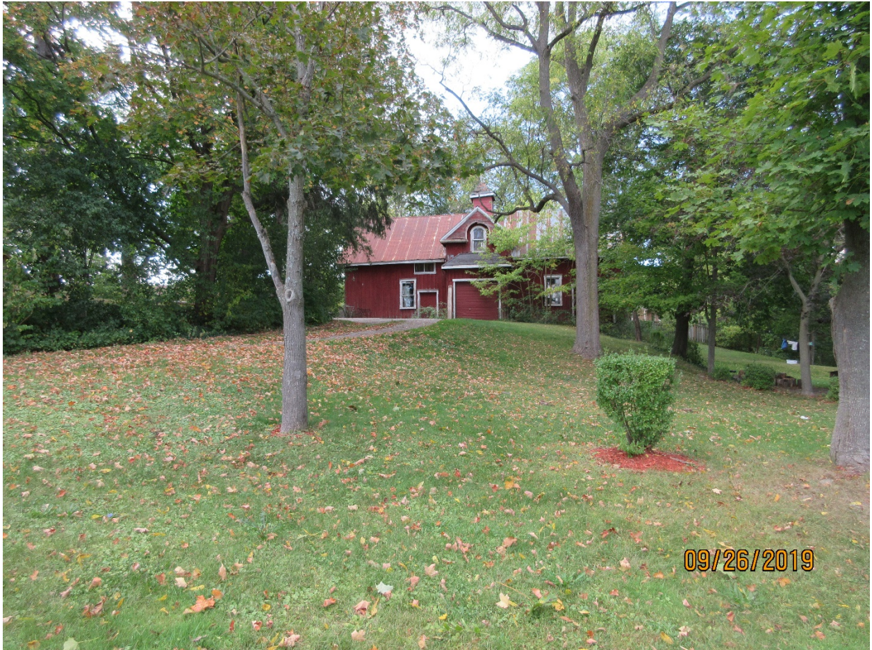
Image 11: Photograph of the accessory building as viewed from Halls Mill Road, September 2019.
