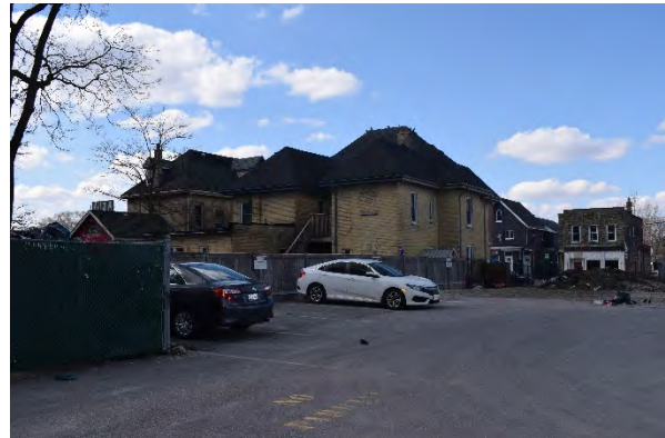
Plate 36: Rear (south) façade, looking north
