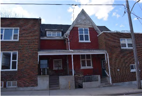
Plate 12: Original portion of 737 Dundas Street, looking west
