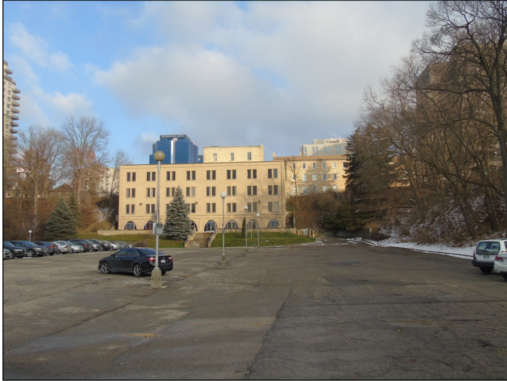
Image 7: View showing modern commercial structure constructed to the rear of 451 Ridout Street North, built into the embankment
