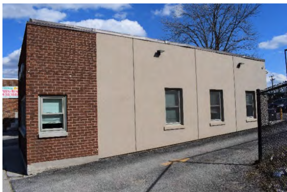
Plate 30: West façade of 729 Dundas Street, looking east
