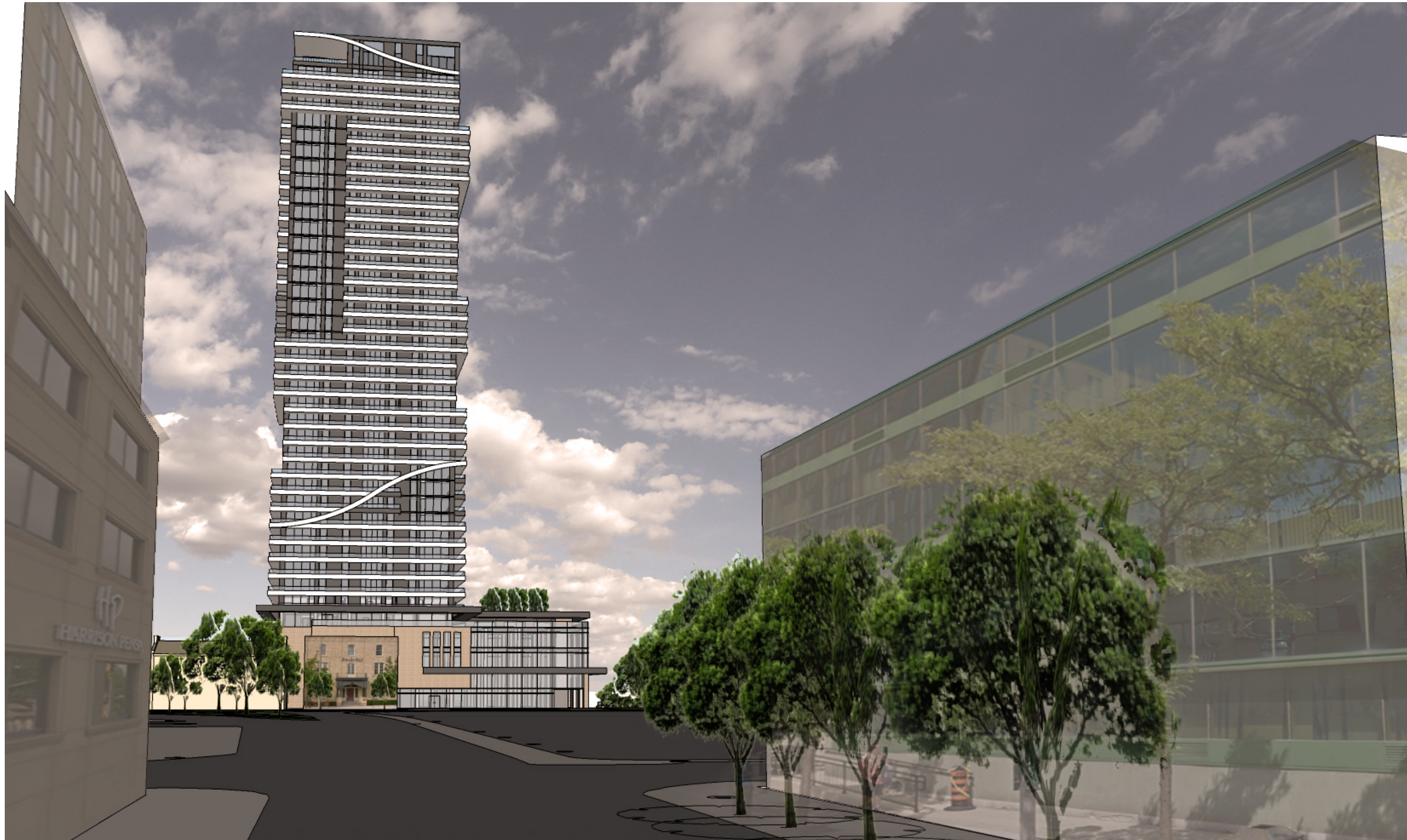
QUEENS AVENUE VIEW (EAST FACADE)
