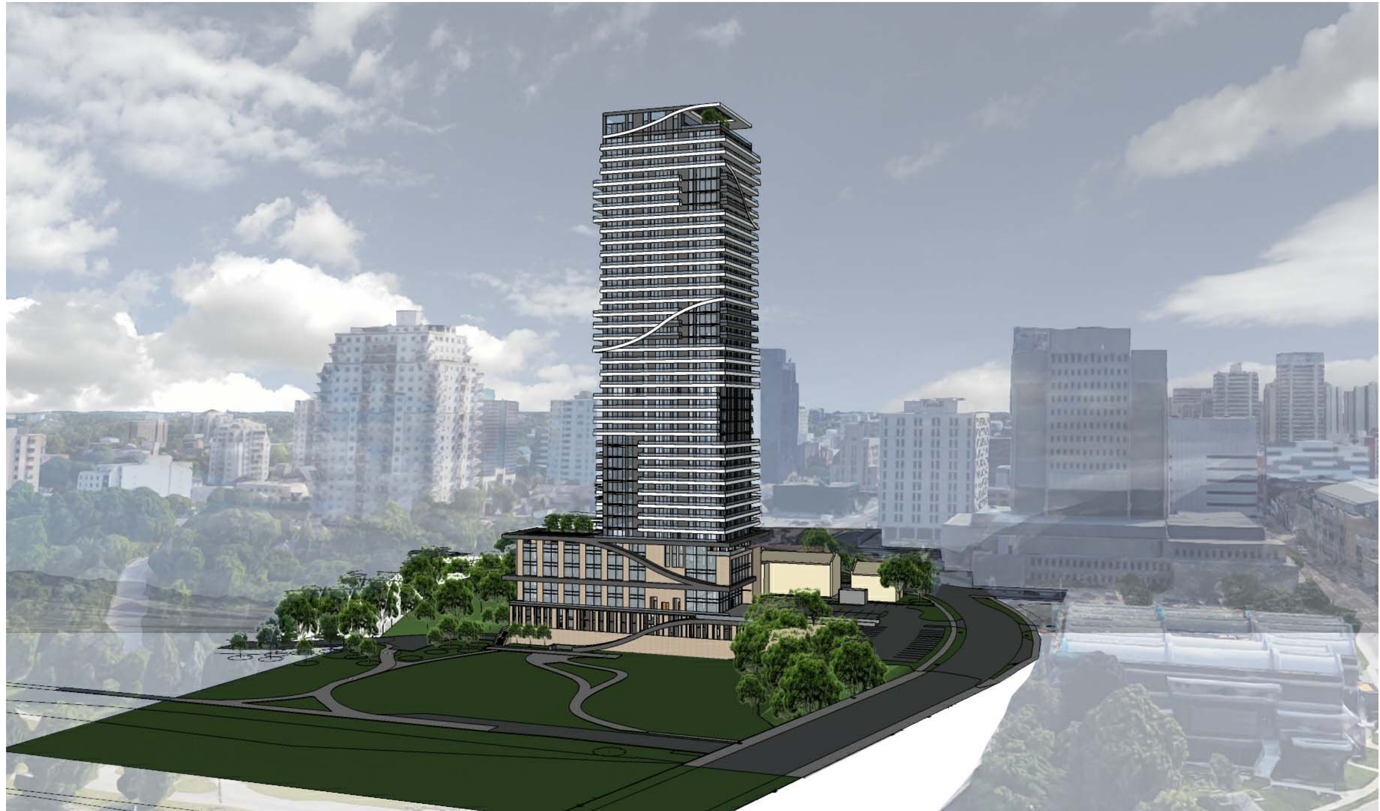
WEST FACADE ARIAL VIEW (PARK)
