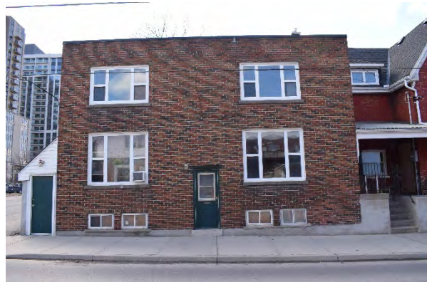
Plate 19: East façade of rear addition, looking west
