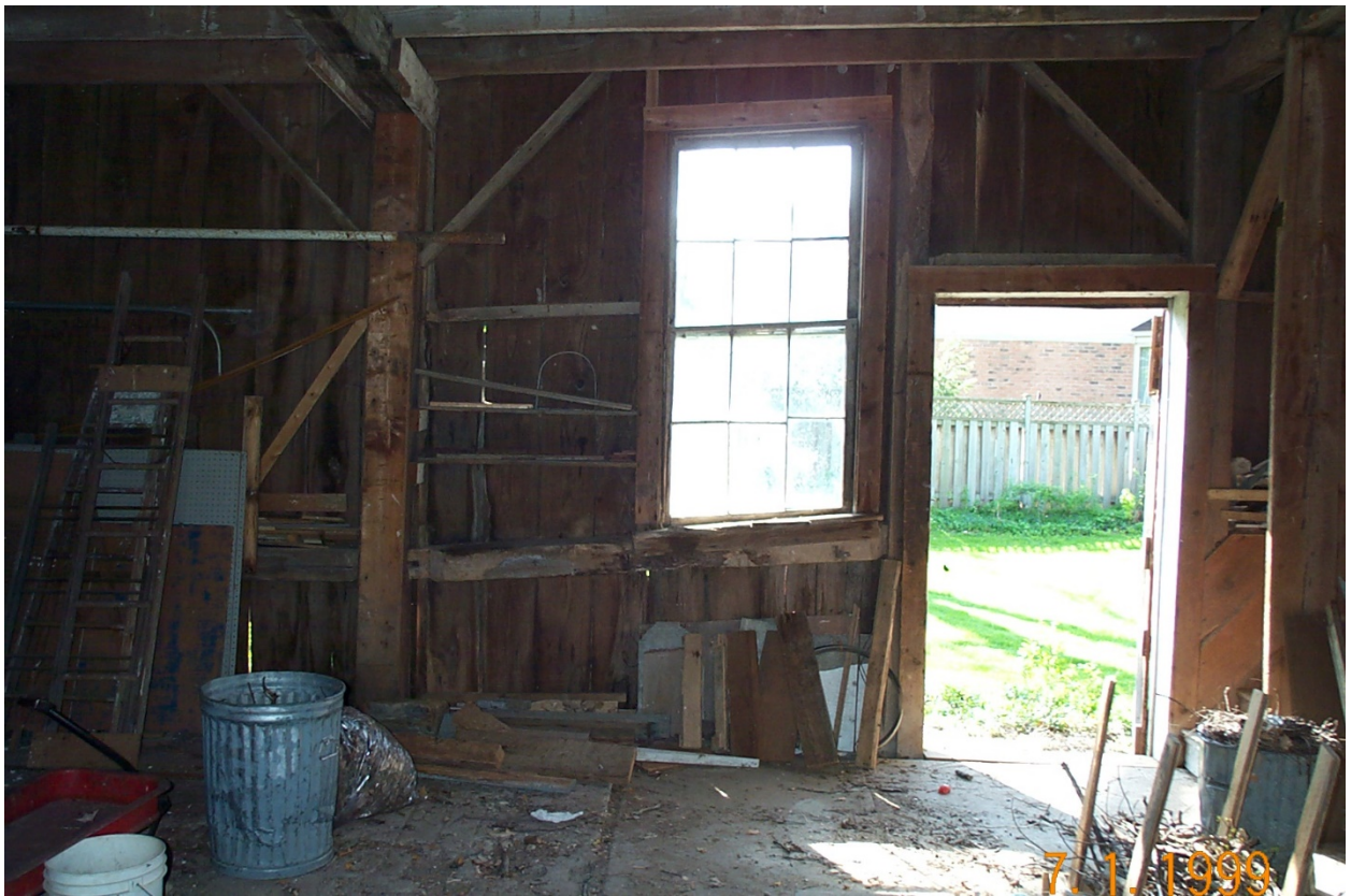
Image 8: Interior photograph of the accessory building, showing the interior of the west wall of the building, 1999.
