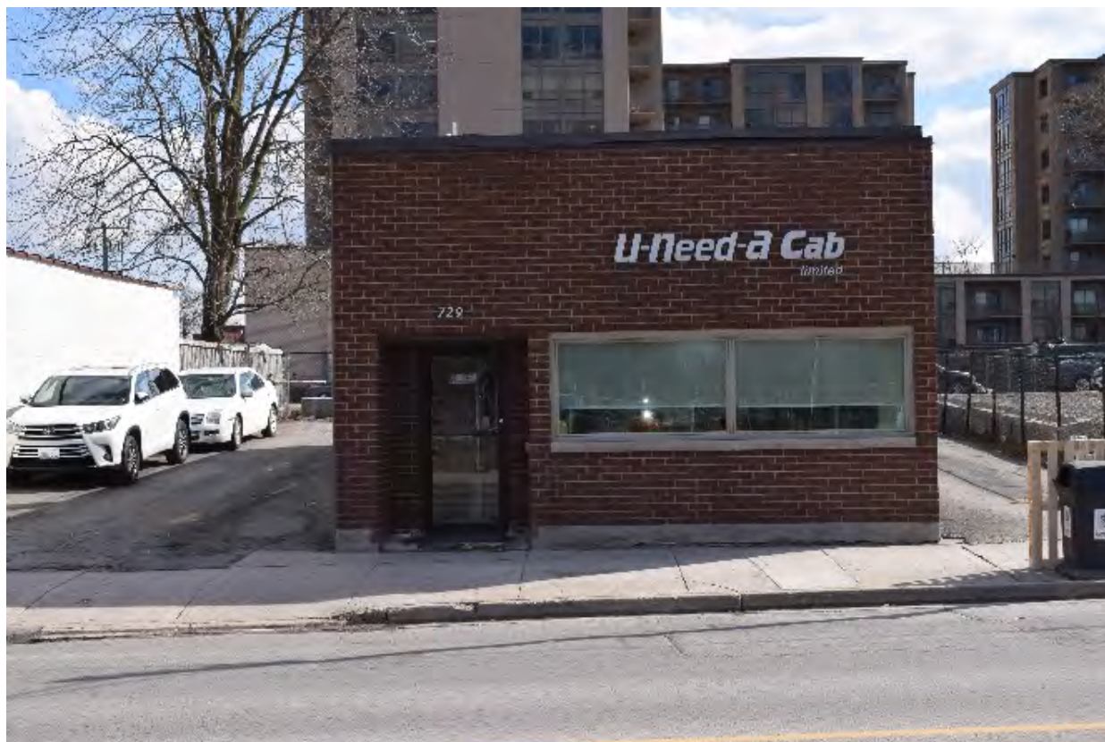
Plate 29: Front (north) façade of 729 Dundas Street, looking south
