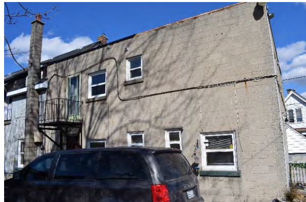
Plate 21: West façade of rear addition, looking east
