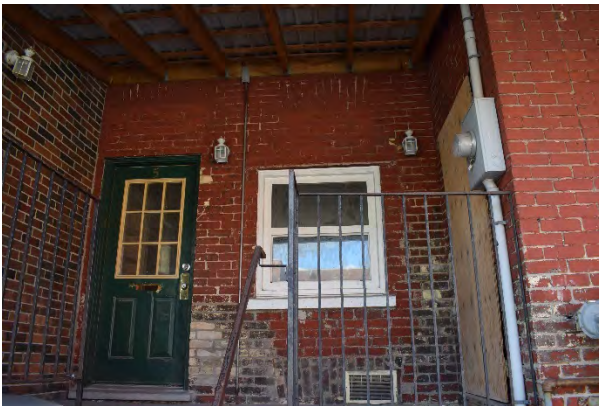
Plate 14: Replacement window and door openings, looking west
