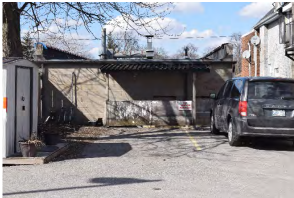
Plate 26: South façade of 735 Dundas Street, looking north
