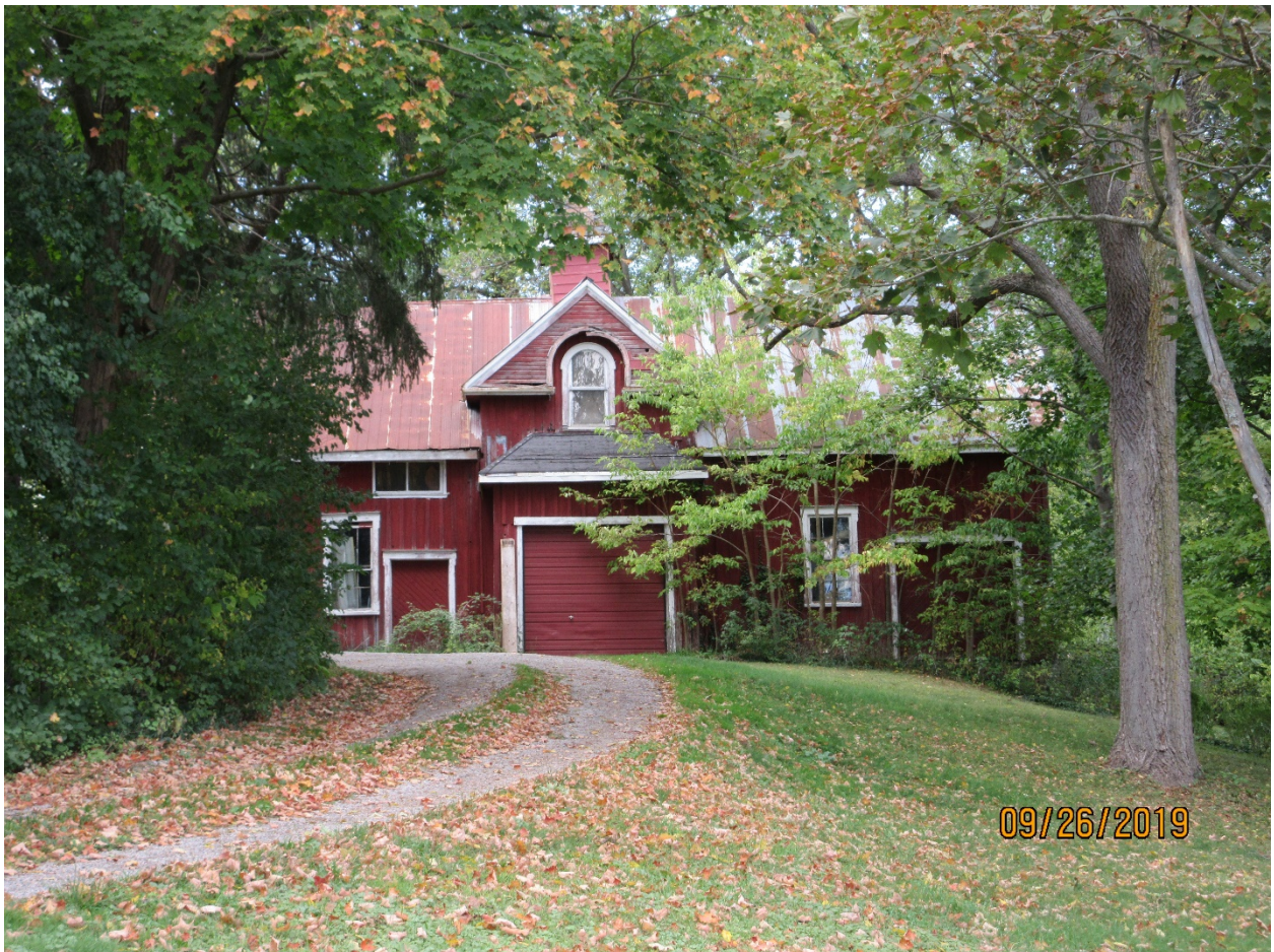
Image 12: Photograph of the east side of the accessory building, September 2019.
