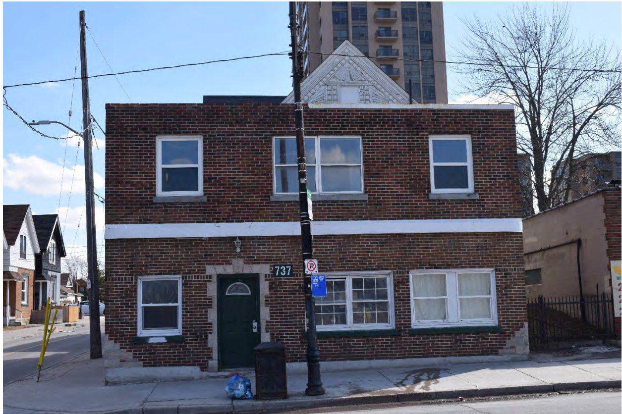
Plate 11: Front (north) façade of 737 Dundas Street, looking south
