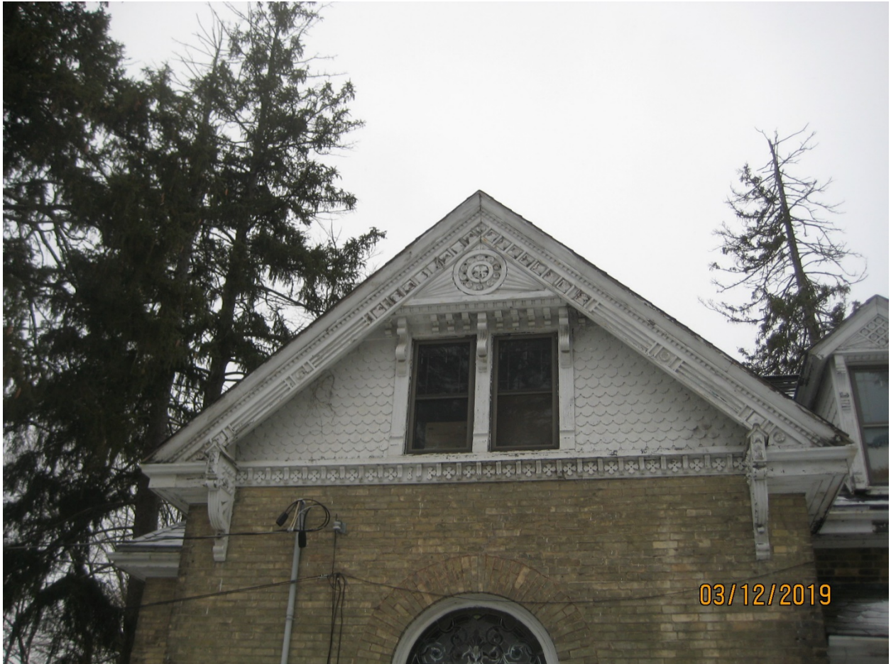
Image 15: Detail showing decorative woodwork in gable on the east elevation of the dwelling, December 2019.
