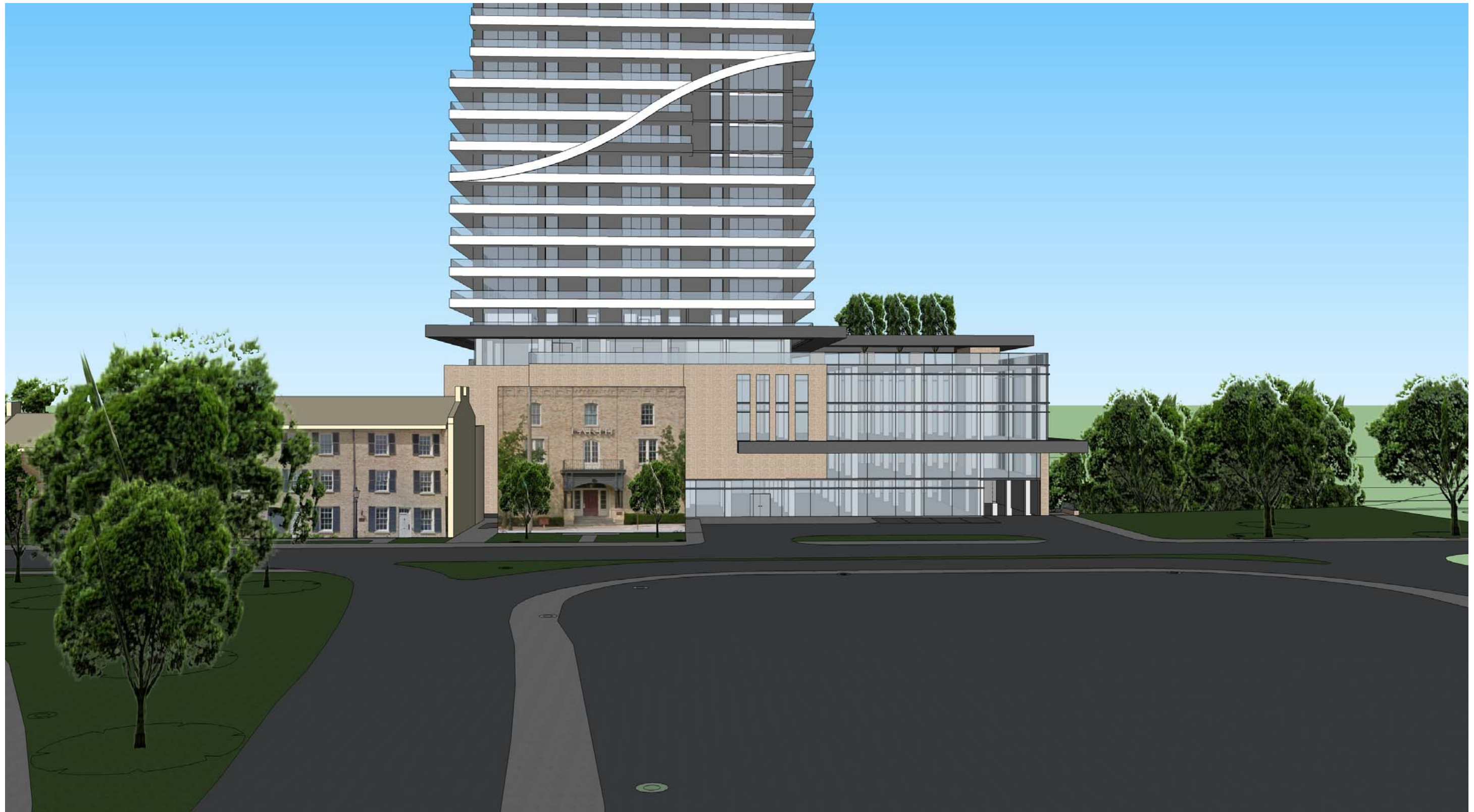
RIDOUT STREET PODIUM ENTRANCE
