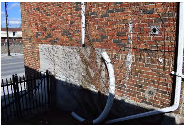
Plate 22: West façade of north addition, looking east
