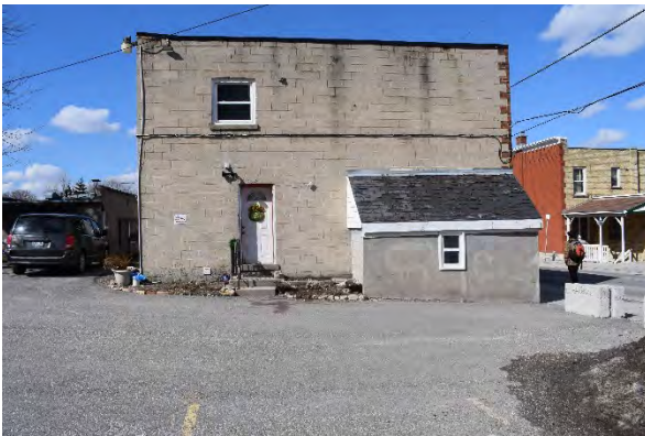
Plate 20: South façade, looking north
