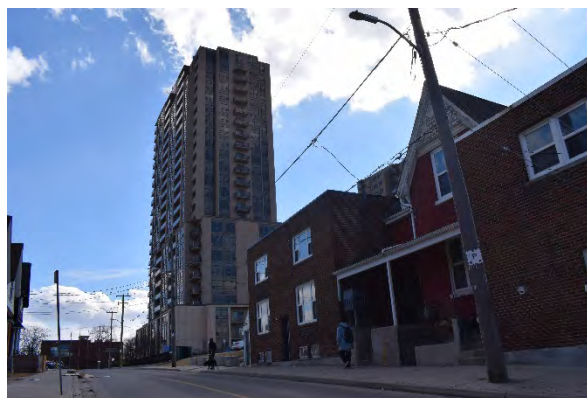
Plate 4: Revo high rise apartment building, looking south
