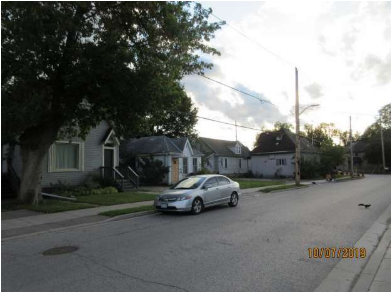
Image 5: View of the south side of Blackfriars Street, looking west towards Wharcliffe Road North including a view of the subject property at 88 Blackfriars Street on October 7, 2019.
