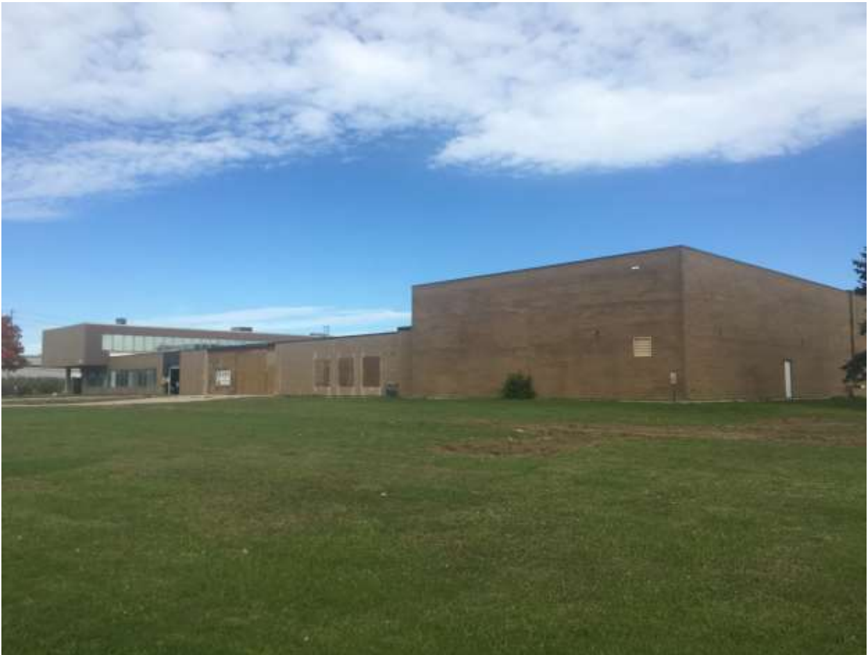
Figure 1: Subject Site (Corner of Wilton Grove Road and Roxburgh Road)
