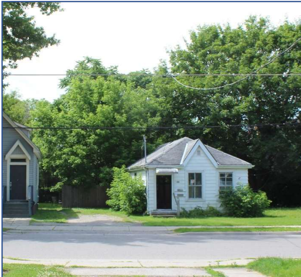
2. No. 88 Blackfriars Street, the subject property. This is identified as a contributing heritage resource to the Blackfriars-Petersville Heritage Conservation District.
