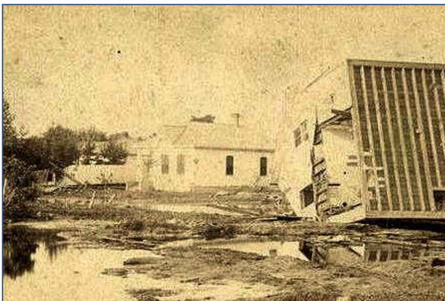
16. This photograph shows the catastrophic damage to homes and property after the flood of 1883. This photograph was taken in the Petersville area. The cottage in the background bears a striking resemblance to 88 Blackfriars Street.
