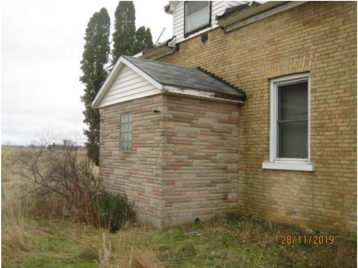
Image 8: View showing front addition on the house. The date of the addition is unclear, however, the exterior is clad with angelstone and vinyl siding.
