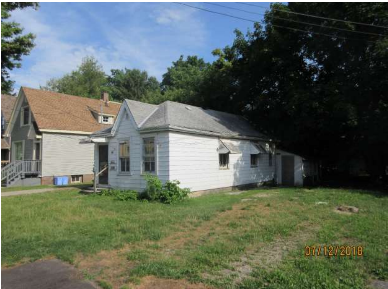
Image 2: View of the main (north) and west elevations of the Contributing Resource at 88 Blackfriars Street on July 12, 2018.
