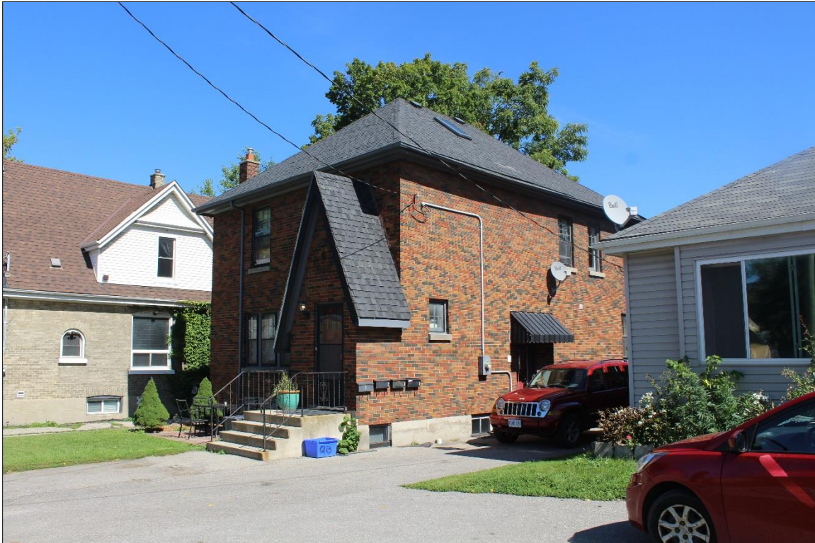
Image 3: South façade of 90 Wellington Road (AECOM, 2019)
