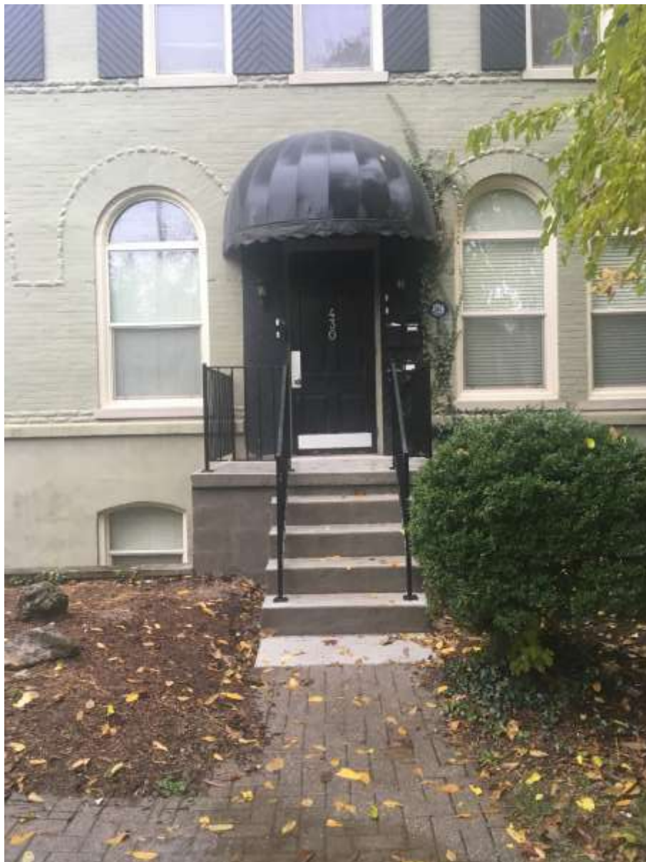
Image 6: Photograph showing the completed alterations to the porch, including re-pouring the concrete and new railings, of the property at 430 Dufferin Avenue (submitted as part of the Heritage Alteration Permit application).
