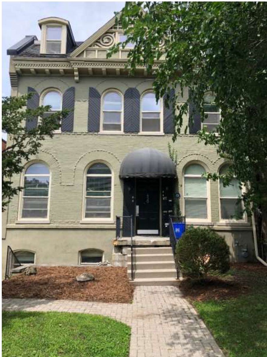
Image 4: Photograph of the property at 430 Dufferin Avenue, showing the porch prior to alteration (submitted as part of the Heritage Alteration Permit application).
