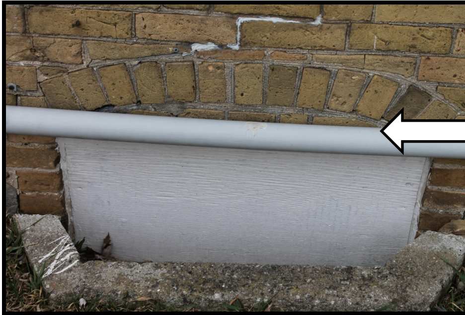
Brick infill in window opening; window boarded up
