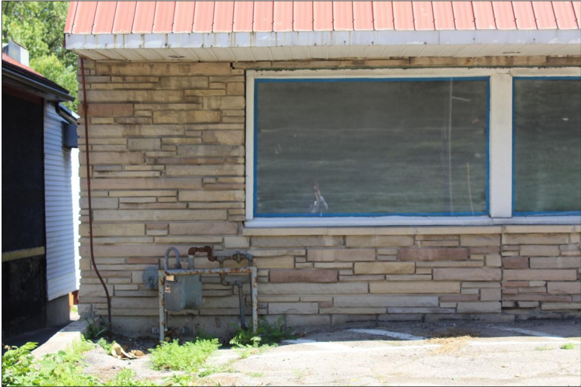
Image 4: Detail of artificial stone cladding on ground floor (AECOM, 2019)
