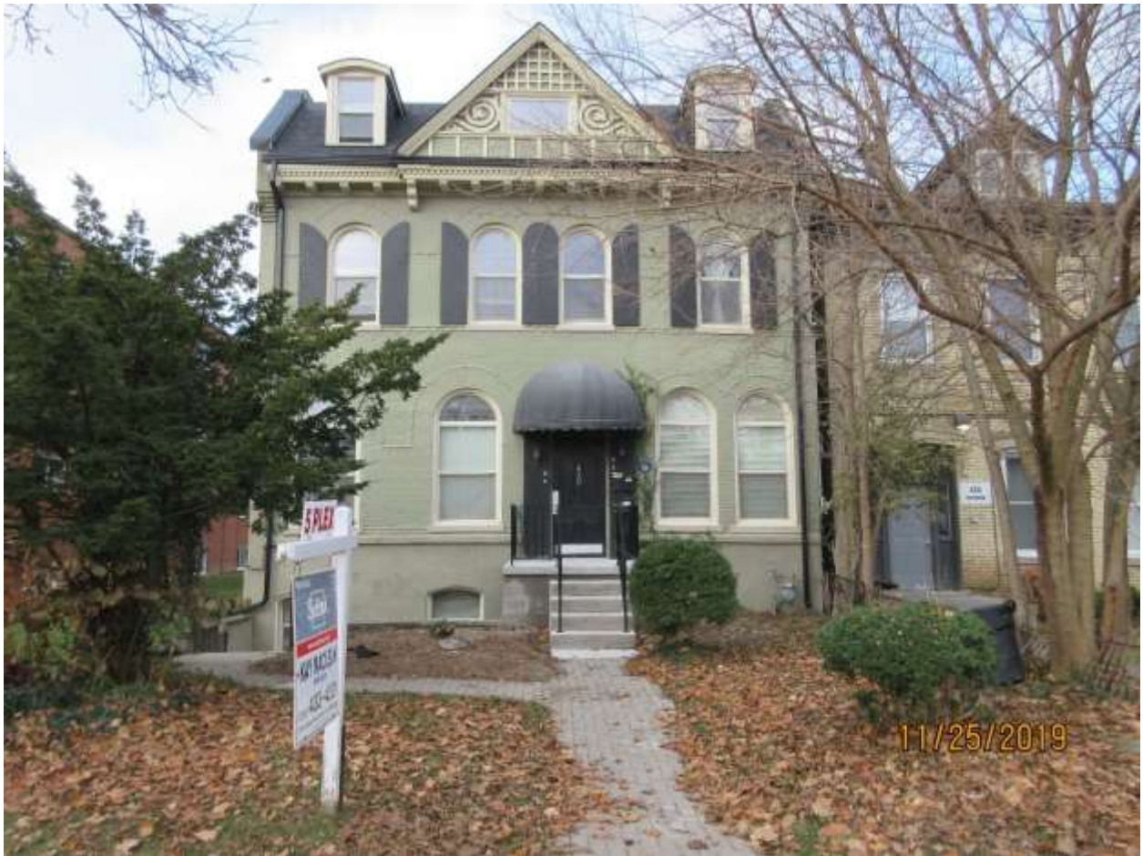
Image 7: Photograph of the property at 430 Dufferin Avenue, with the alterations to the front porch completed.
