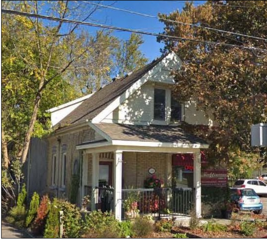
1025 Gainsborough Road - Current
