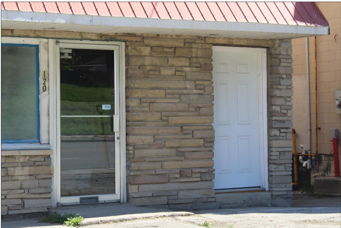
Image 5: Entrance doors on front facade (AECOM, 2019)
