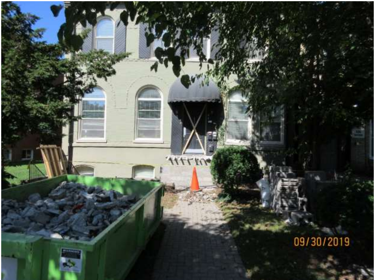
Image 5: Photograph of the property at 430 Dufferin Avenue on September 30, 2019 showing work underway.
