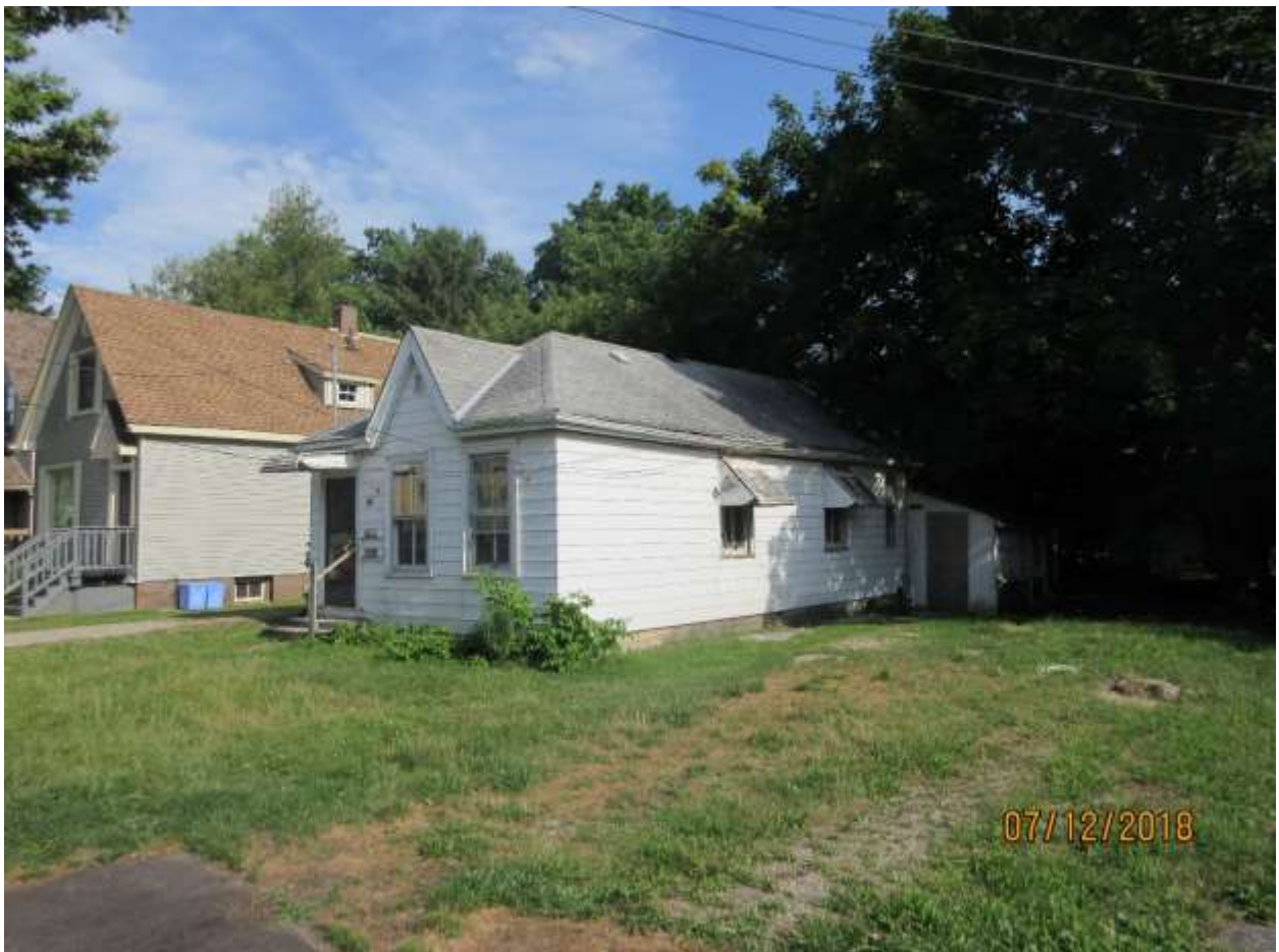
Image 2: View of the main (north) and west elevations of the Contributing Resource at 88 Blackfriars Street on July 12, 2018.
