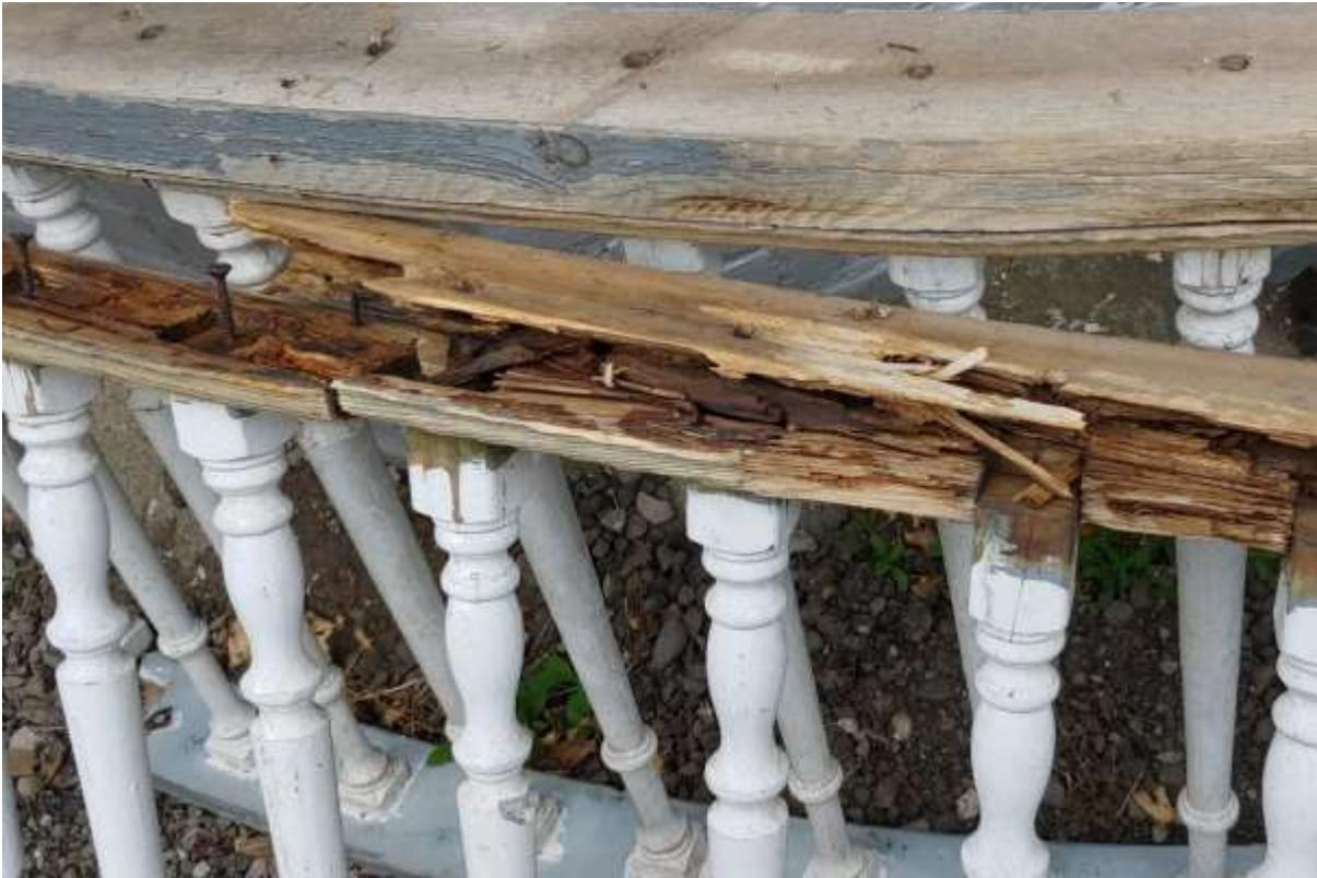
*Image 3: Detail of the top and bottom rails on the porch at 906 Lorne Avenue submitted as a part of the Heritage Alteration Permit application, showing the deteriorated wooden elements (October 2019).*
