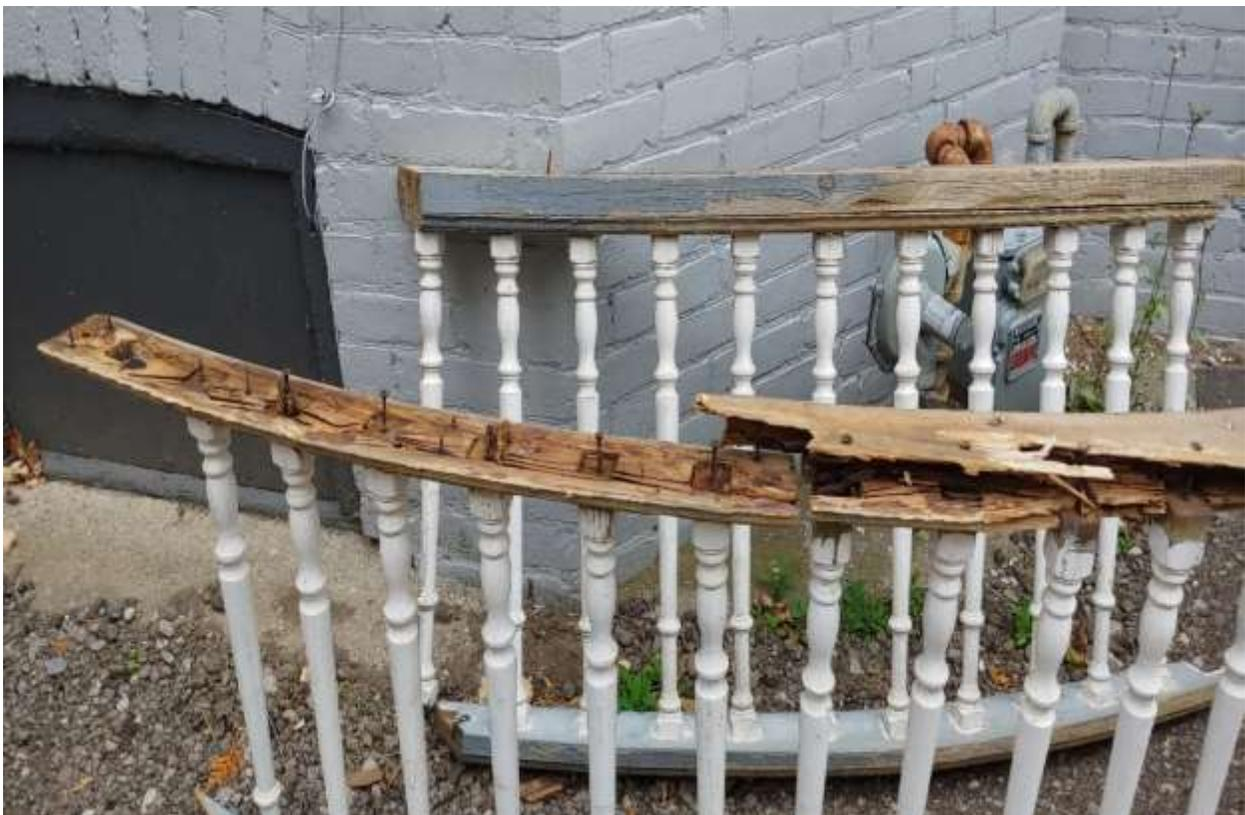
*Image 4: Photograph of the top and bottom rails on the porch at 906 Lorne Avenue submitted as a part of the Heritage Alteration Permit, showing the deteriorated wooden elements (October 2019). Note, the railings are sitting upside down so the rotted bottom rail is most visible in the photograph.*
