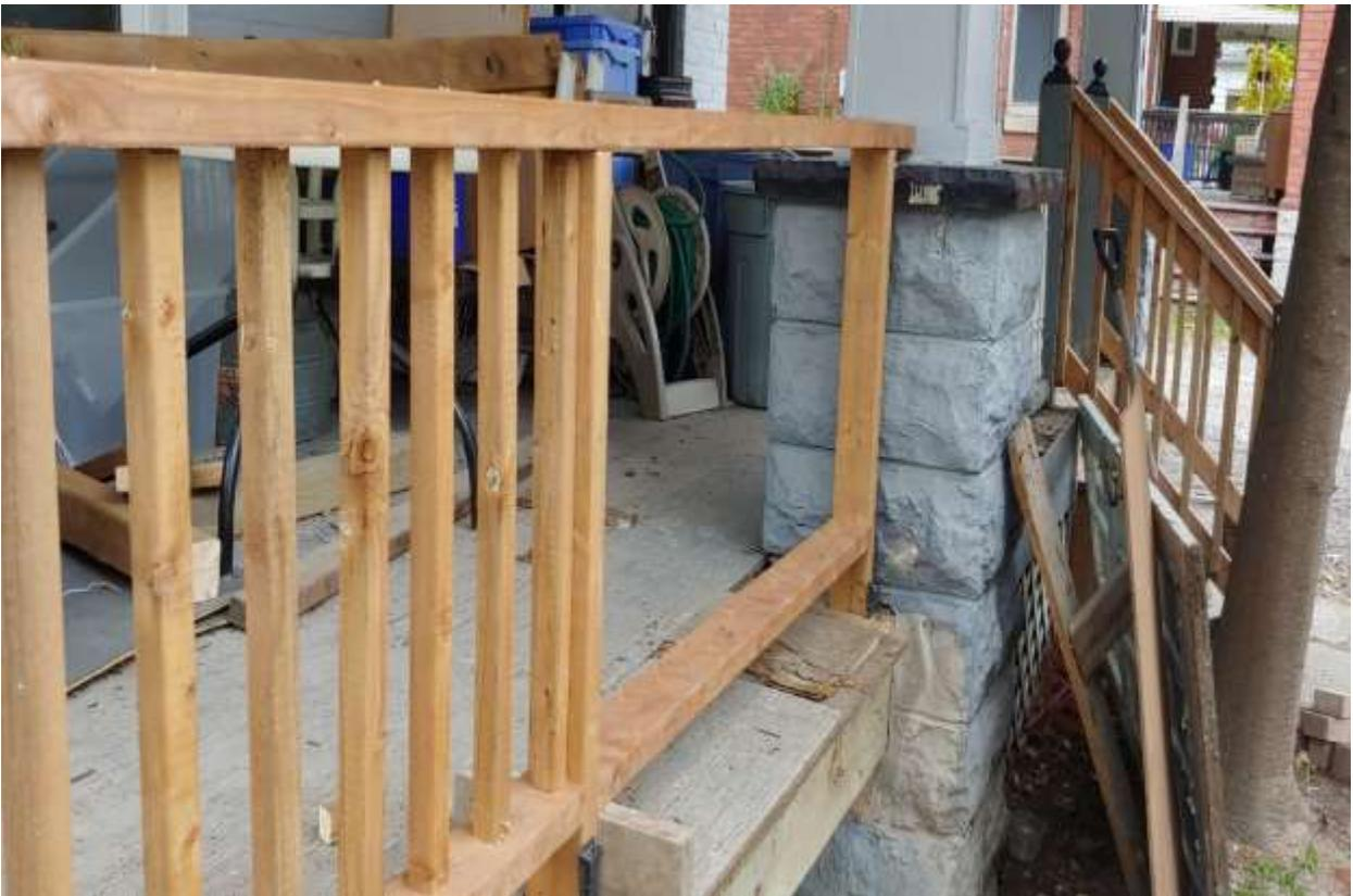
*Image 6: Photograph showing proposed railing and square spindle alterations to the porch at 906 Lorne Avenue, submitted as a part of the Heritage Alteration Permit application (October 2019). Note, the new height of the top rail will be required in order to meet the requirements of the Ontario Building Code.*
