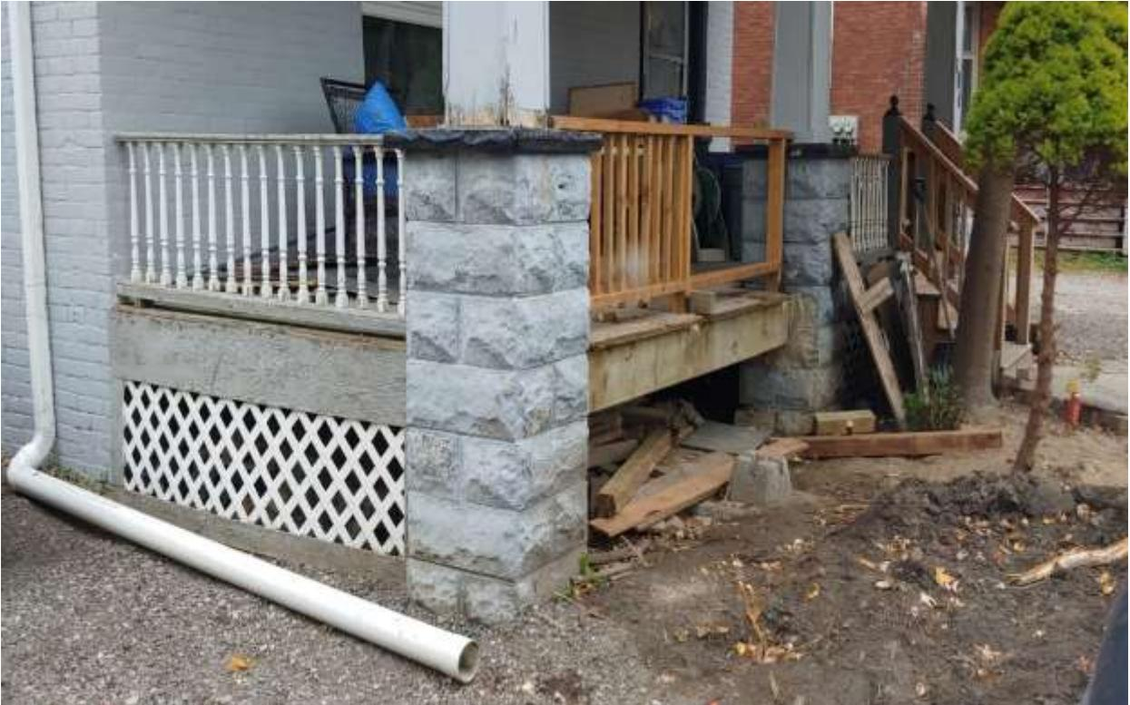
*Image 5: Photograph showing the unapproved alterations underway at 906 Lorne Avenue submitted as a part of the Heritage Alteration Permit application. The existing railing and square spindles are shown on the left, and the proposed replacement railings are shown on the right of the post (October 2019). Note, a new lattice porch skirt and base of the column should be added as a part of the Heritage Alteration Permit.*
