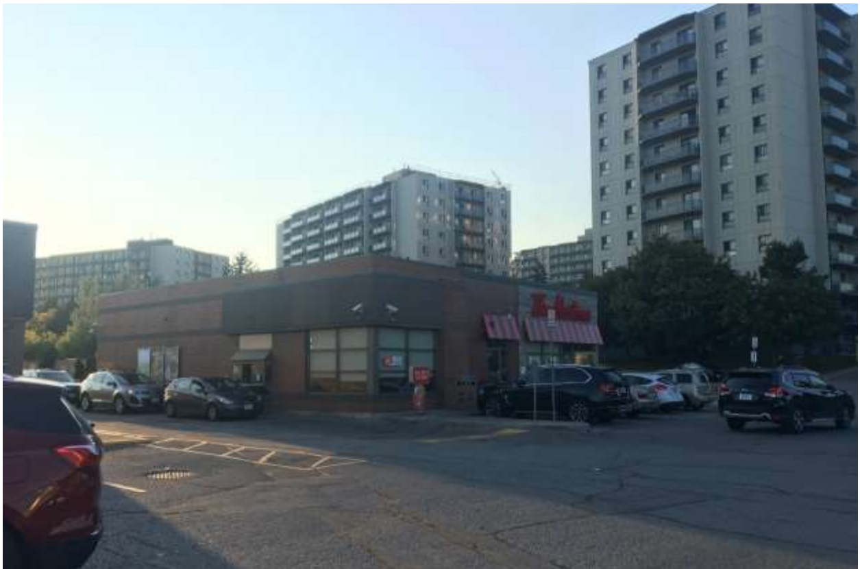
Figure 2: Second building located on the subject site
