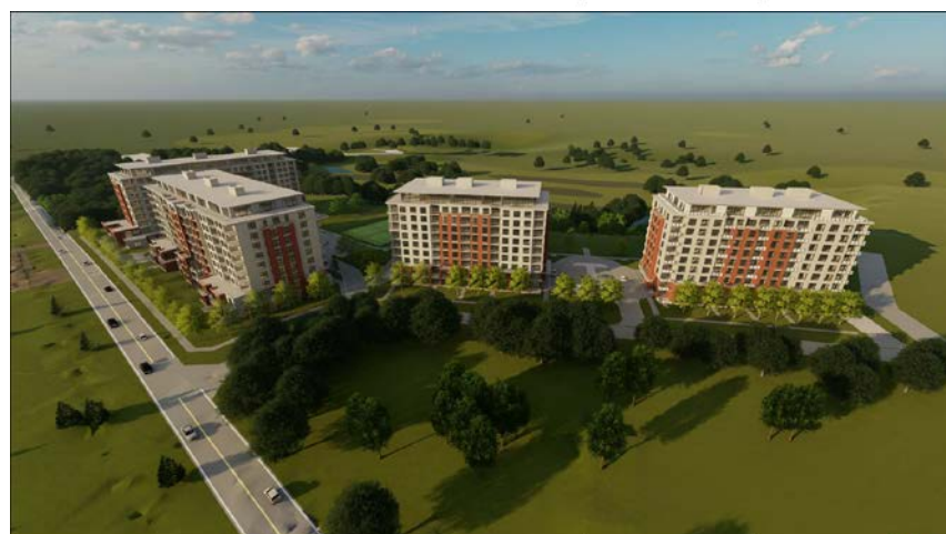
AERIAL VIEW - OVERALL 420, 440, 460, 480 CALLAWAY ROAD LONDON, ON
