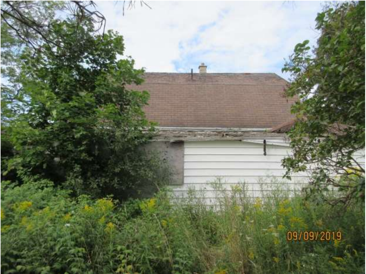
Image 5: Rear (east) façade of the dwelling at 6100 White Oak Road.
