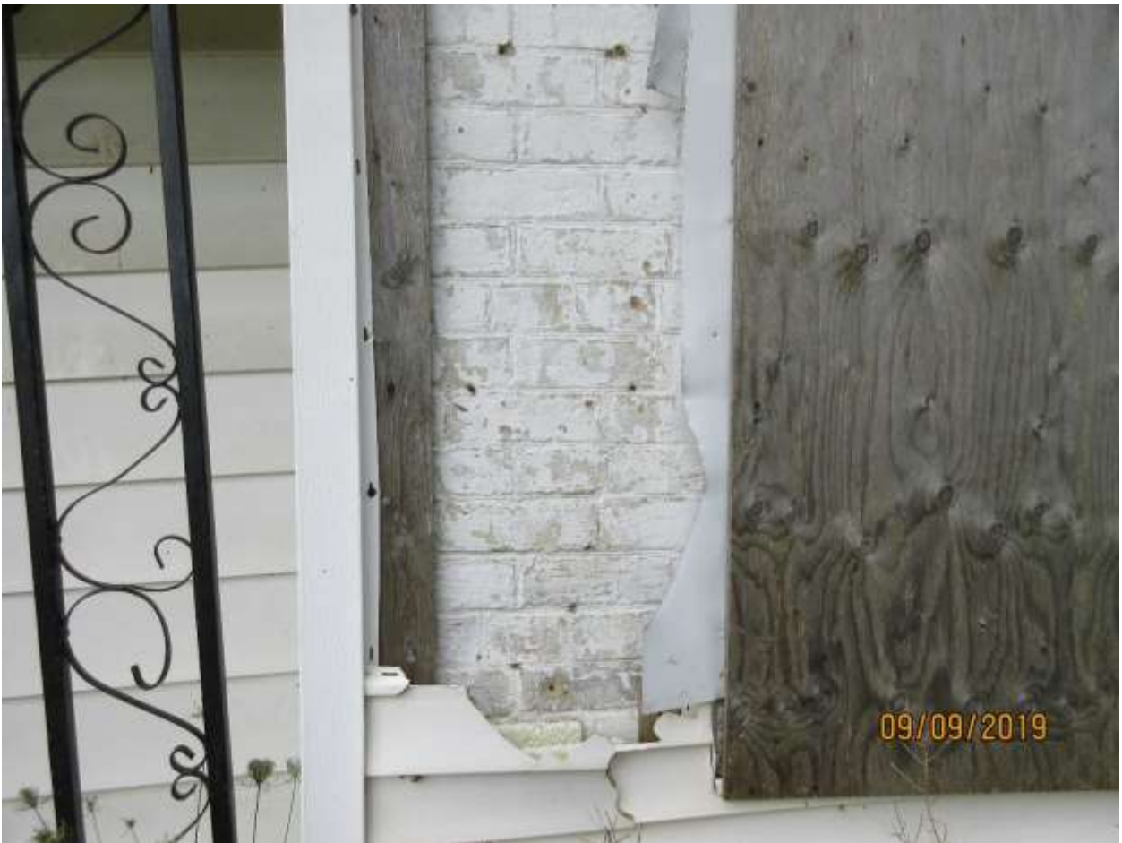
Image 6: Detail of the brickwork, underneath the existing vinyl siding. The brick work appears to be buff brick, with several layers of paint applied. The brickwork appears to be laid in a common bond pattern. The brickwork appears to extend to the ground level, however board cladding prevented the confirmation of this detail.
