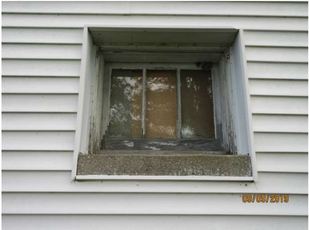
Image 7: The above pictured window on the south façade of the dwelling at 6100 White Oak Road is the only main storey window that is not secured from the exterior (it is boarded from the interior). Also note the concrete window sill.
