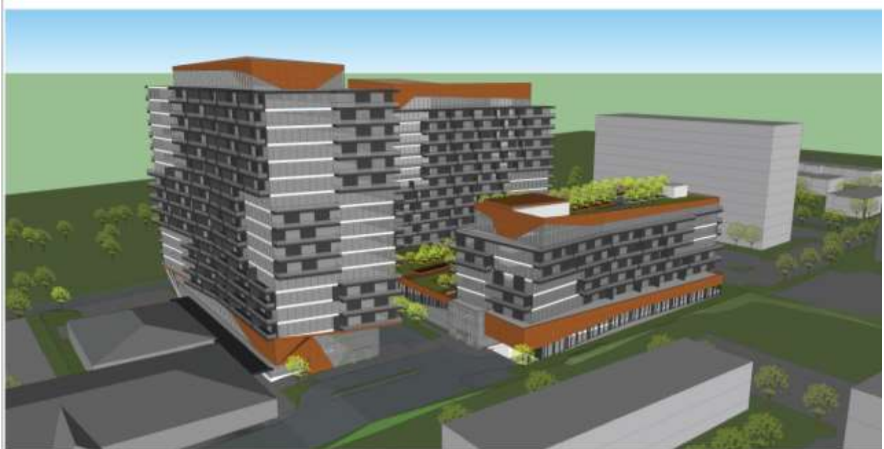
Aerial View Looking Southeast
