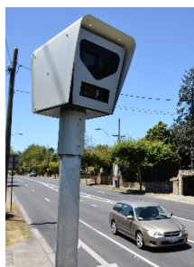
Figure 1: Semi-Fixed ASE Installation
