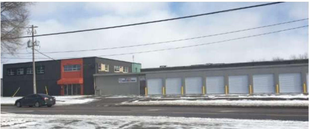
Figure 4: 600 Third Street (east side) looking east
