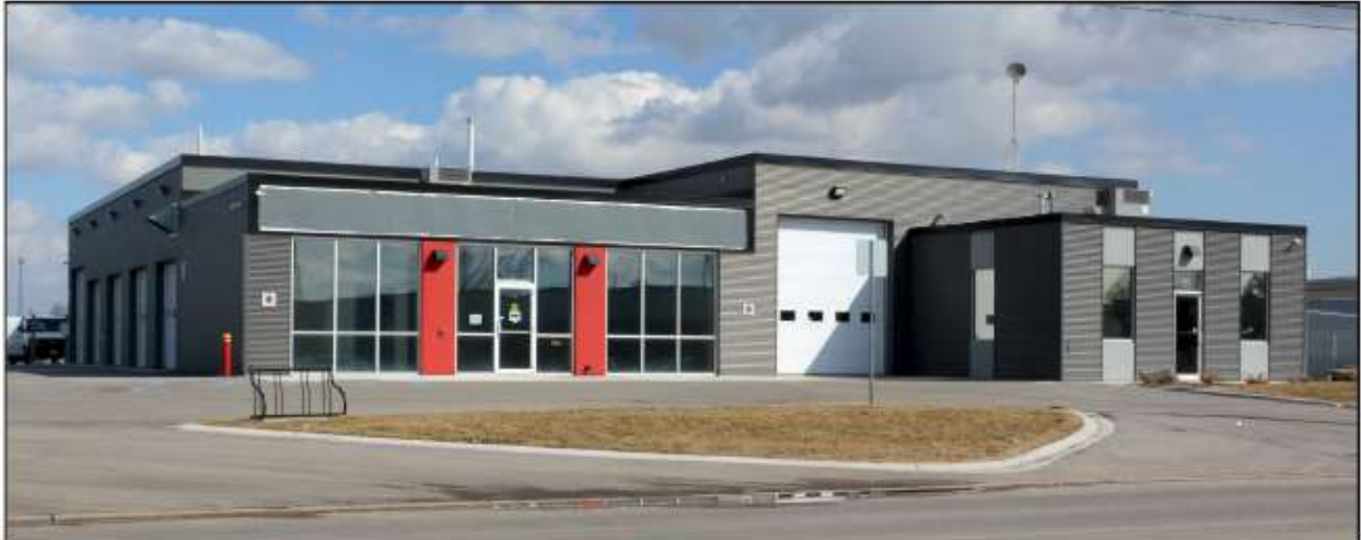
Figure 1 – View of building from the street, showing new addition with garages
