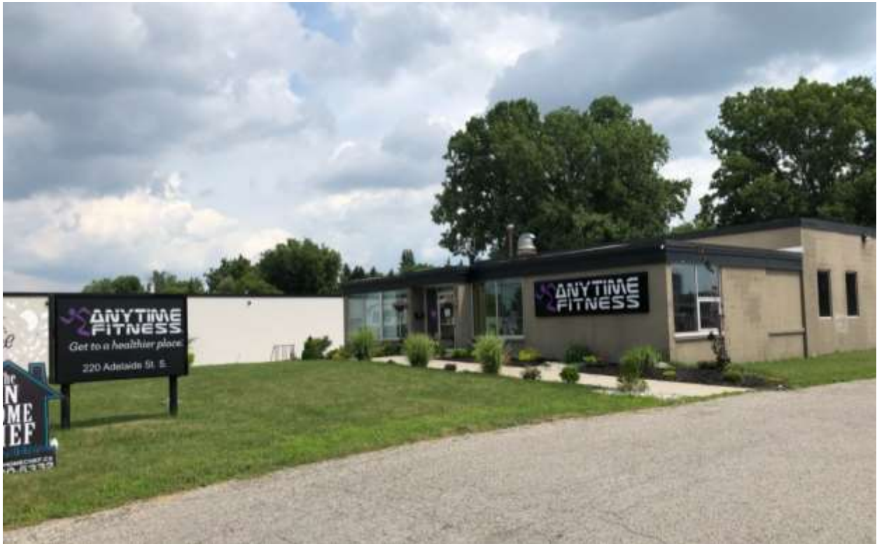
Figure 1: 220 Adelaide Street South
