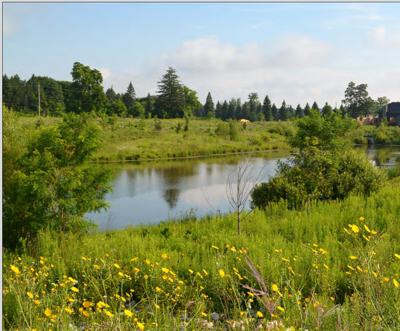
Stormwater Management Facility – Sunningdale Road W.
