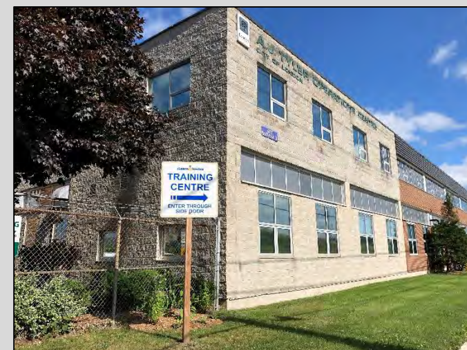
A.J. Tyler Operation Centre – Bathurst Street
