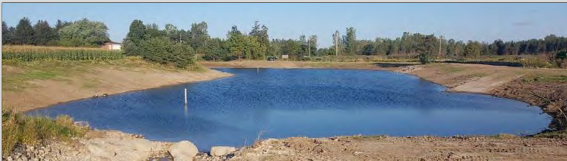
Stormwater Management Facility
