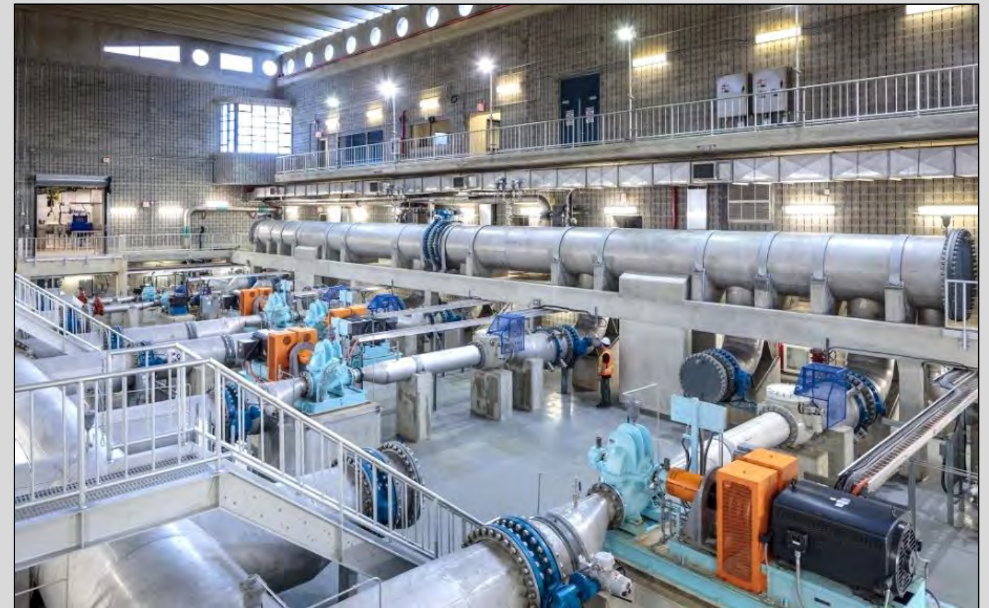
South East Reservoir Interior – Highbury Ave. S
