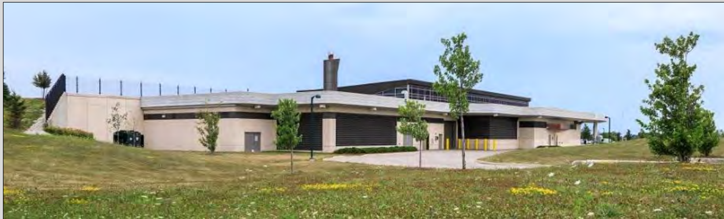
South East Reservoir Exterior – Highbury Ave. S
