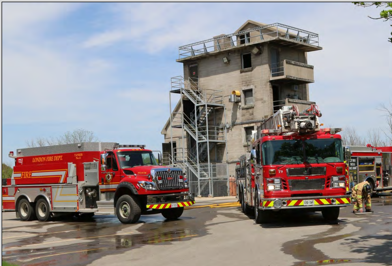
Training Tower – Fire Station # 9
