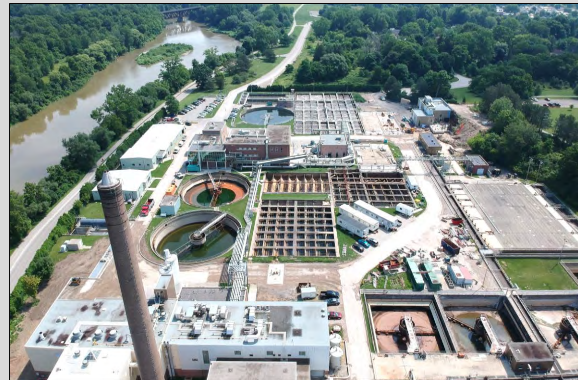
Greenway Wastewater Treatment Plant – Greenside Ave.
