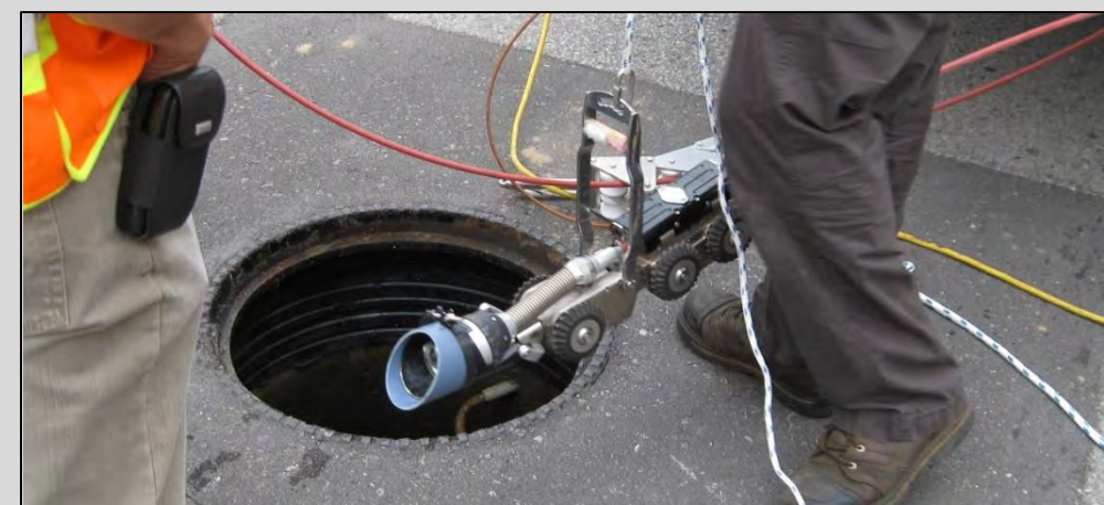
Inspection and Condition Assessment using CCTV
