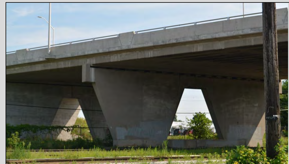
Bridge on Highbury Ave N
