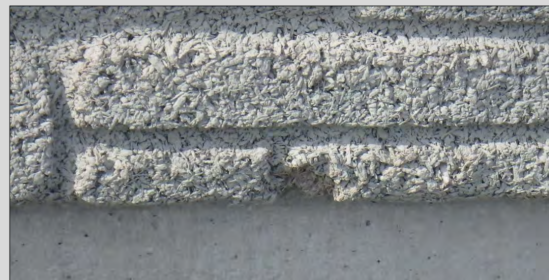
Spalling - Noisewall
