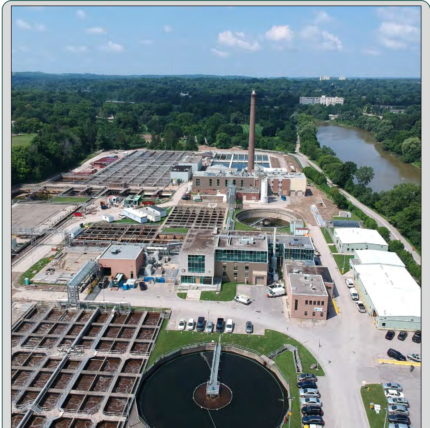
Greenway Wastewater Treatment Plant – Greenside Ave.
