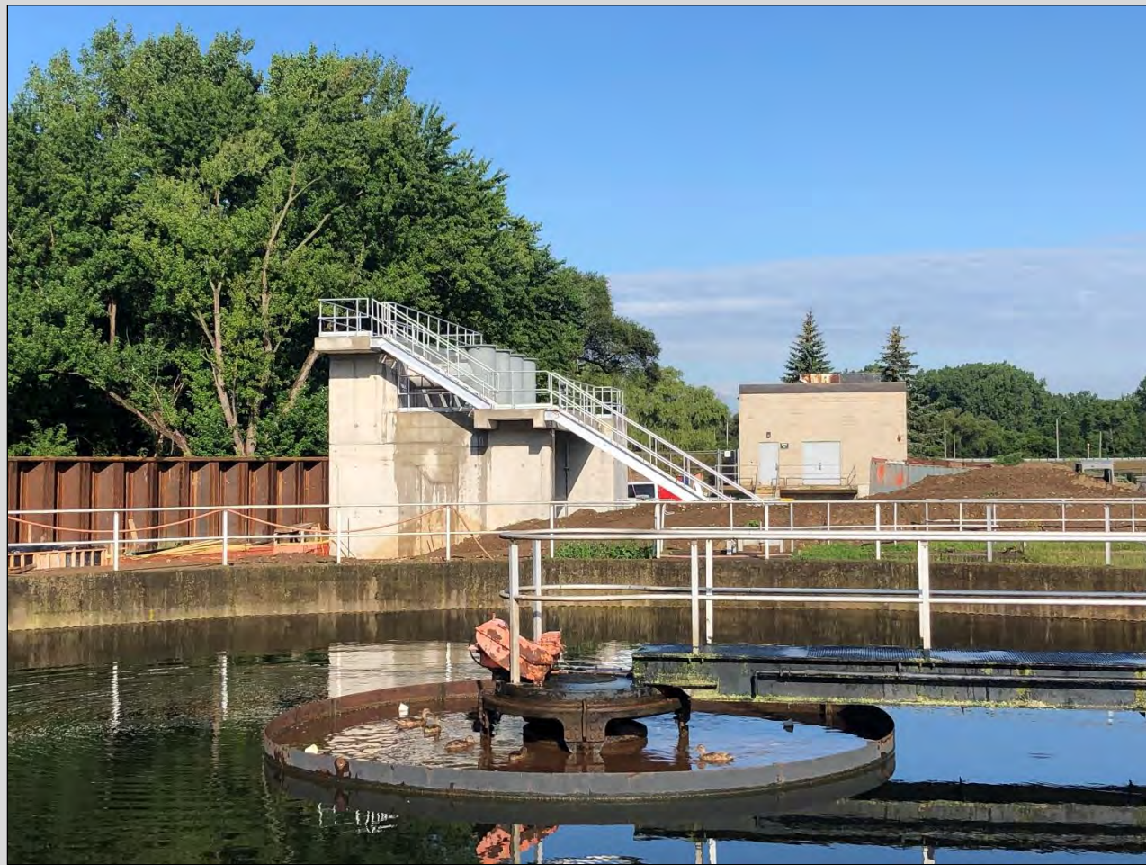
Effluent Pumping Station at Vauxhall Wastewater Treatment Plant – Price Street
