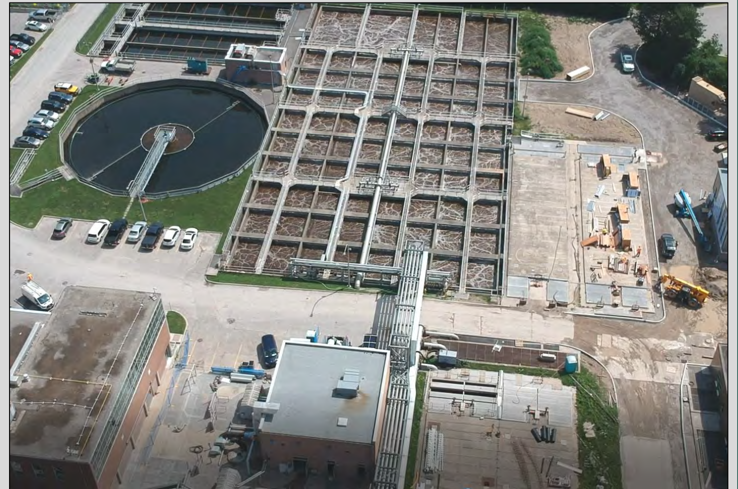
Greenway Wastewater Treatment Plant – Greenside Ave.
