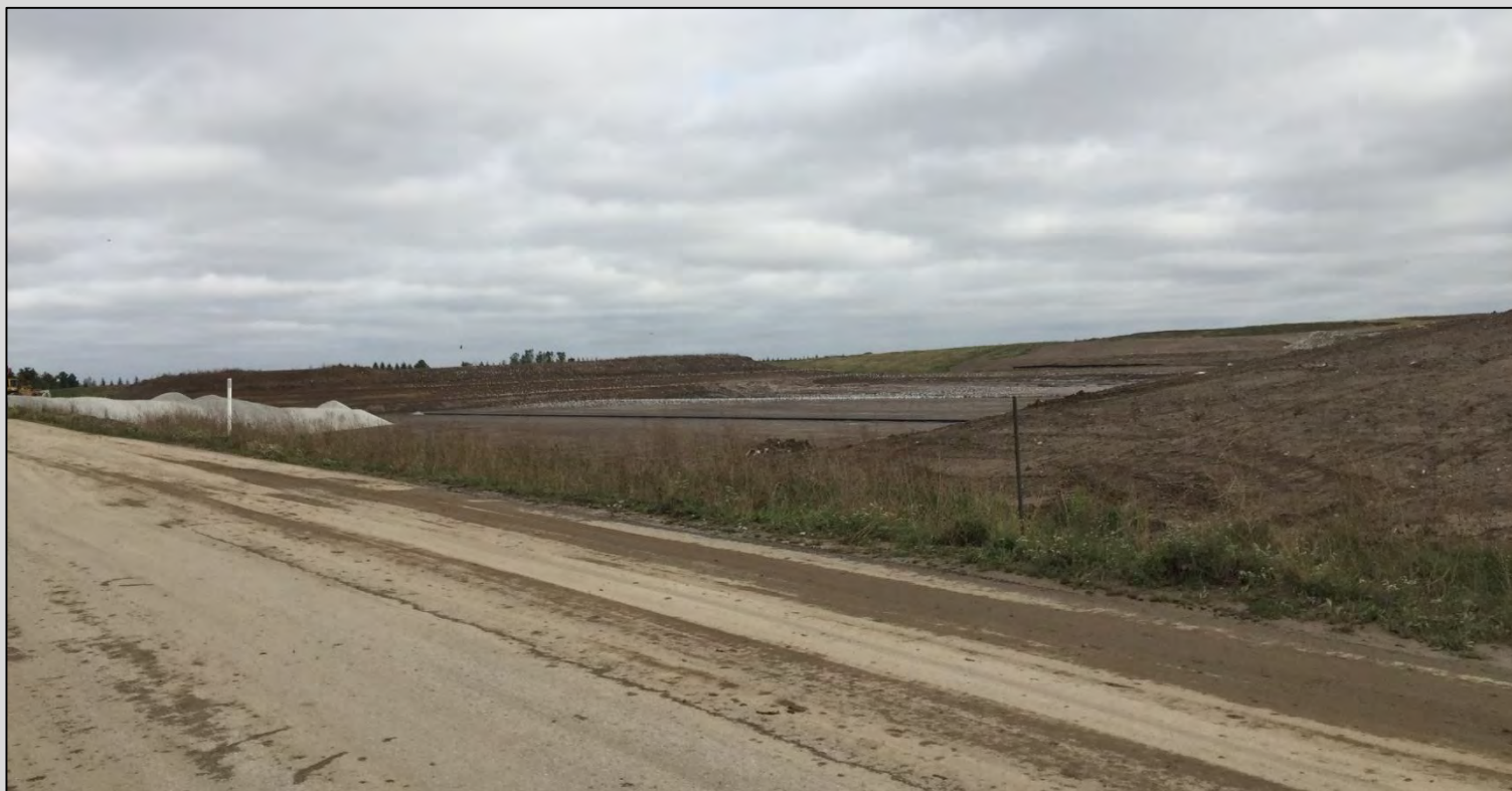
W12A Cell Construction
