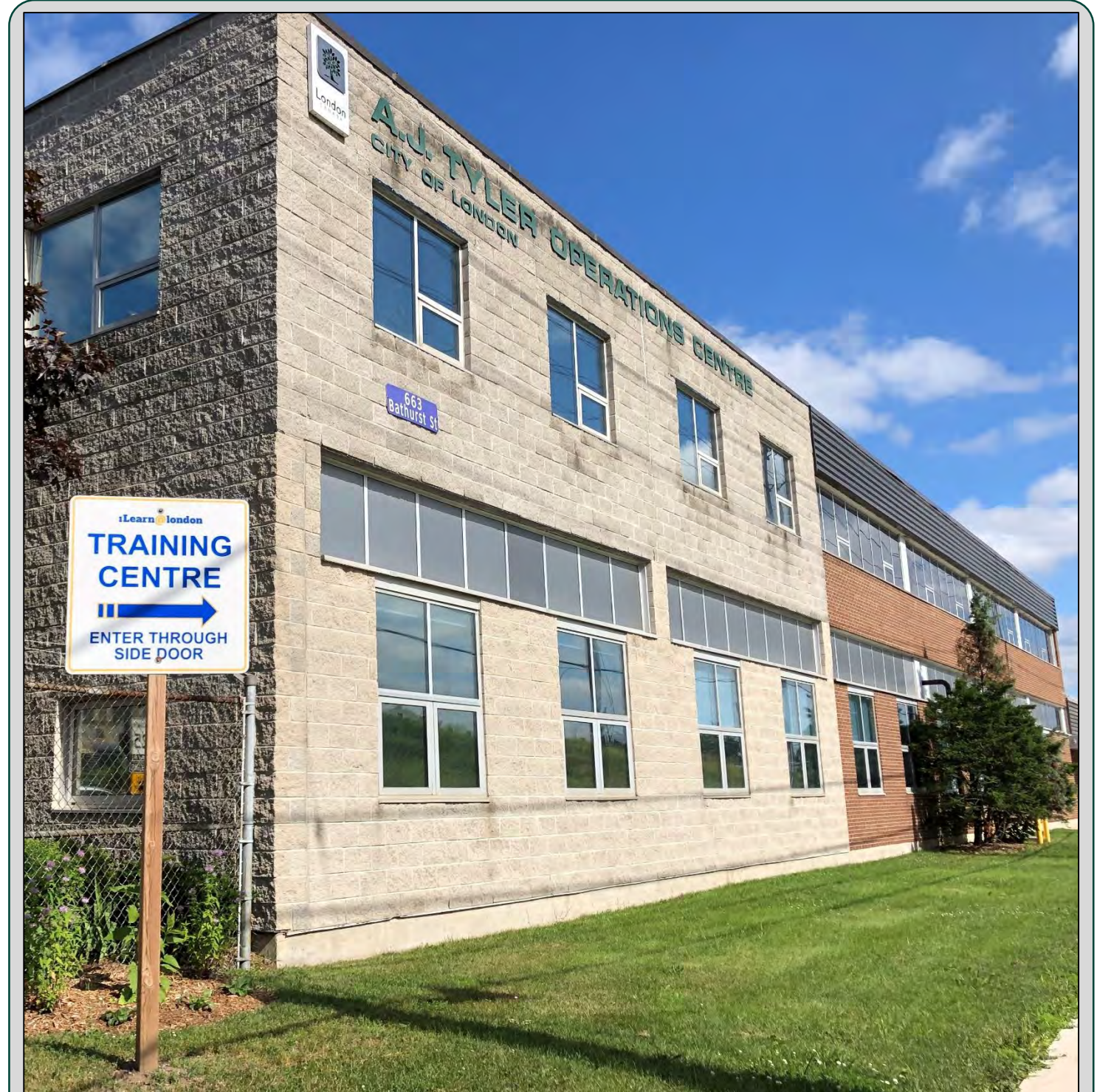
A.J. Tyler Operations Centre – Bathurst Street
