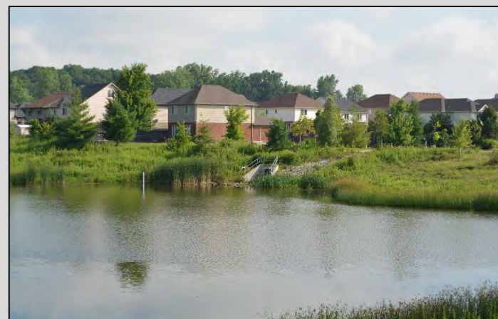
Stormwater Management Pond – Sunningdale Rd
