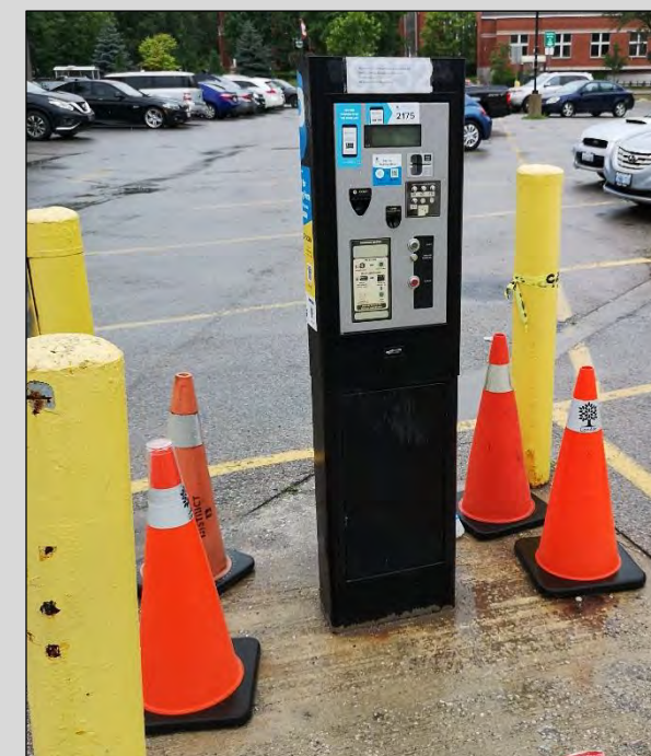
Parking Meter in Deteriorating Condition
