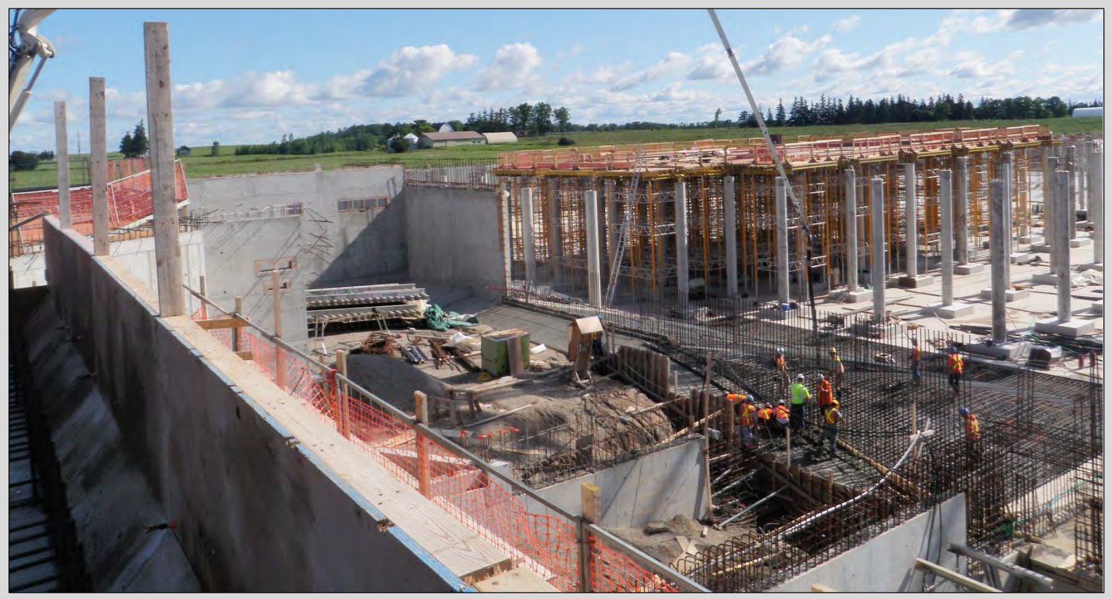
Construction of South East Reservoir
