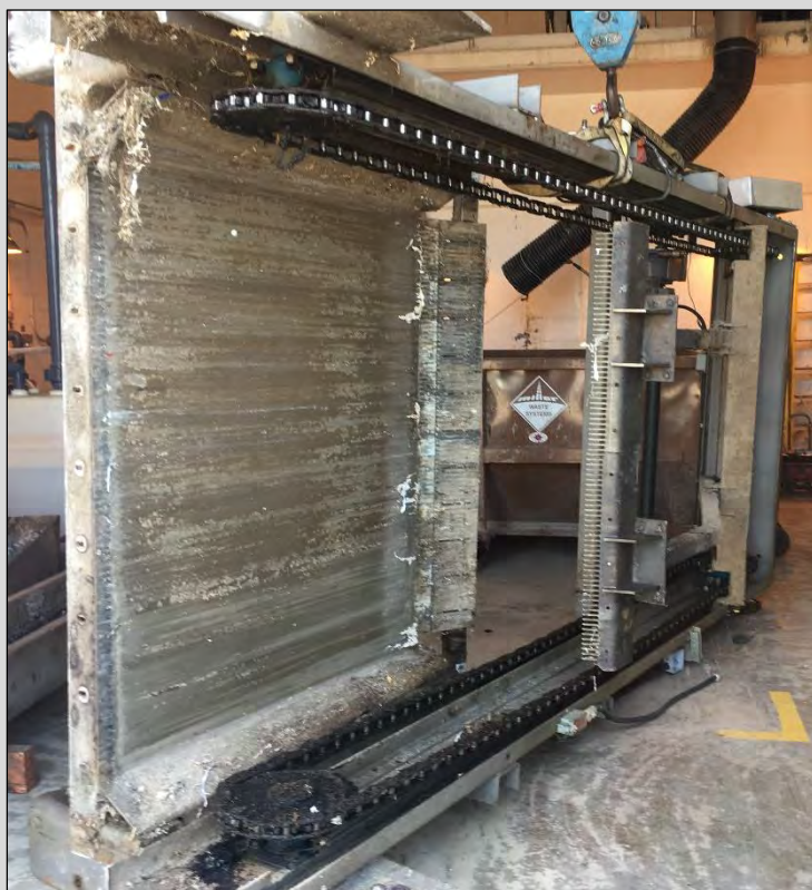
Replaced Screen at Adelaide Wastewater Treatment Plant
