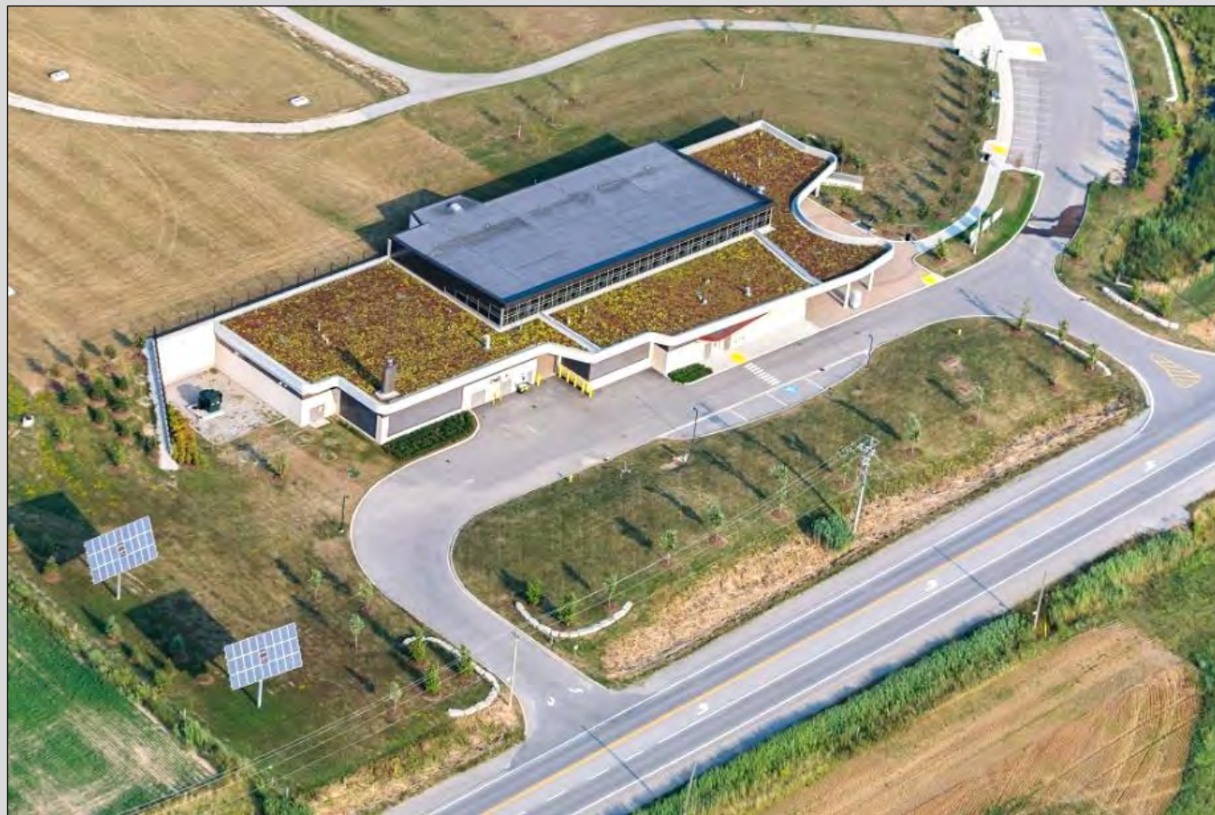
South East Reservoir – Highbury Ave. S
