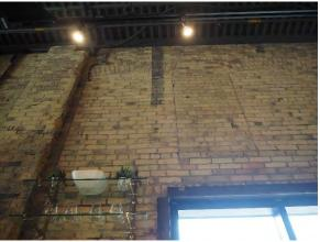
Plate 20: Interior brick wall and bricked up windows on south elevation of 1 Bathurst Street, looking south.
