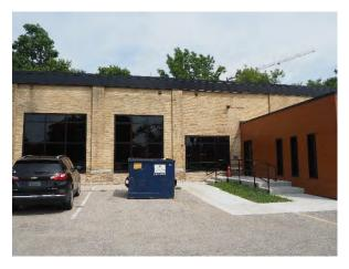
Plate 13: South elevation of 1 Bathurst Street showing buff brick and metal flashing, looking north.
