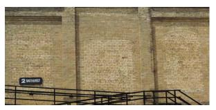
Plate 27: Bricked in windows and soldier arch on east elevation of 2
