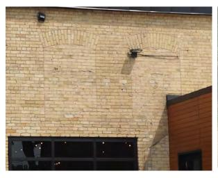
Plate 17: Segmental arch window openings and soldier arch, south elevation of 1 Bathurst Street, looking north.
