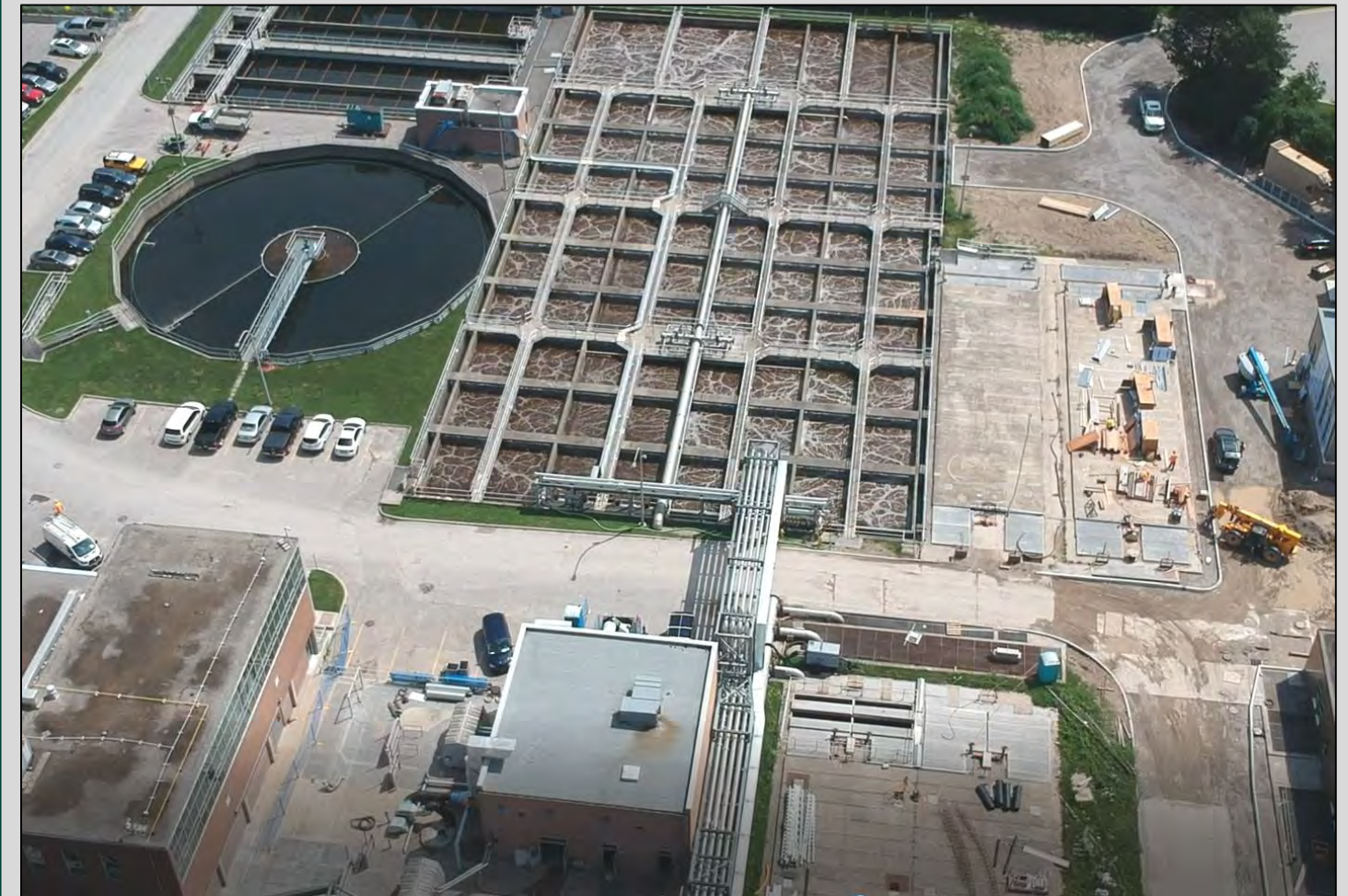
Greenway Wastewater Treatment Plant – Greenside Ave.
