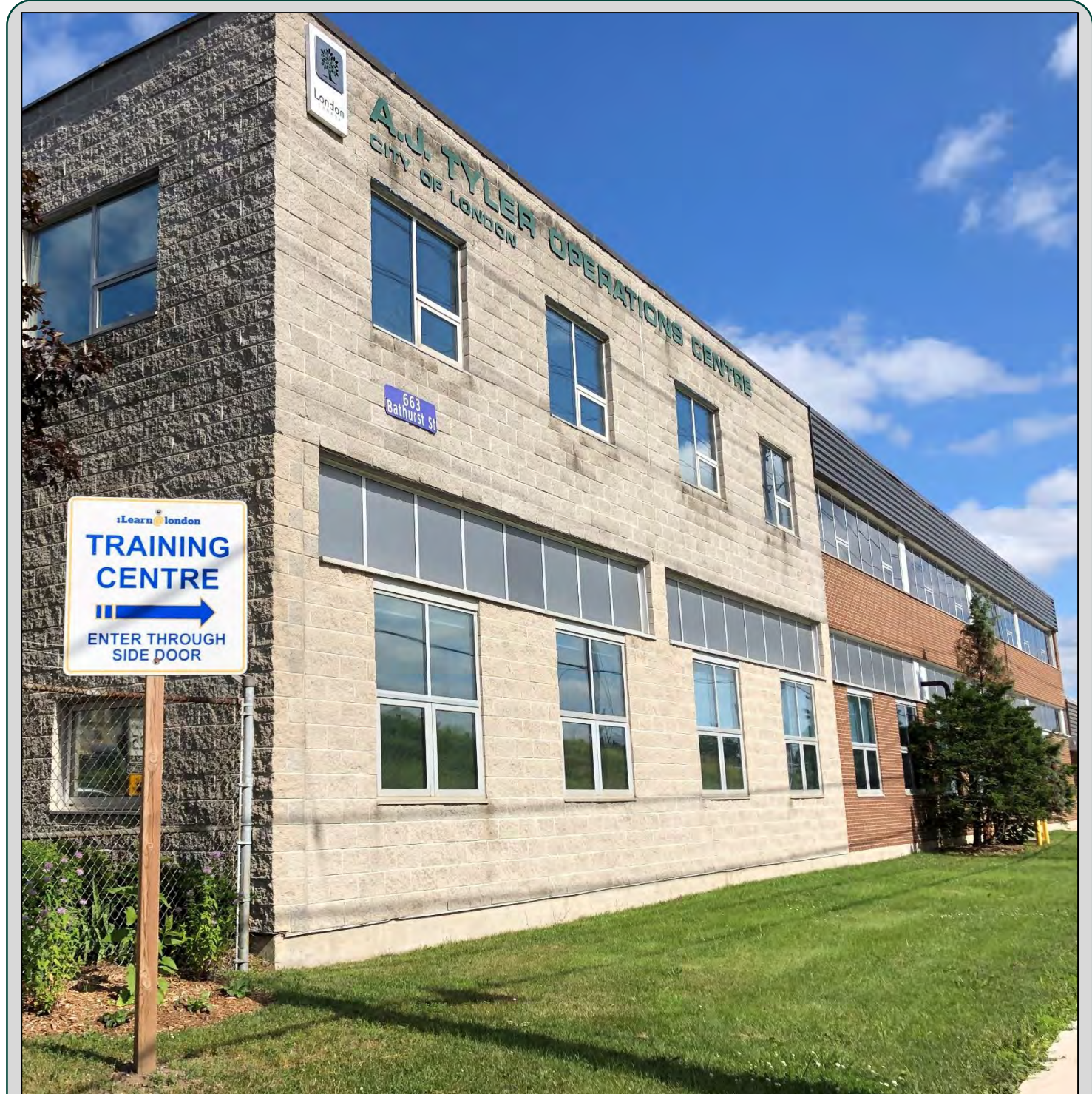
A.J. Tyler Operations Centre – Bathurst Street
