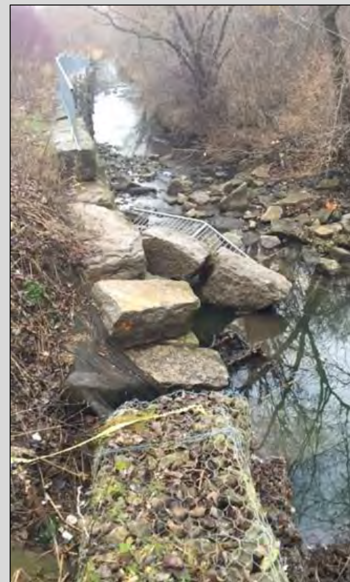
Channel Before Restoration work
