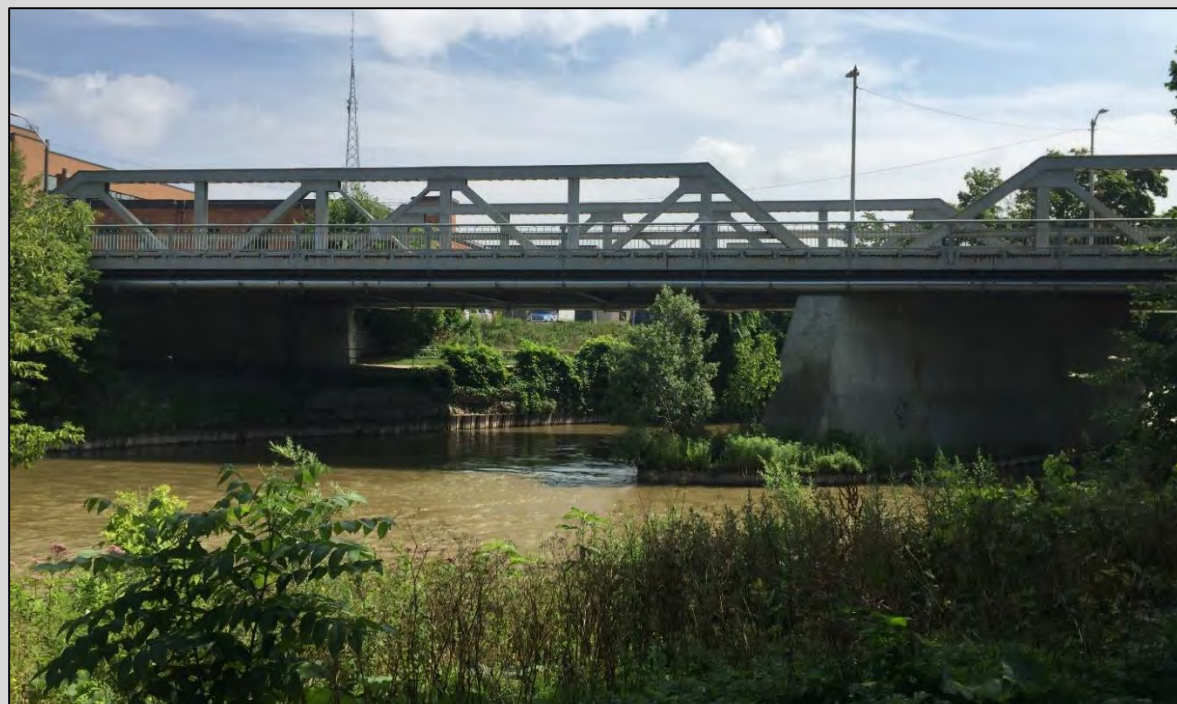
Bridge at Ridout St N
