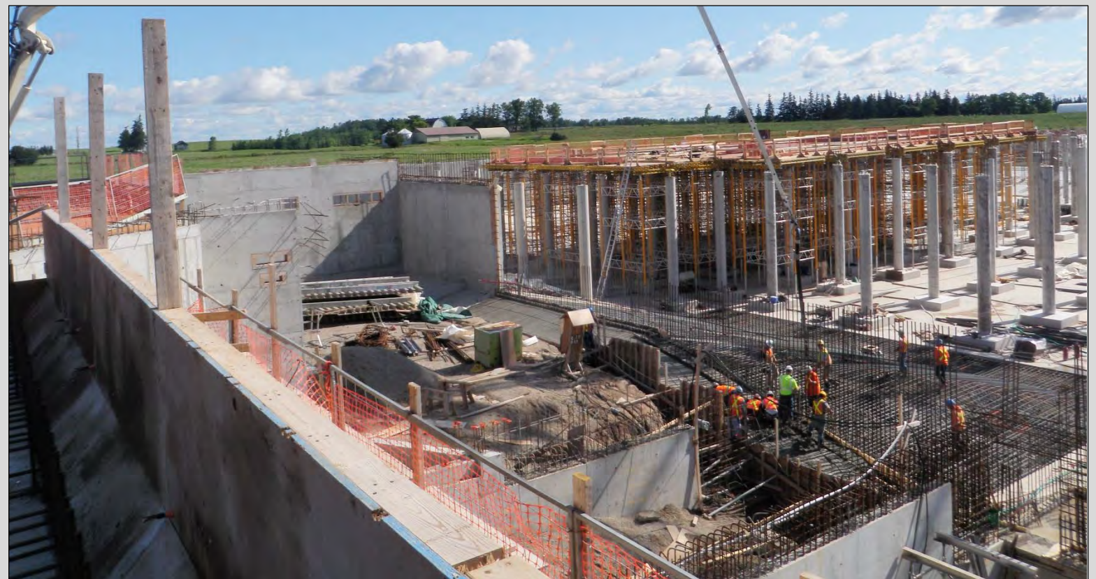
Construction of South East Reservoir
