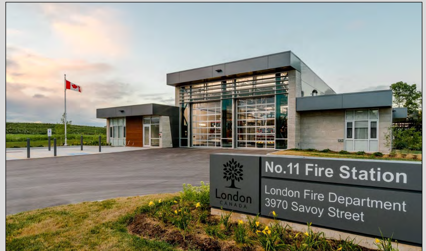
Fire Station # 11 – Savoy street
