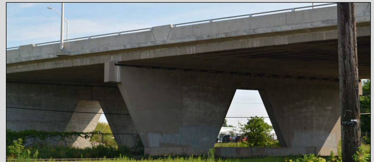
Bridge - Highbury Avenue Overhead at CN Rail
