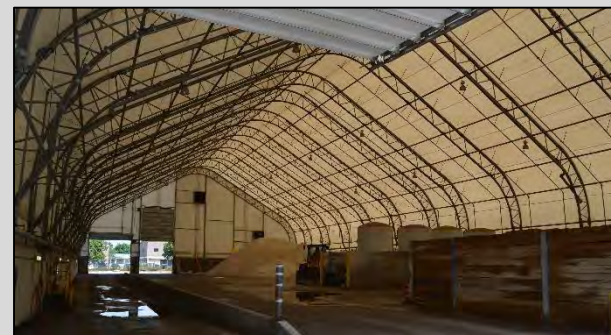
Sand/Salt Dome – Exeter Operation Centre
