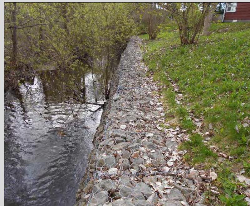
Bridge Gabion Baskets
