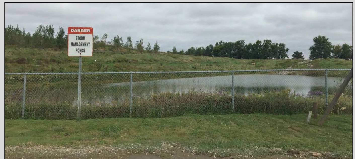
Stormwater Management Pond at W12A Site
