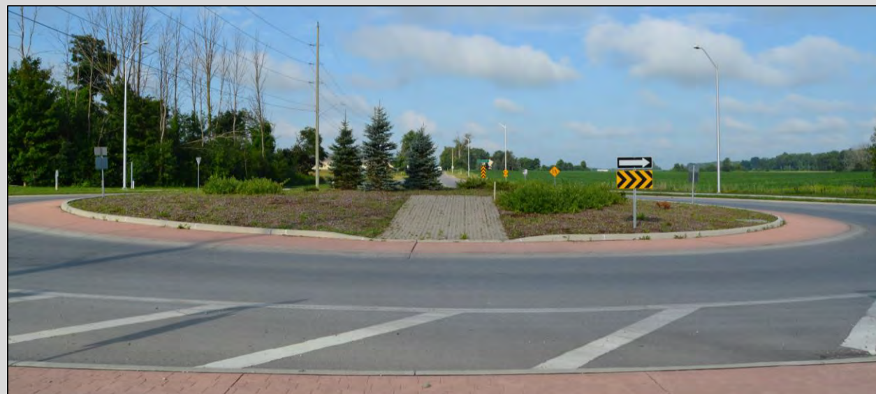
Wonderland Road N and Sunningdale Road W. Intersection
