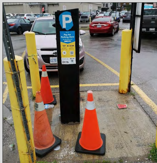
Parking Meter in Deteriorating Condition
