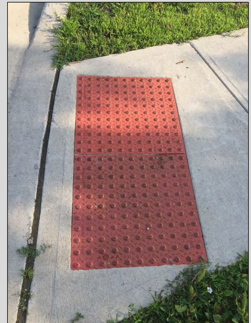
Sidewalk tactile paving
