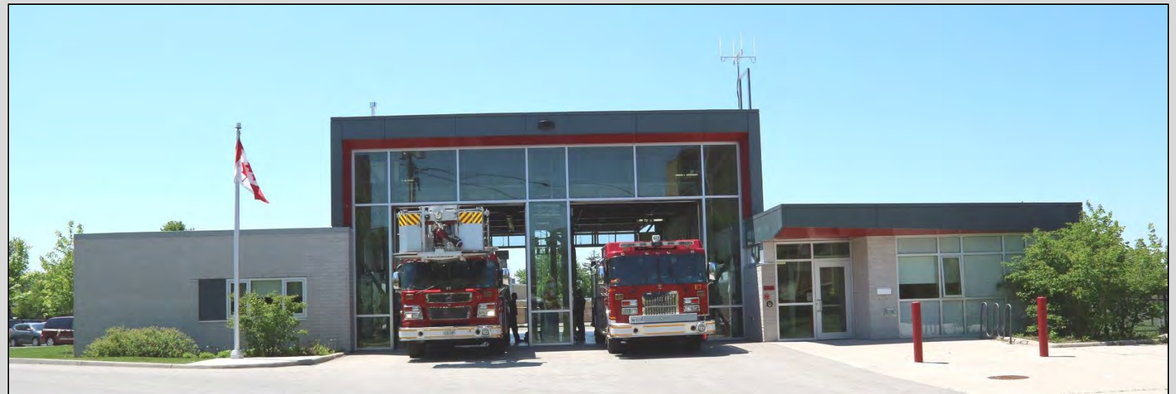
Fire Station # 7 – Webster street
