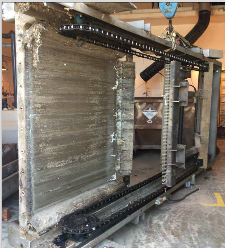
Replaced Screen at Adelaide Wastewater Treatment Plant
