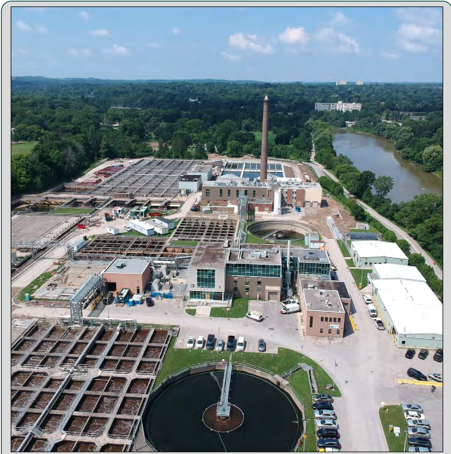
Greenway Wastewater Treatment Plant – Greenside Ave.
