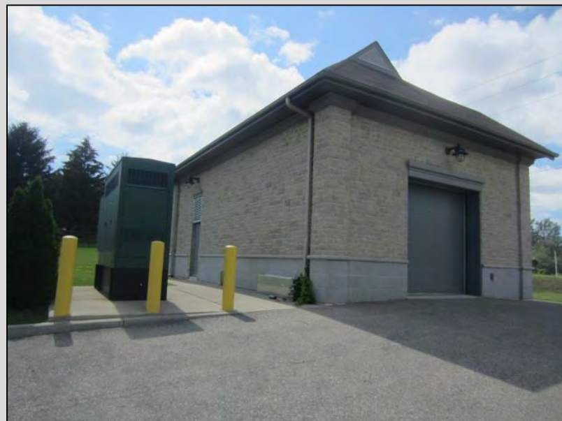
Sunningdale Water Pumping Station
