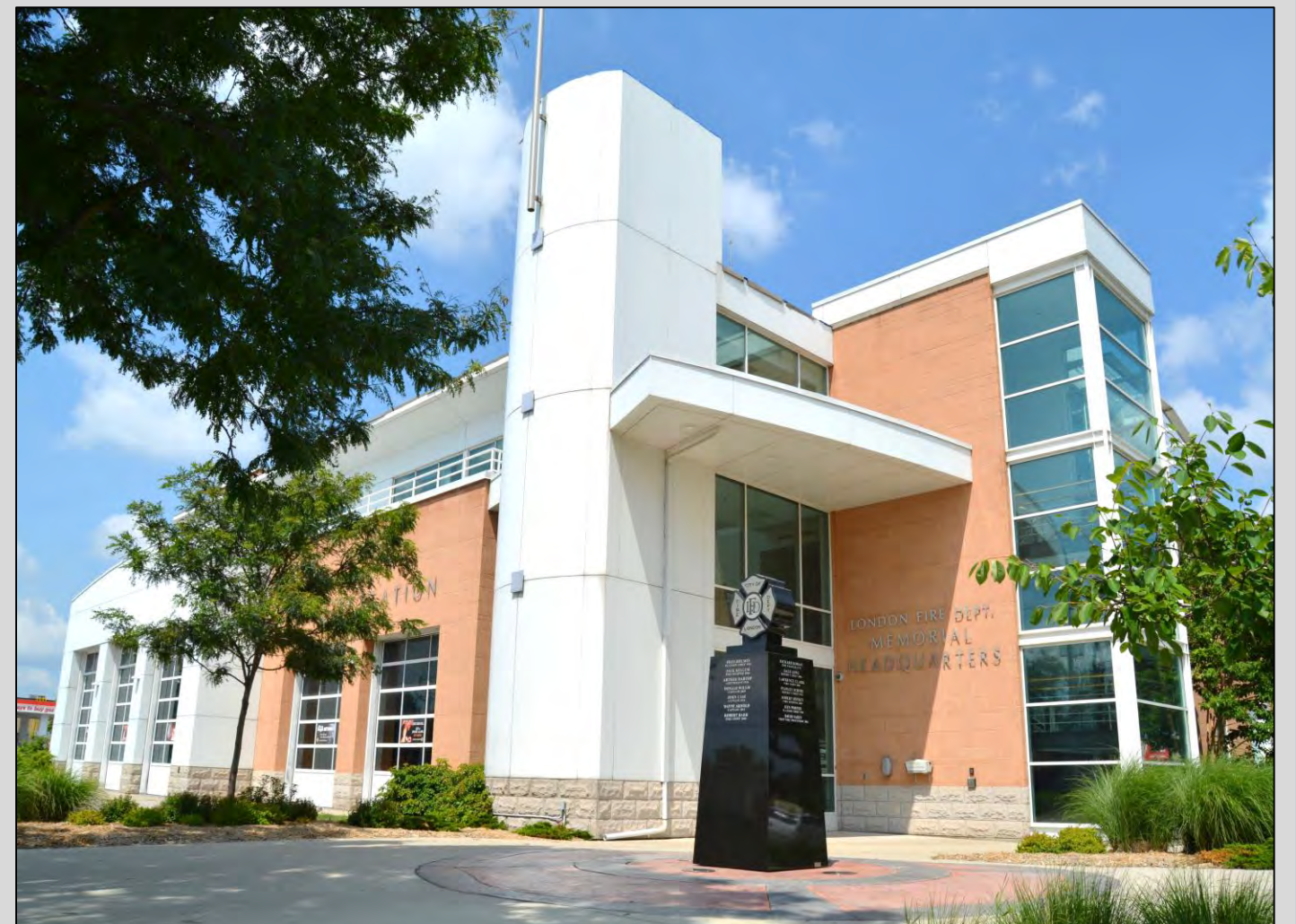
Fire Station # 1 and Head Quarter – Horton St E
