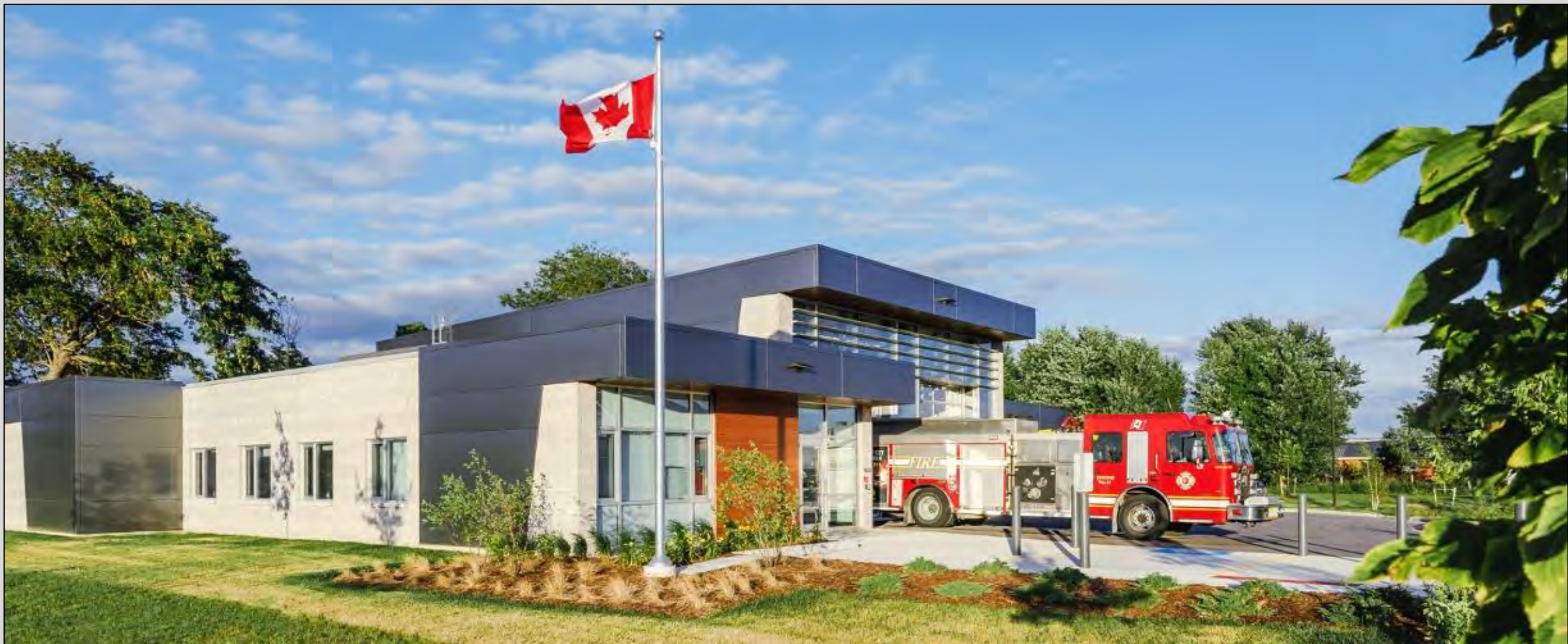
Fire Station # 11 – Savoy street
