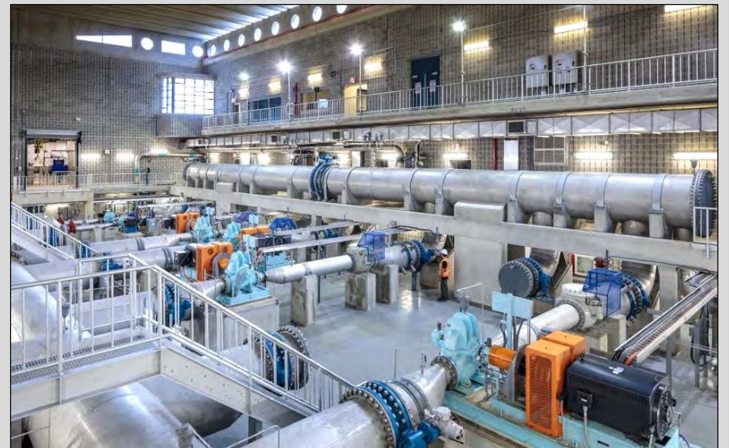
South East Reservoir Interior – Highbury Ave. S
