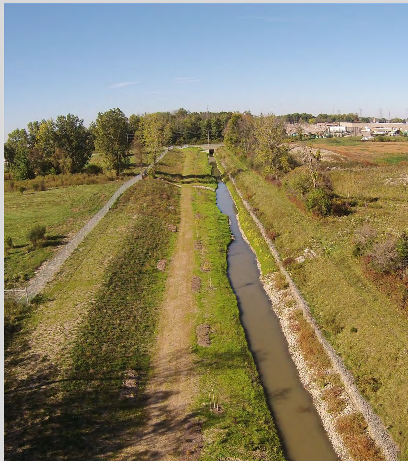
Green Valley Drain
