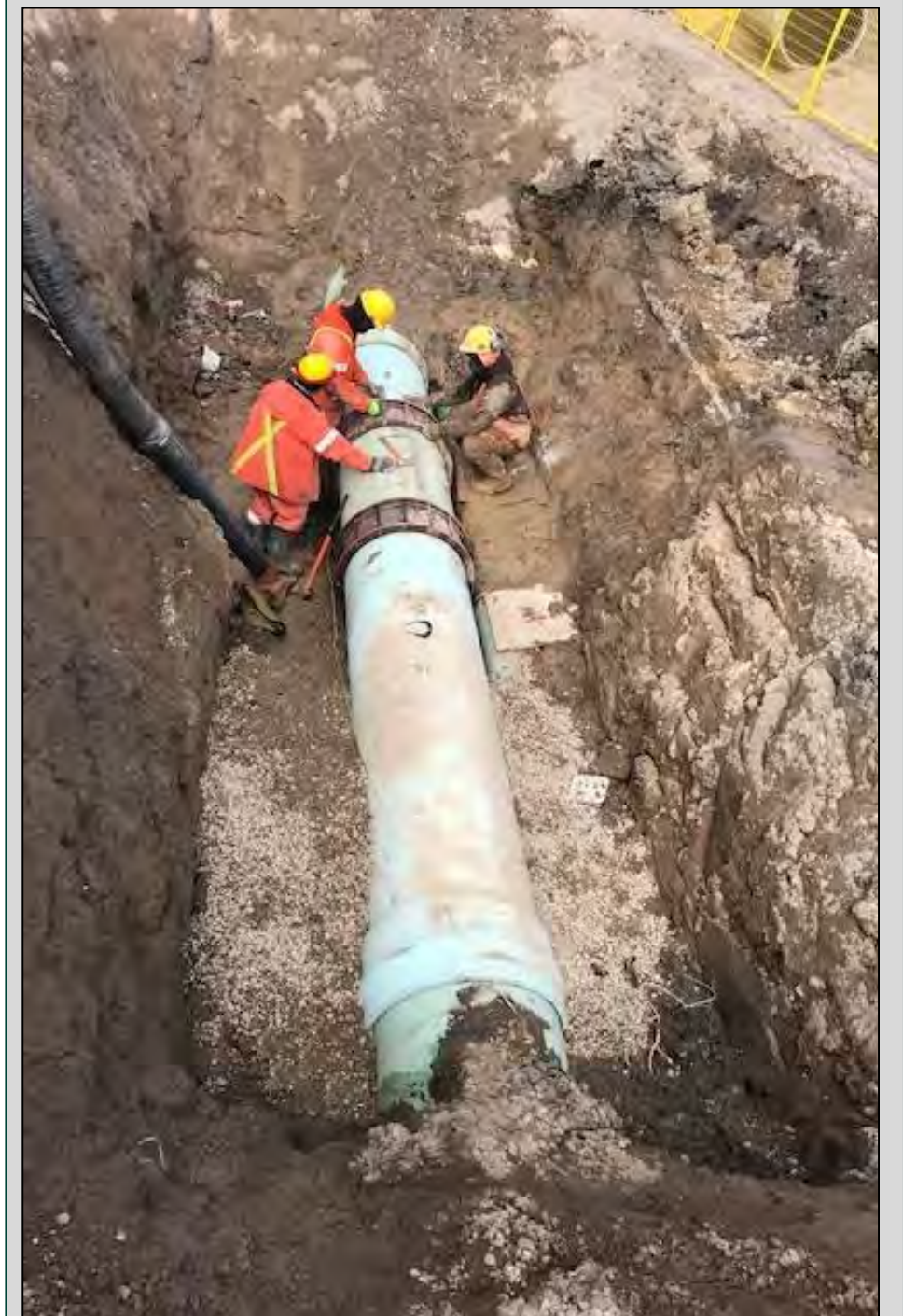
Stormwater Sewer pipes – Conveyance System
