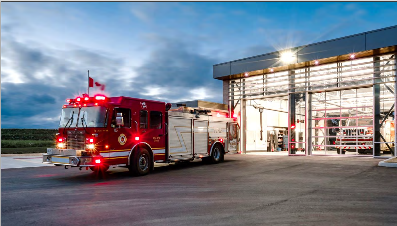
Fire Station # 11 – Savoy Street
