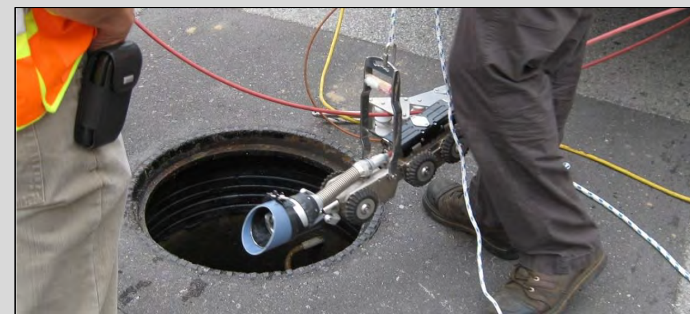
Inspection and Condition Assessment using CCTV
