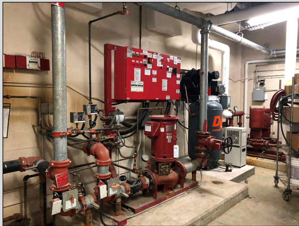
Dearness Home – Boiler and Pump Room
