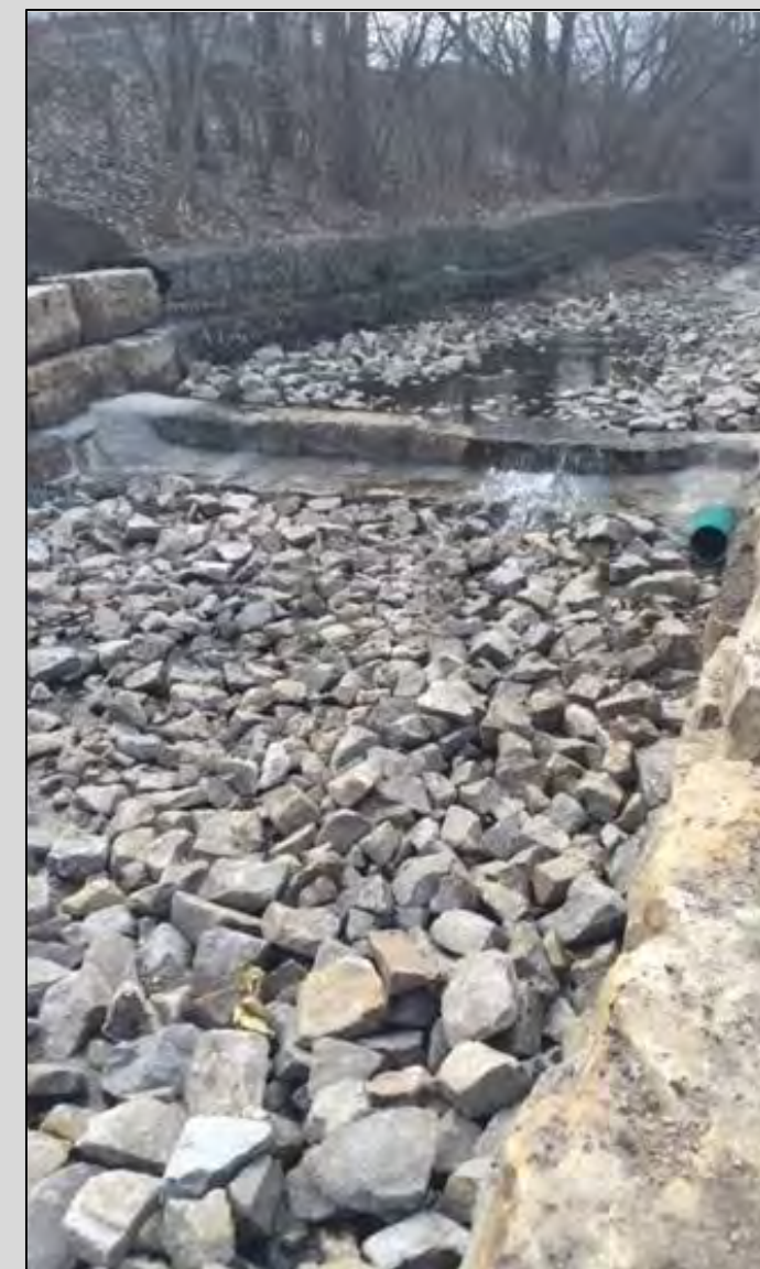
Channel After Restoration work
