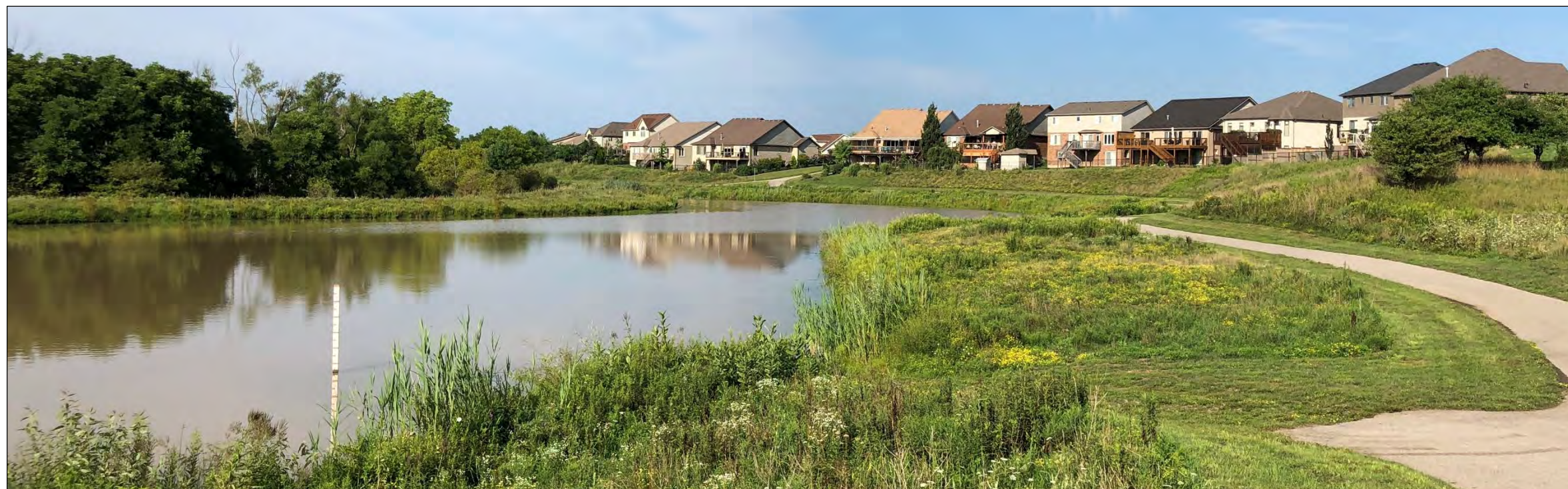
Talbot Village Stormwater Management Facility
