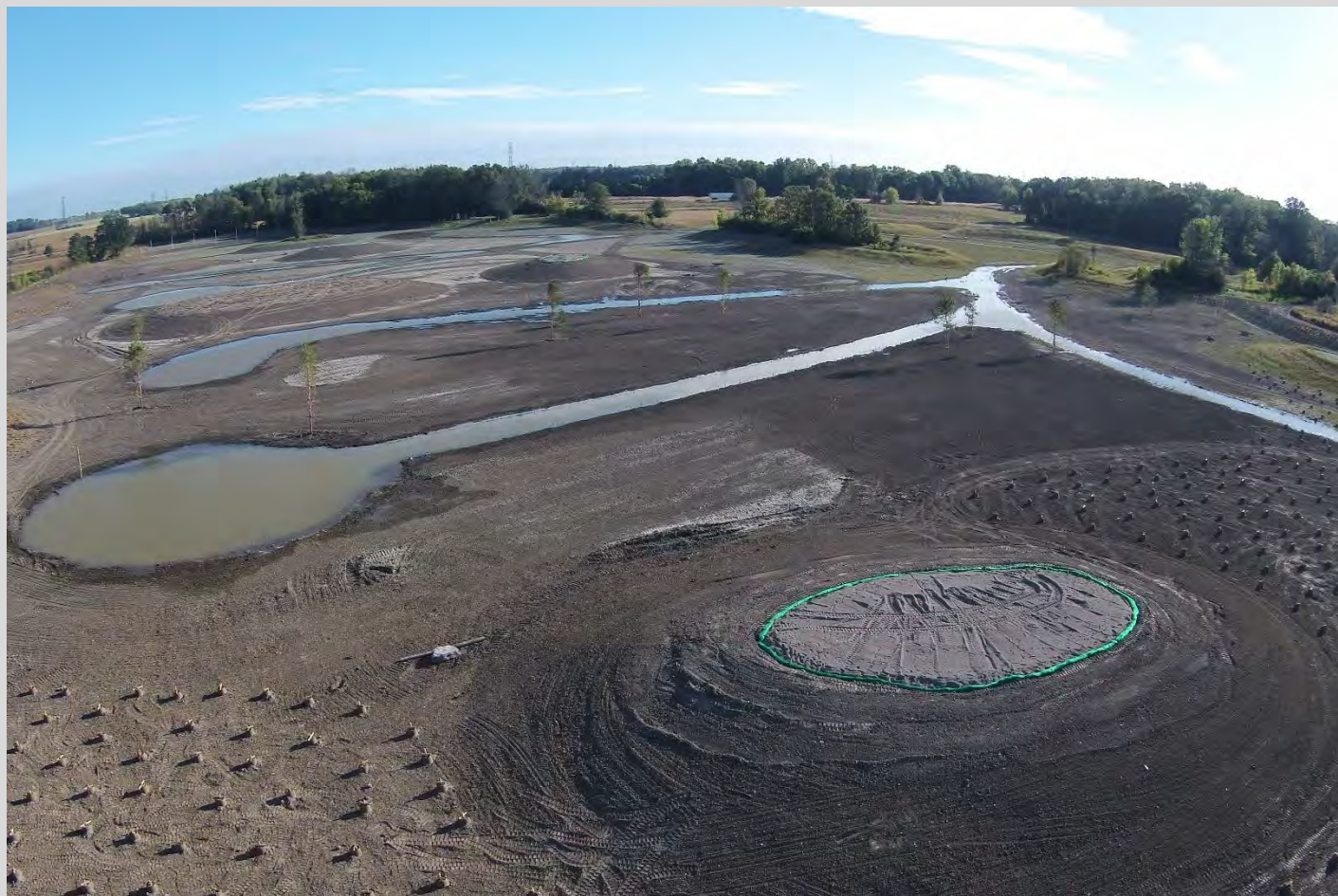
Dingman Erosion Control Facility
