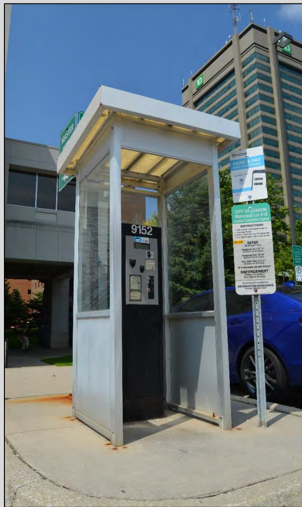
Pay Station Shelter at Parking lot #15
