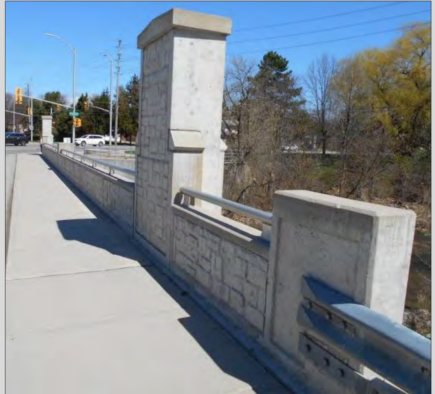
Bridge with Parapet Wall
