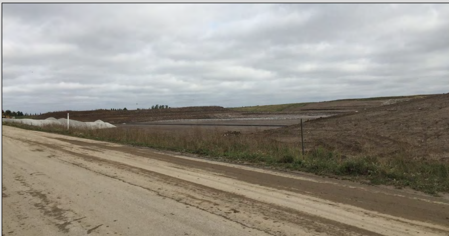
W12A Cell Construction
