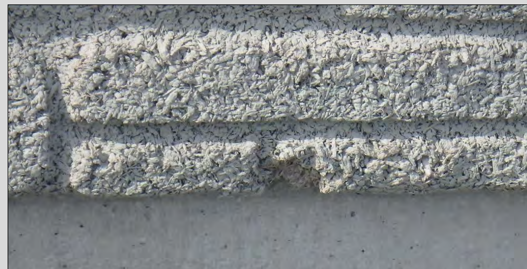
Spalling - Noisewall
