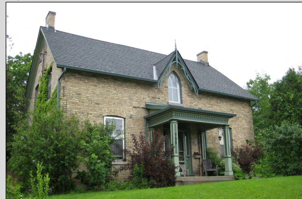
Baty House – Pond Mills Road
