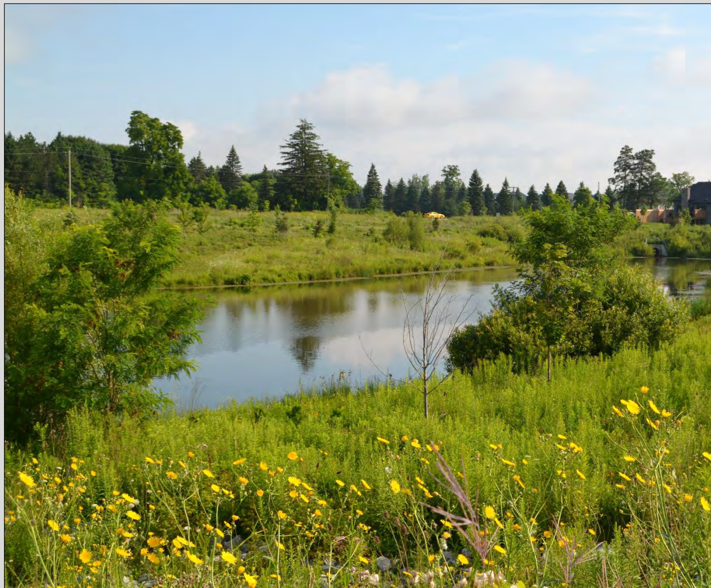
Stormwater Management Facility – Sunningdale Road W.
