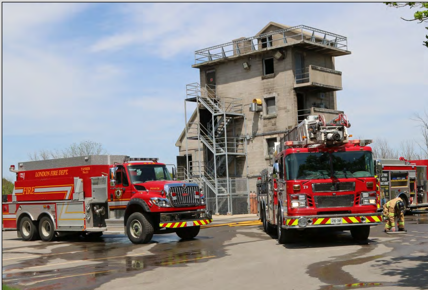
Training Tower – Fire Station # 9
