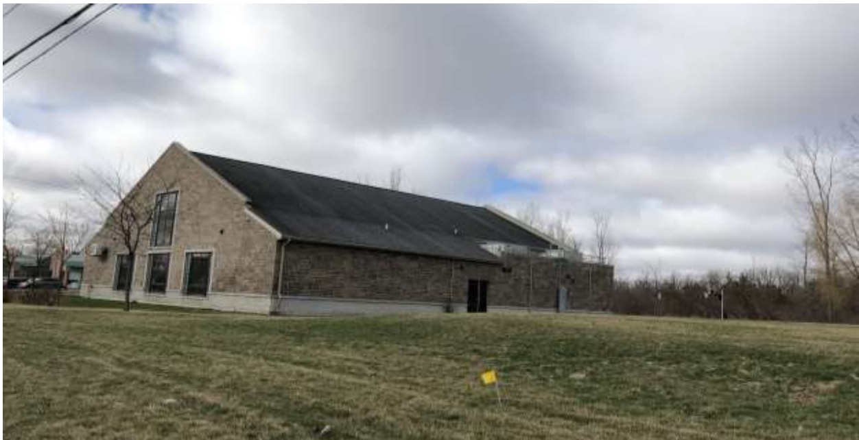
Figure 2: Existing Place of Worship at 85-91 Meg Drive (view from 79 Meg Drive)
