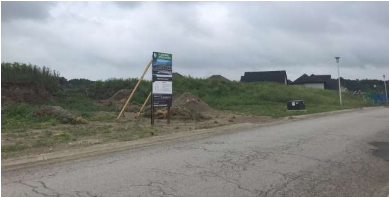
Figure 1: 3086 Tillmann Road – view from Tillmann Road frontage
