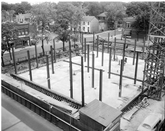
Plate 8: The Lipton Building under construction, 1955 (London Free Press 1955)
