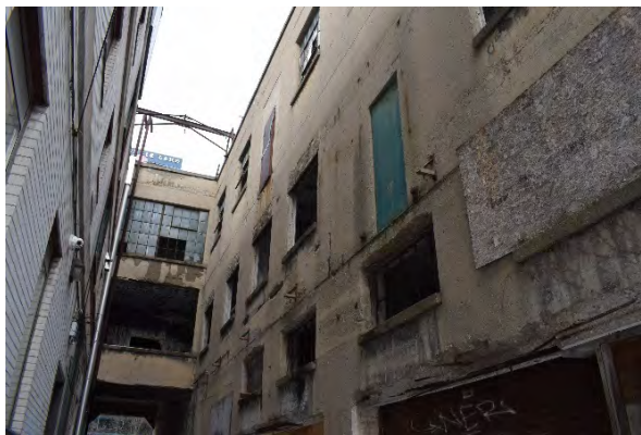
Plate 39: Window openings along alleyway, looking north
