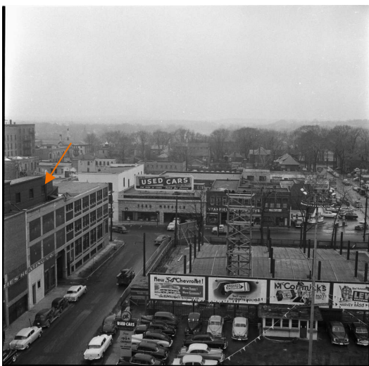
Plate 4: View of front façade of 123 Queens Avenue, 1954 (London Free Press 1954)
