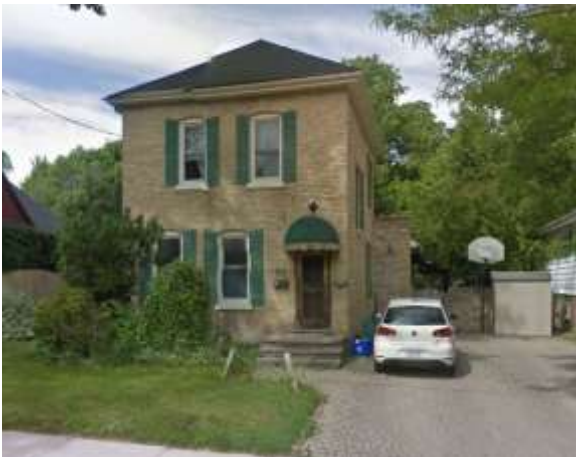
Image 22: 25 Palace Street (1899), East Woodfield Heritage Conservation District (June 2014, courtesy Google).
