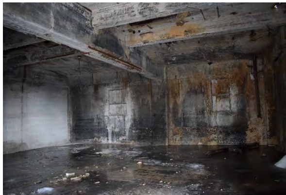
Plate 81: Easterly room, looking north
