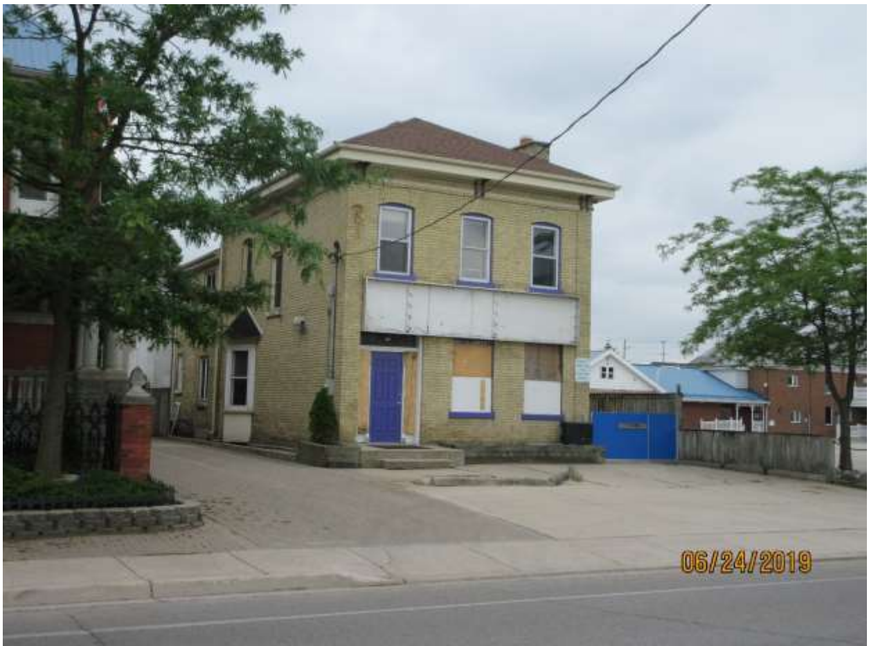
Image 2: Showing the north (main) and east façades of the building at 567 King Street. The adjacent property at 575 King Street (red brick) is shown on the left.
