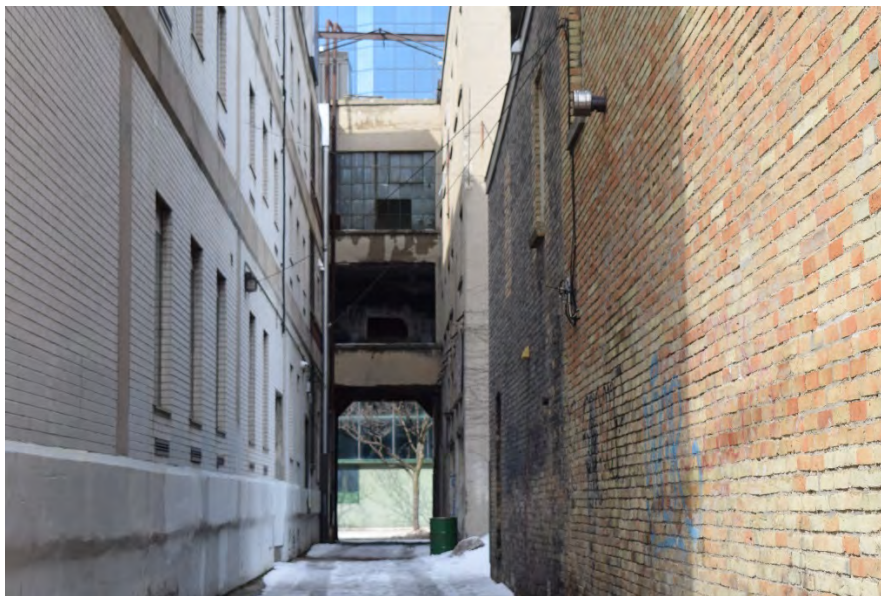
Plate 89: Original exterior of 450 Talbot Street, at left, looking north
