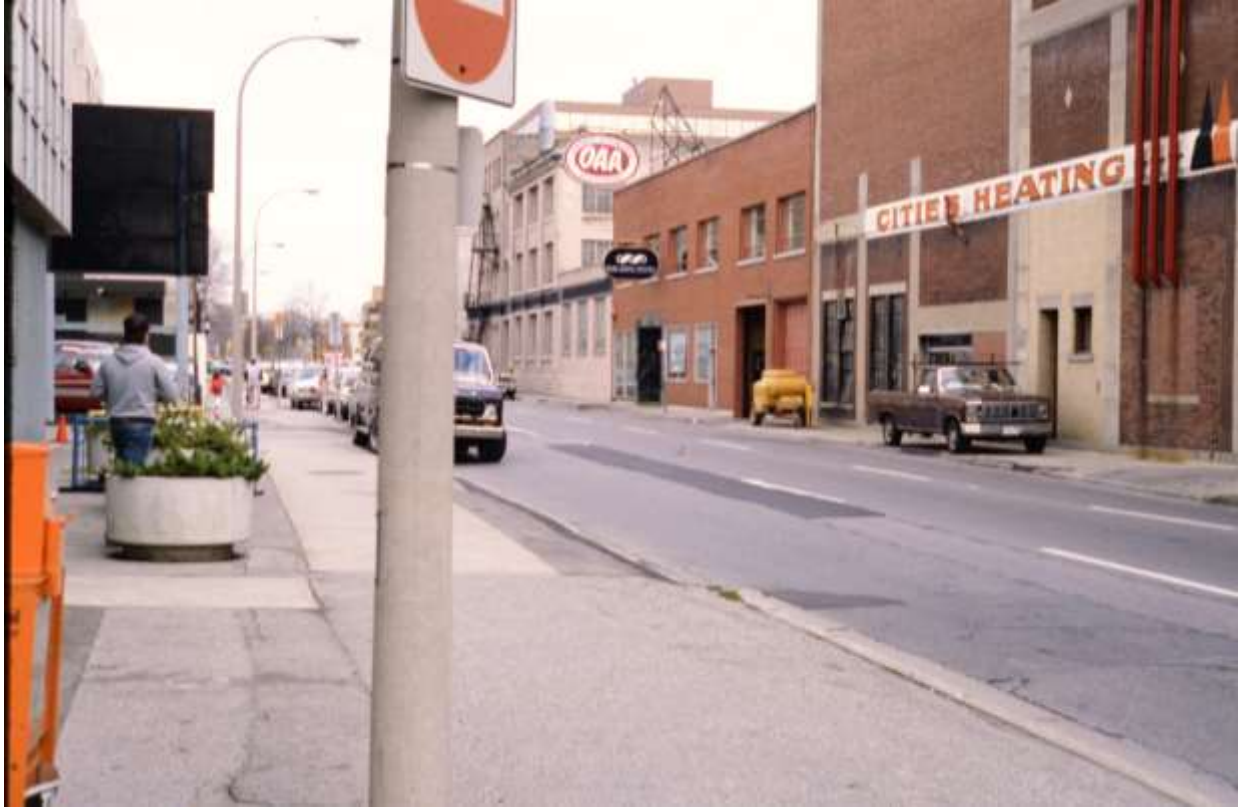
Image 5 – Photo of the south side of Queens Avenue looking east from Talbot Street. Photo taken prior to 1988. The photo shows the bricked in windows at 123 Queens Avenue, but also shows 3 pipes running into the building through the former openings. The exact date of the photo has not been confirmed, but an aerial from 1988 shows the lot located at 134 Carling Street as vacant, which dates the photo to prior 1988 as the photo shows a building on the property at 134 Carling Street. This means that the windows were bricked in at some point between 1955 and 1988.
