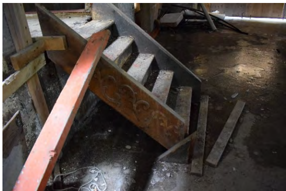
Plate 54: Staircase from Level 2 with scroll detailing
