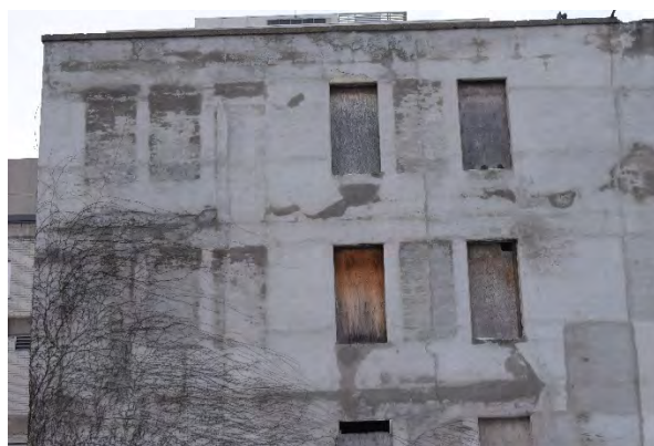
Plate 26: Blind and boarded windows on second and third storey on south half of east façade, looking west
