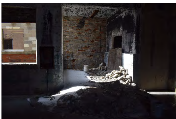
Plate 68: Former connection between 450 Talbot Street and 123 Queens Avenue, looking west
