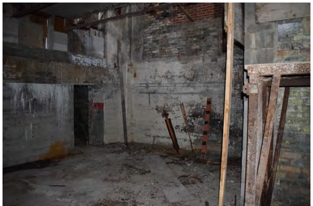
Plate 82: Main basement room, looking north
