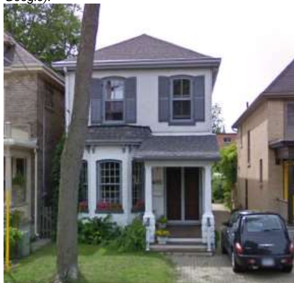
Image 9: 485 Dufferin Avenue (c.1881), East Woodfield Heritage Conservation District (July 2009, courtesy Google).
