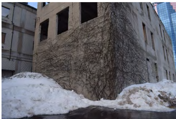
Plate 33: First storey of south façade, looking north
