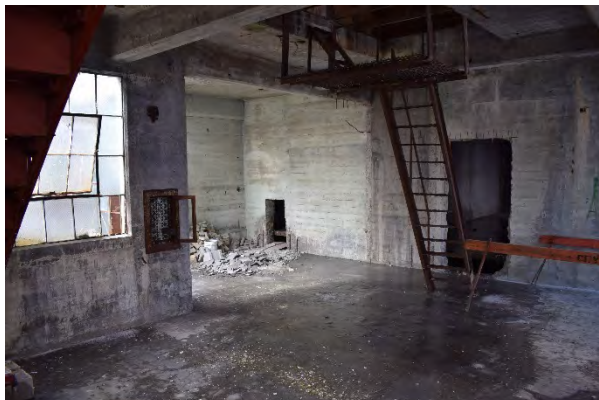
Plate 73: Metal staircase, looking north
