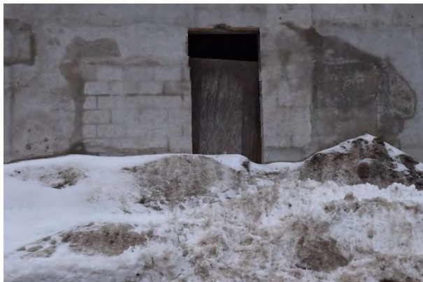
Plate 29: Concrete block wall on part of east façade, looking west
