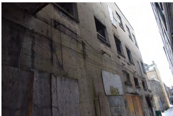
Plate 40: Window openings along alleyway, looking south
