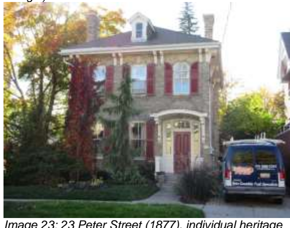
Image 23: 23 Peter Street (1877), individual heritage designated property (October 22, 2015).
