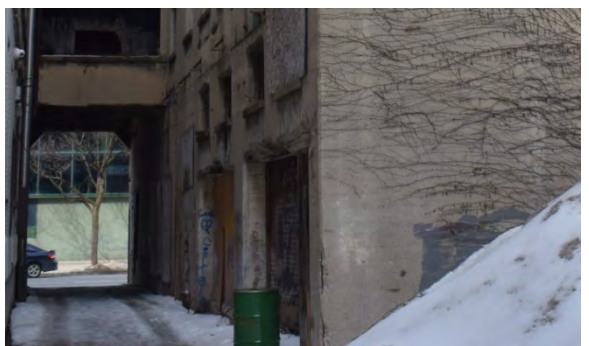
Plate 41: First storey entrances on west façade, looking north
