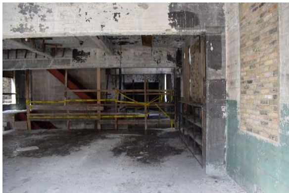
Plate 65: Window openings bricked with buff brick
