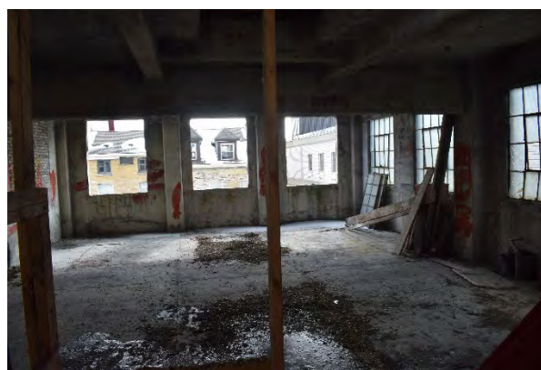
Plate 71: South and west walls, looking south
