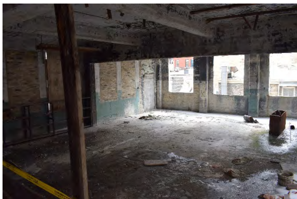
Plate 62: Southeast corner of south section, looking south
