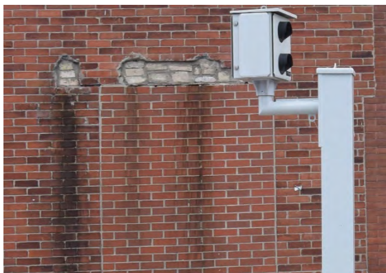
Plate 23: Missing red brick cladding, exposing buff brick
