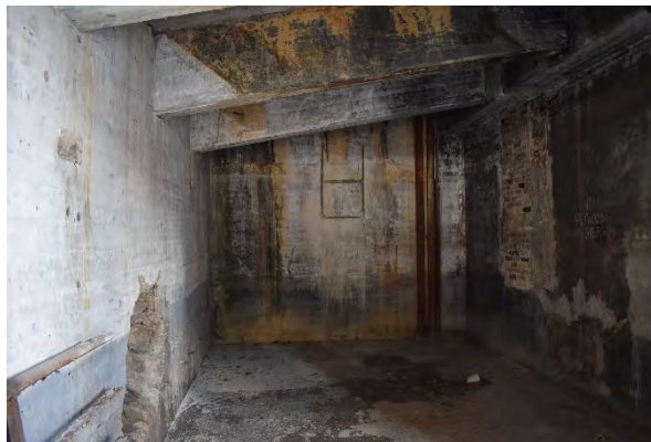
Plate 79: Most westerly room, looking north
