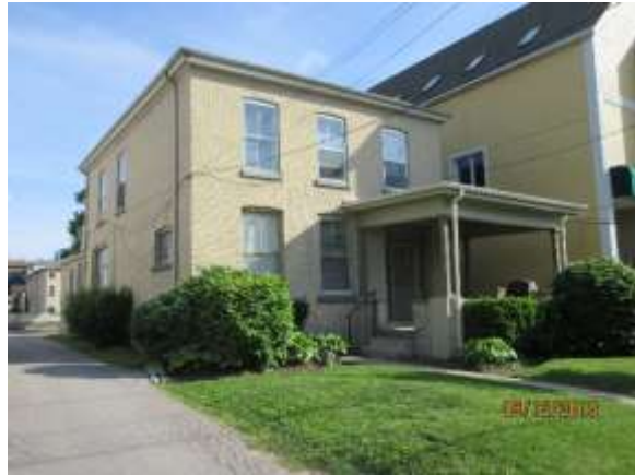
Image 5: 185 Central Avenue (1881), heritage listed property.
