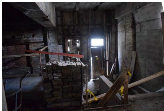
Plate 51: Level 1 of first storey showing entrance
