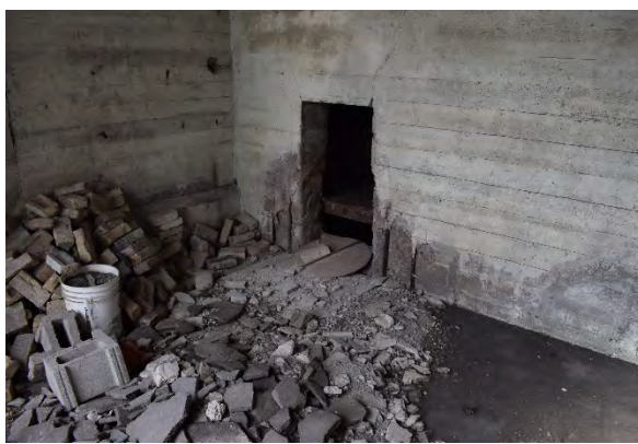
Plate 77: Opening in concrete wall adjacent to metal doors, looking north
