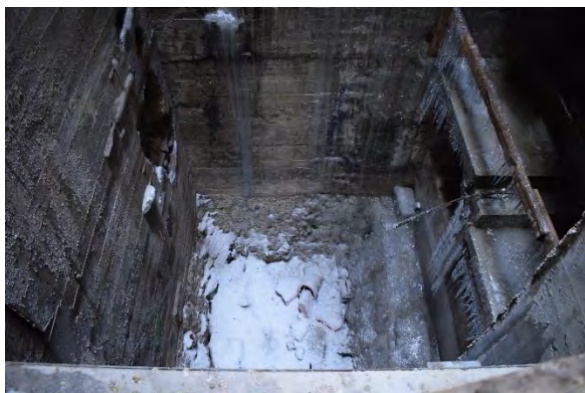
Plate 48: Open area spanning basement to third floor, viewed from first floor
