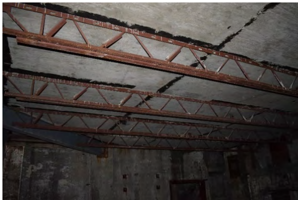
Plate 83: Metal beams in basement and plywood ceiling
