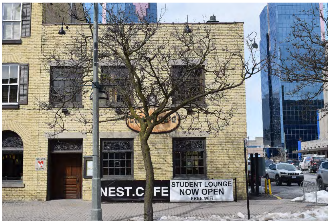
Plate 91: 126 Carling Street, looking north
