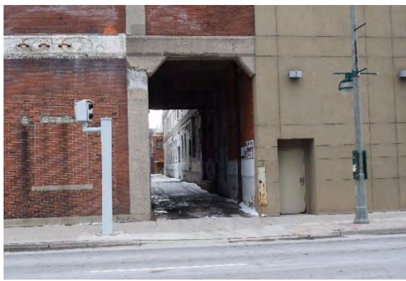
Plate 24: Laneway, looking south
