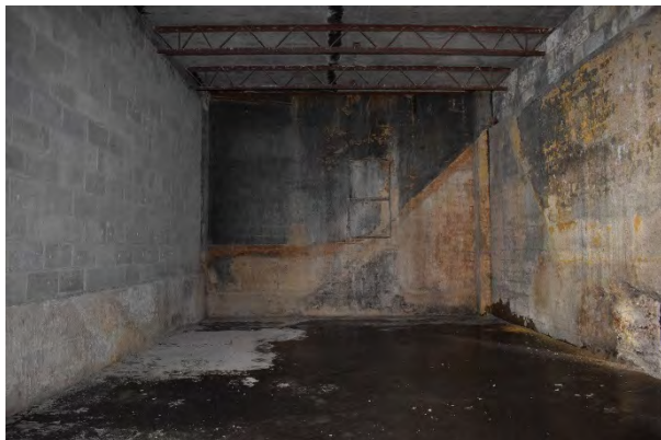
Plate 80: Middle room, looking north
