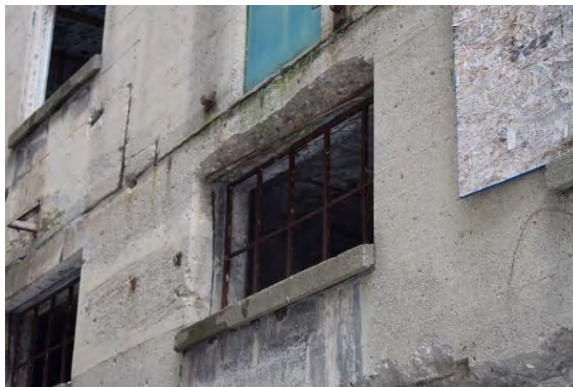
Plate 43: Windows with bars on west façade, looking east
