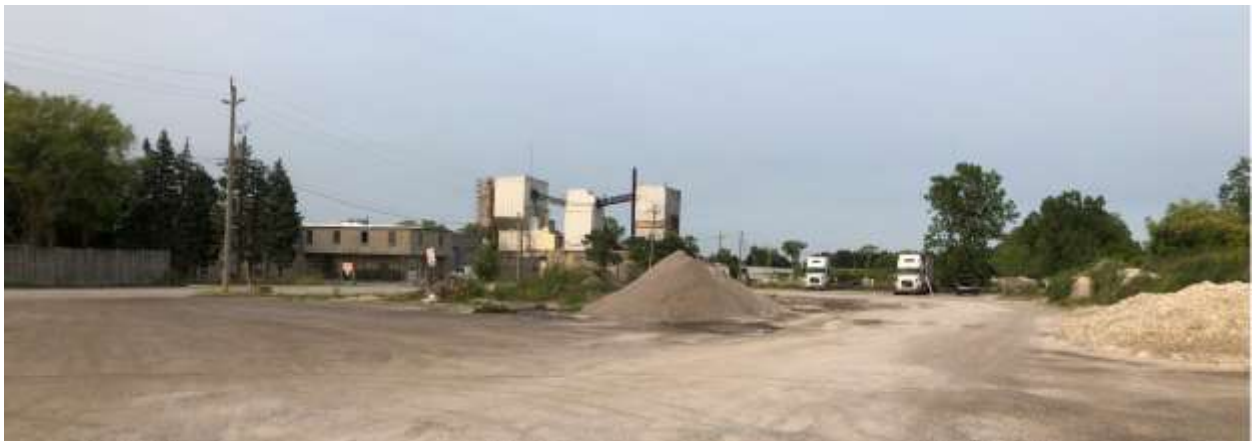
Figure 3 – View of Concrete Batching Plant from 3354 Wonderland Road South
