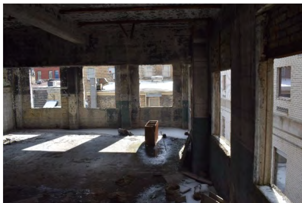
Plate 63: Southwest corner of south section, looking south
