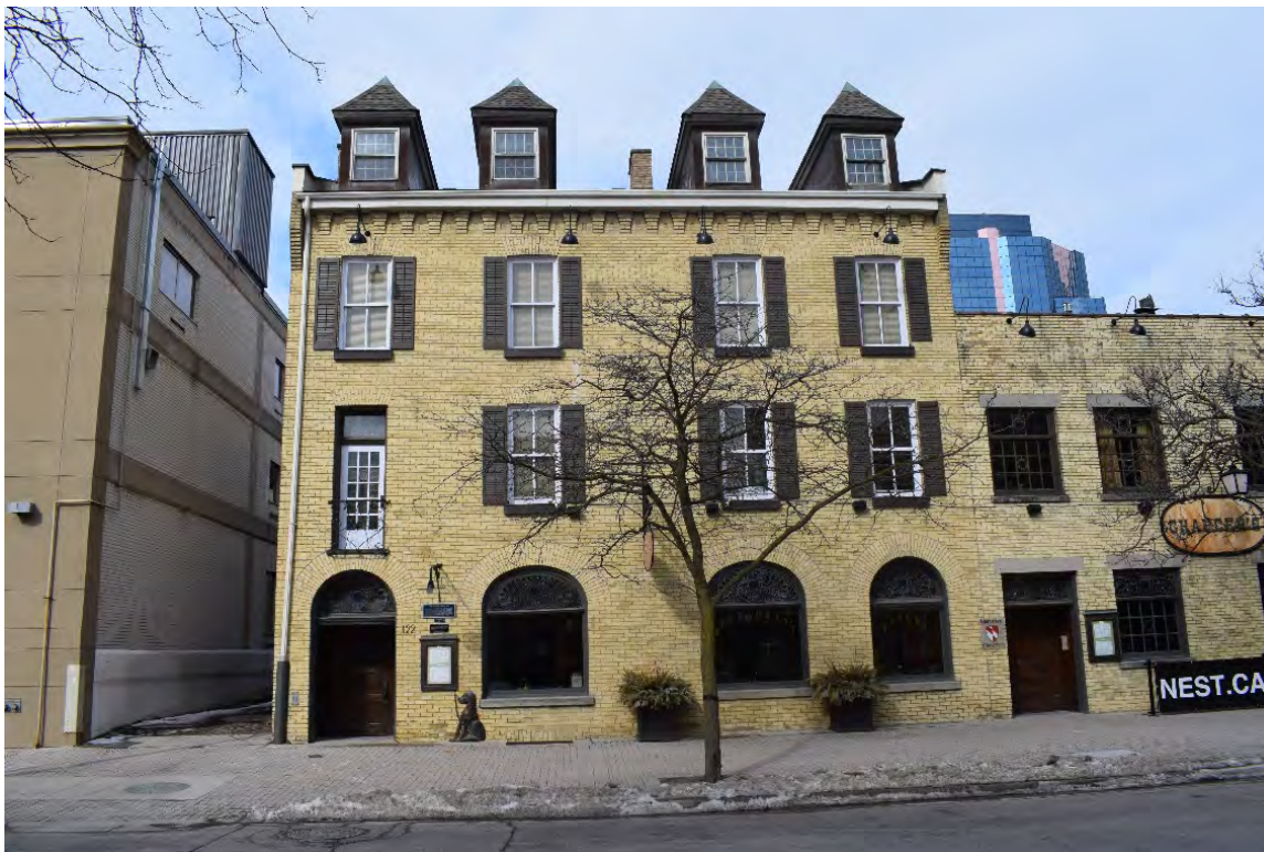
Plate 90: 122 Carling Street, looking north
