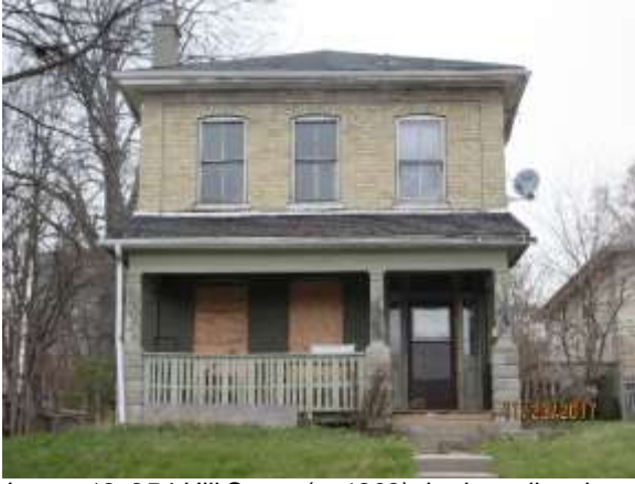
Image 18: 254 Hill Street (p. 1868), heritage listed property (November 23, 2017).
