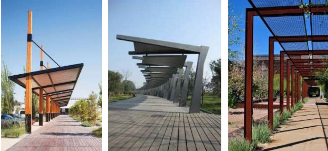
Figure 11 – Examples of Built Form Canopy Structures
