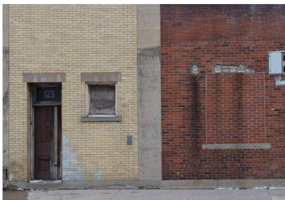
Plate 22: Entrance door, transom, window, and blind window, looking south
