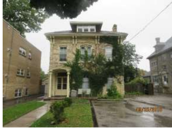
Image 43: 480 William Street (c.1875), East Woodfield Heritage Conservation District (September 25, 2018).
