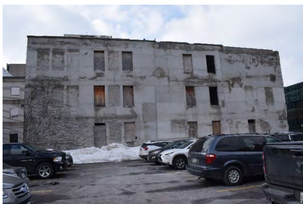
Plate 25: East façade, looking west
