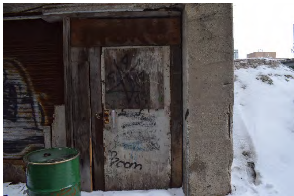
Plate 42: Doorway at rear of west façade, looking east
