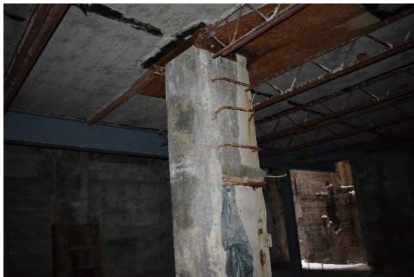
Plate 84: Concrete column and ladder rungs, looking east
