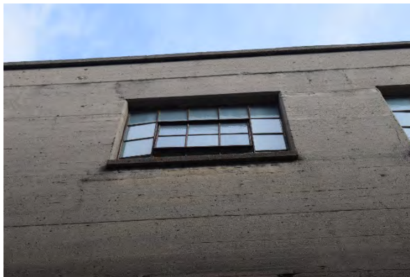
Plate 37: Opaque glass window on west façade, looking east
