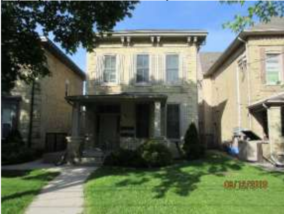
Image 36: 640 Talbot Street (c.1874), heritage listed property.
