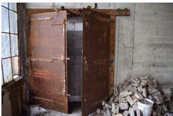
Plate 76: Metal doors, looking west
