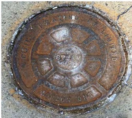
Plate 13: CHC manhole cover, located outside 171 Queens Avenue
