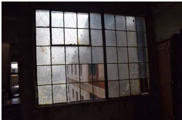
Plate 78: Window in corridor connecting 123 Queens Avenue and 450 Talbot Street, looking south
