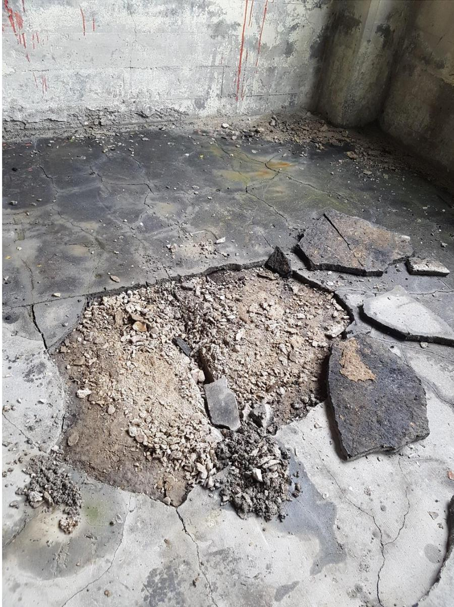
Photograph No. 2 – Asphalt Layer Overlying the Poor Concrete Floor Slab
