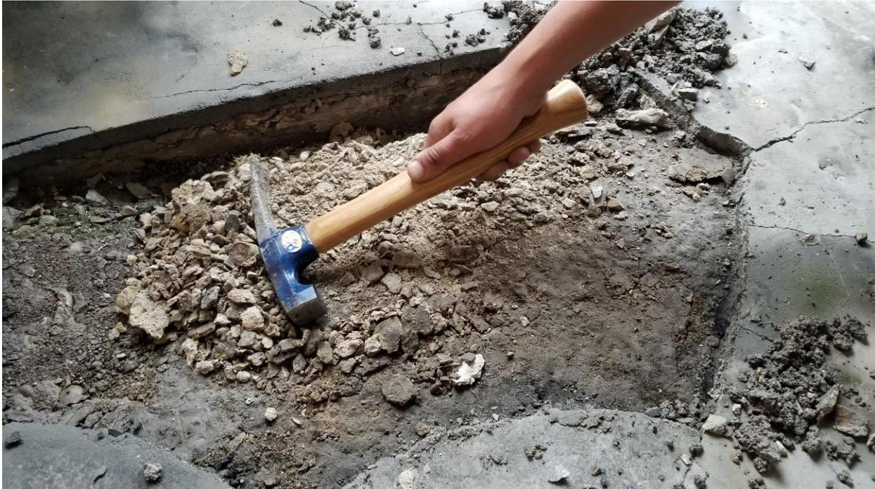
Photograph No. 4 – Broken Pieces/Crumble of Concrete Floor Showing Unsuitable Coring Conditions
