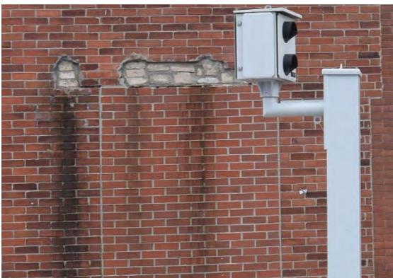
**Plate 23: Missing red brick cladding, exposing buff brick**
