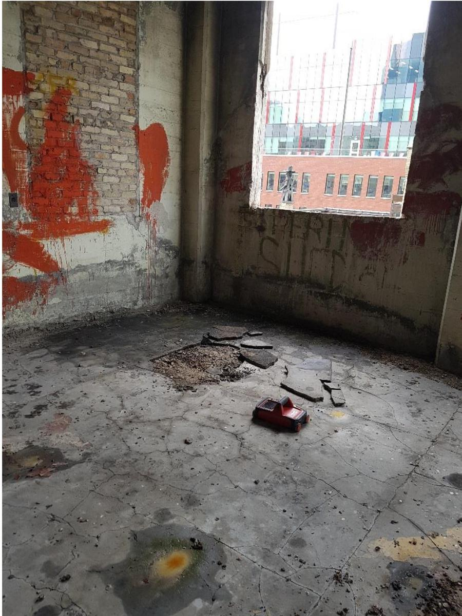
Photograph No. 1 – Severe Concrete Floor and Wall Cracks
