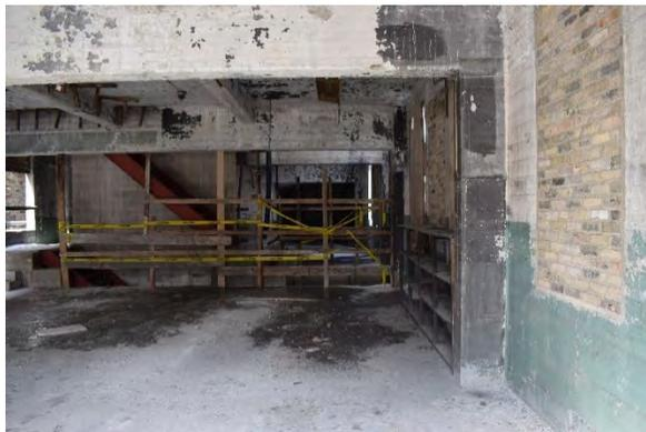
**Plate 65: Window openings bricked with buff brick**
