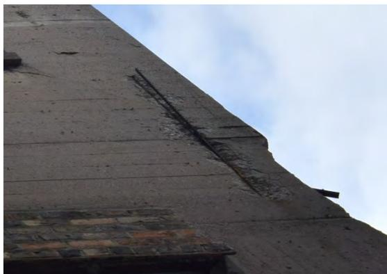
Plate 35: Exposed rebar on west façade, looking east
