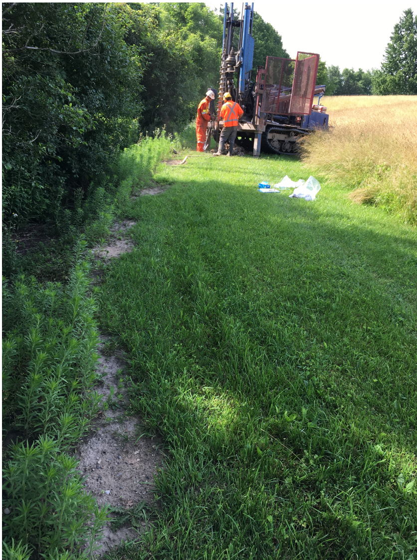
Photo 1 – Tableland and slope crest at Borehole BH1.
