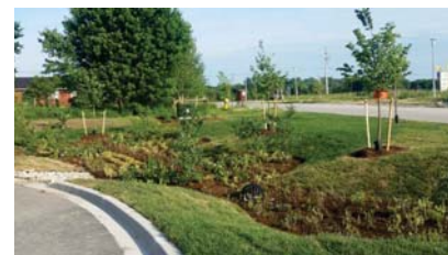
Firehall 11, London Ontario, Constructed 2017
