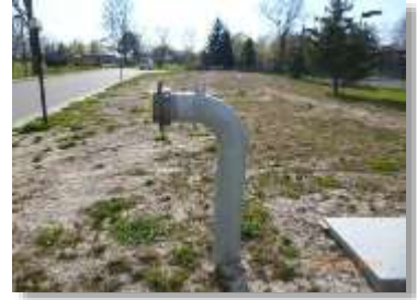
Figure 1: Drafting Port Side View - 90 Deg Elbow
