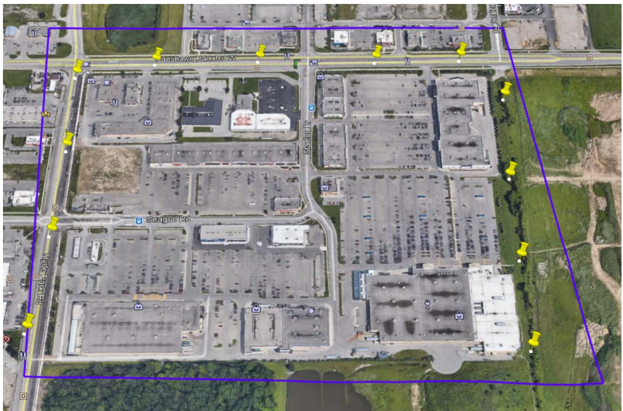
Figure 3: North London pilot area small cell locations.
