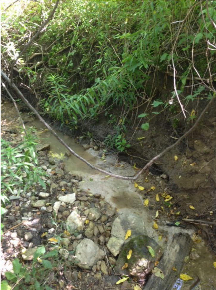
Photo 2 – Drainage Creek Base
