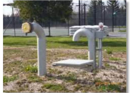
Figure 5: Underground Tank with Vent and Access
