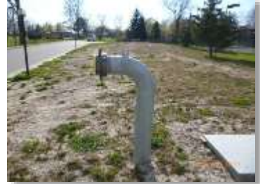
Figure 1: Drafting Port Side View - 90 Deg Elbow
