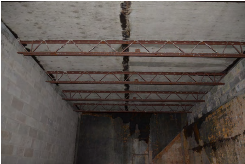
Photo No 02: Added Hambro Floor System
