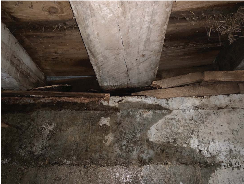
Figure 7.0 - Photo of Damaged Perimeter Sill-plate
