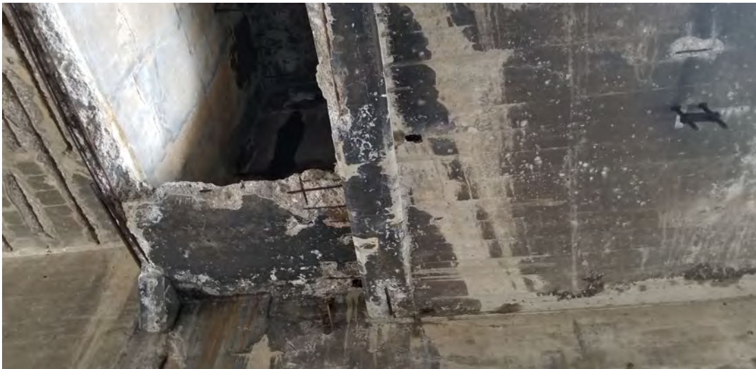
Photo No 05: Delaminated Concrete Beam at Link
