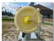
(4) the aforementioned threaded connection must be perpendicular to the side of the fire truck when positioned (see Figure 4).
