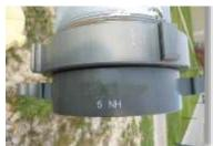
(3) to prevent debris being thrown into the drafting port, the 5 inch (127mm)NH female swivel shall be closed with a 5 inch(127 mm) NH thread male cap or plug (see Figure 3); and
