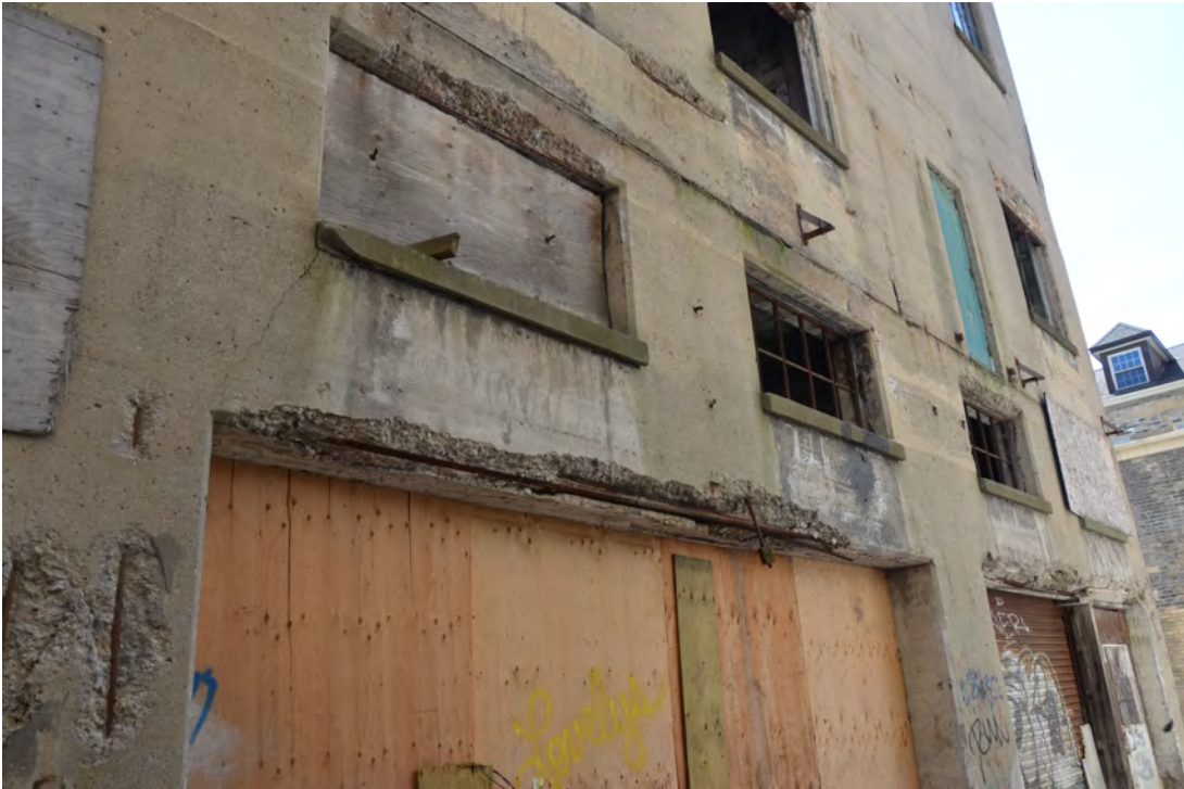
Photo No 04: Delaminated Concrete Beams
