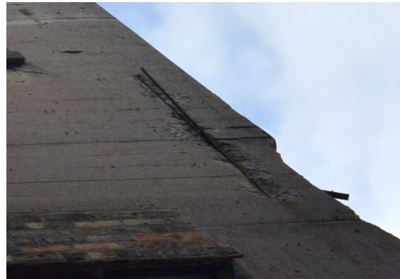
Plate 35: Exposed rebar on west façade, looking east
