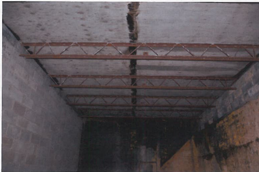
Photo No 02: Added Hambro Floor System
