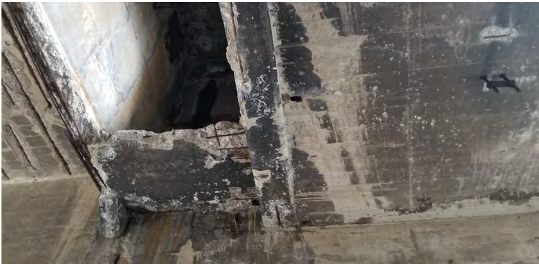
Photo No 05: Delaminated Concrete Beam at Link
