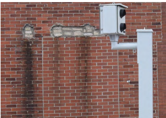
Plate 23: Missing red brick cladding, exposing buff brick
