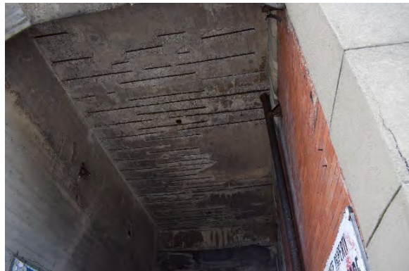
Plate 45: Exposed rebar, looking south
