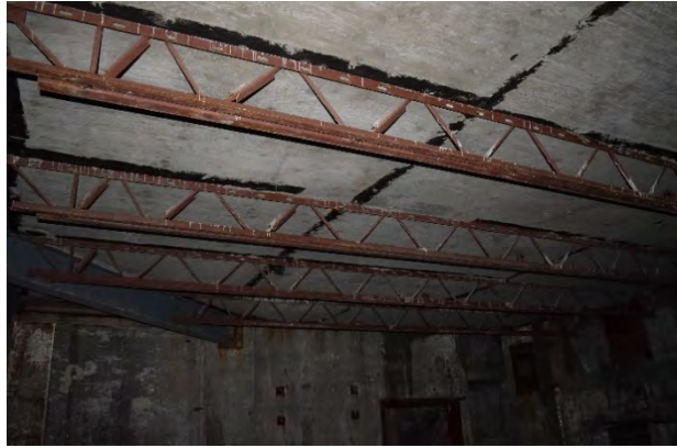
Plate 83: Metal beams in basement and plywood ceiling
