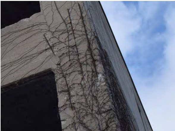
Plate 31: Exposed rebar, looking north
