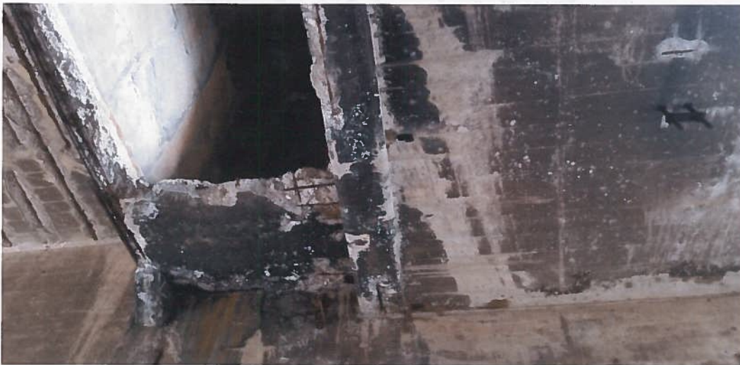
Photo No 05: Delaminated Concrete Beam at Link
