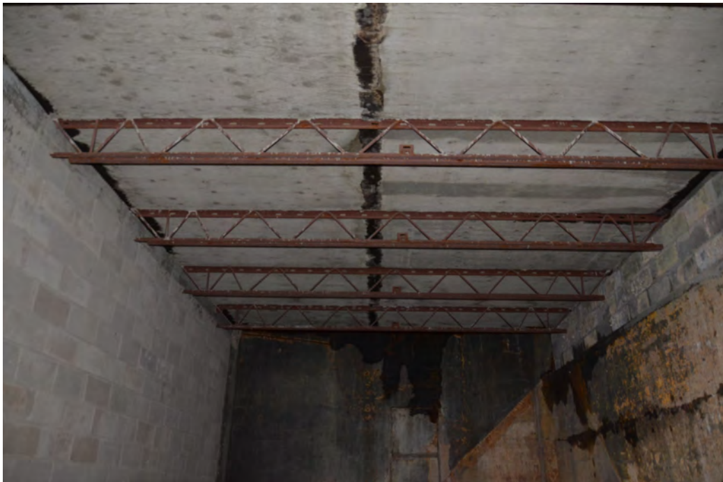
Photo No 02: Added Hambro Floor System
