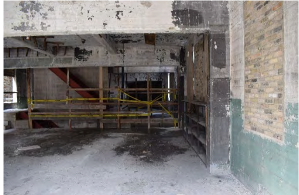
Plate 65: Window openings bricked with buff brick
