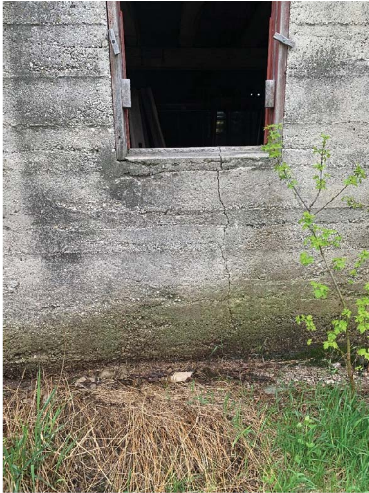
Figure 9.0 – Photo of Cracked Existing Foundation Wall
