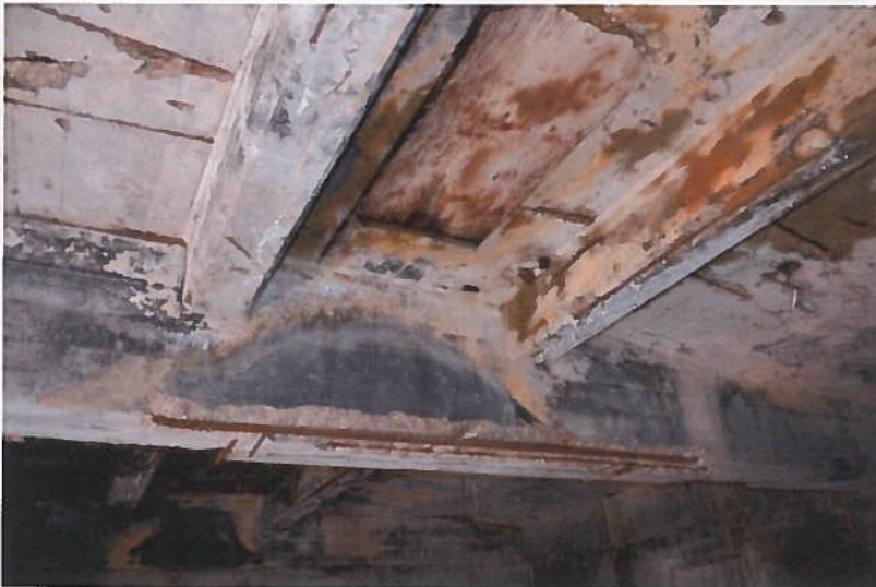
Photo No 08: Typical Interior Upper Beam
