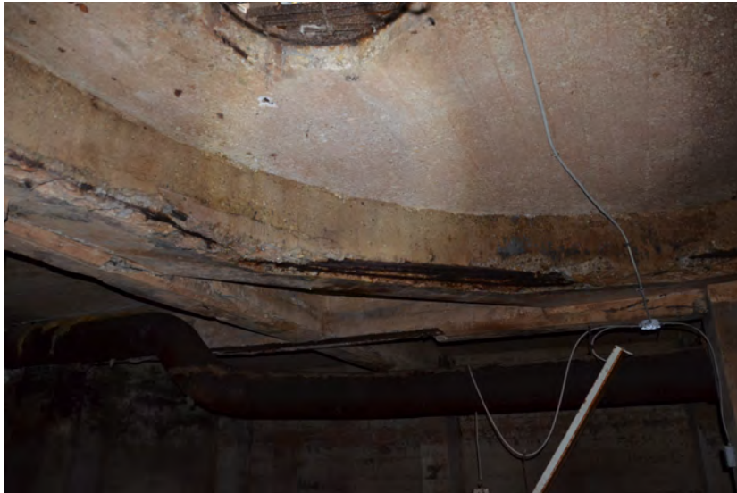
Photo No 09: Interior Basement Beams (south end)
