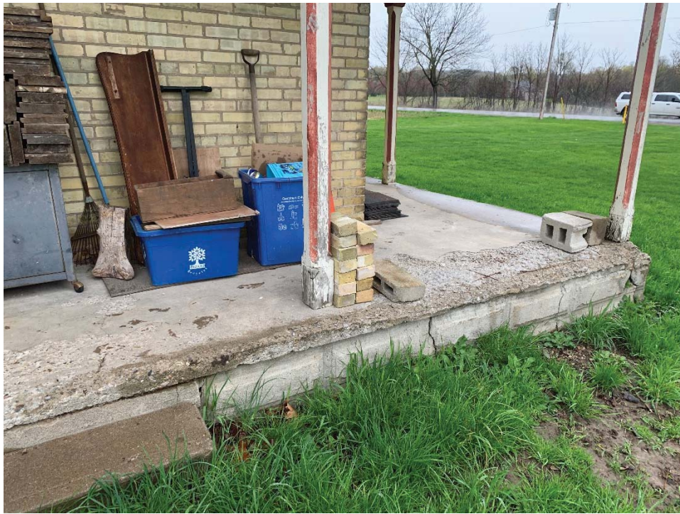
Figure 1.0 – Photo of Existing Porch Slab and Foundation Structure
