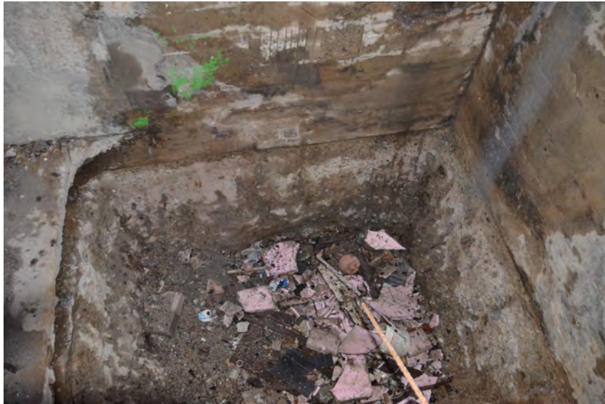
Photo No 07: Excavation of the Interior (east Side)
