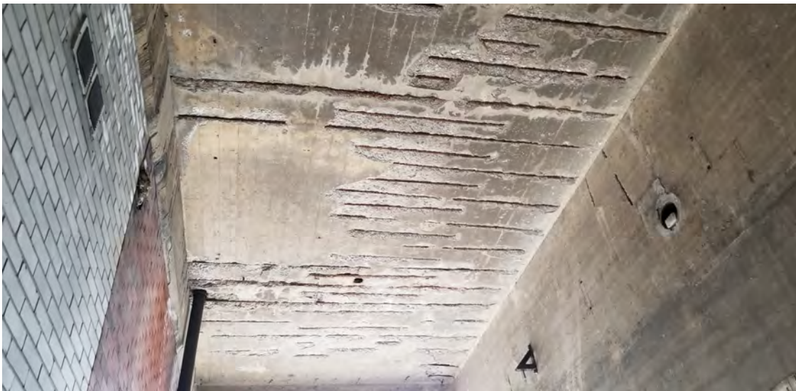
Photo No 06: Suspended Link Slab (Exterior)
