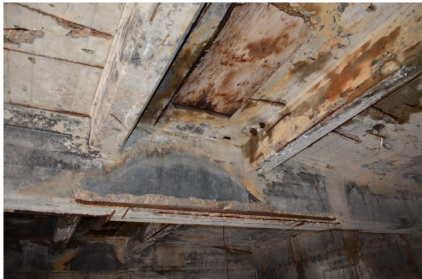
Photo No 08: Typical Interior Upper Beam
