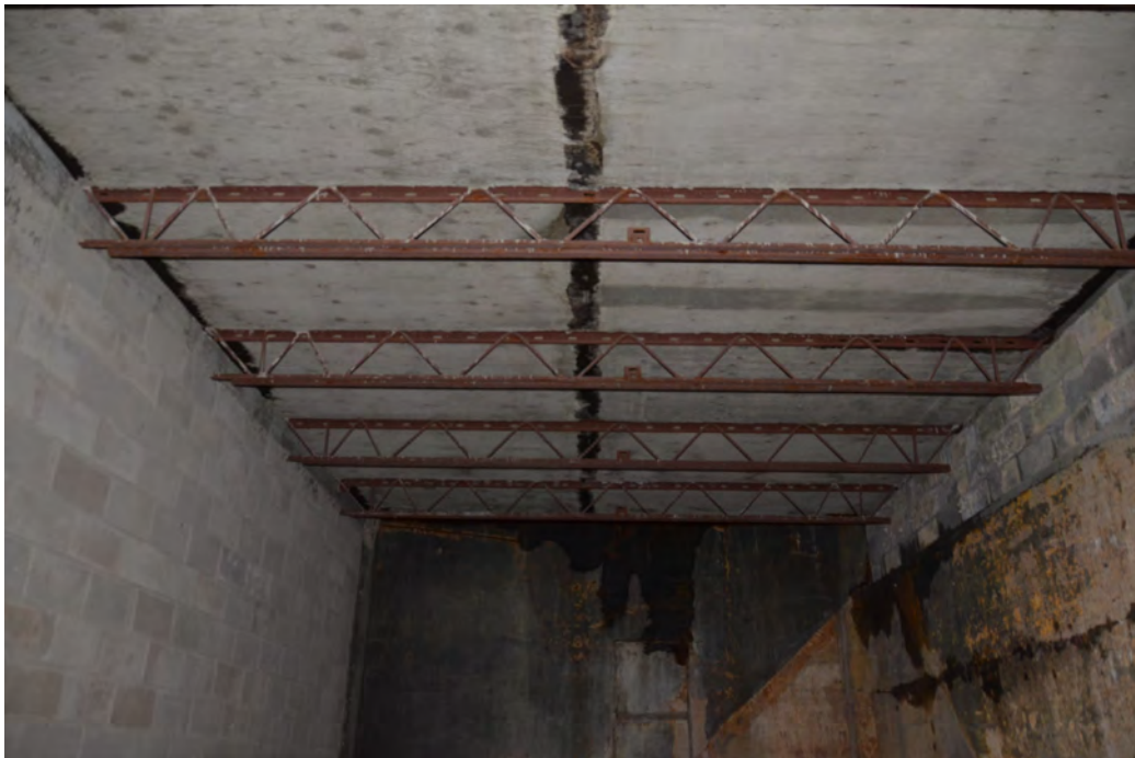
Photo No 02: Added Hambro Floor System
