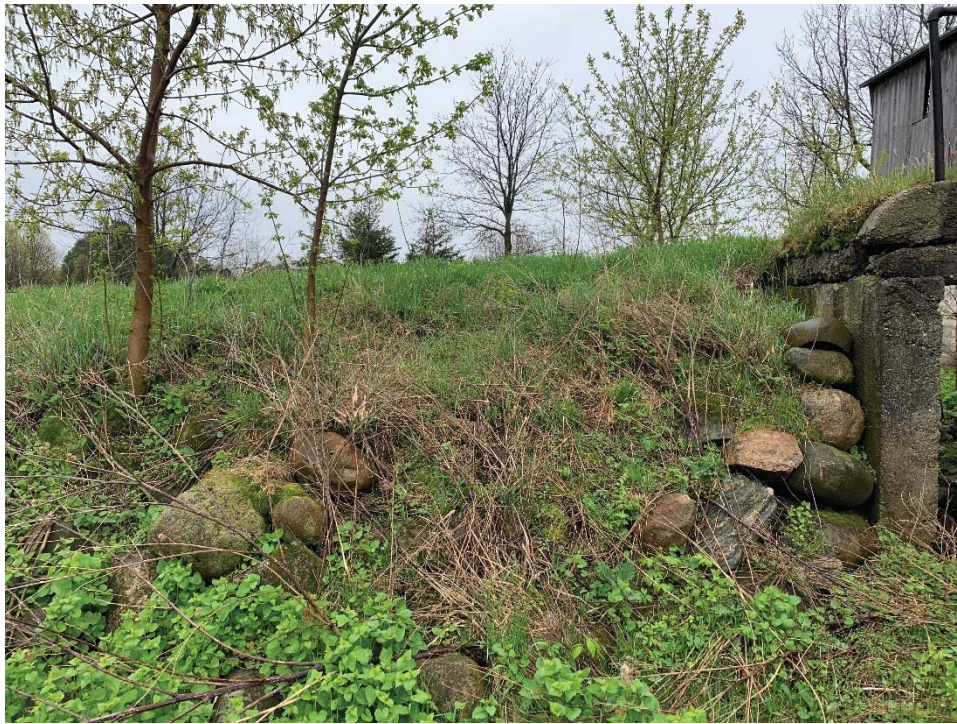
Figure 1.0 – Photo of Existing Approach Ramp to Barn (Bank Barn)
