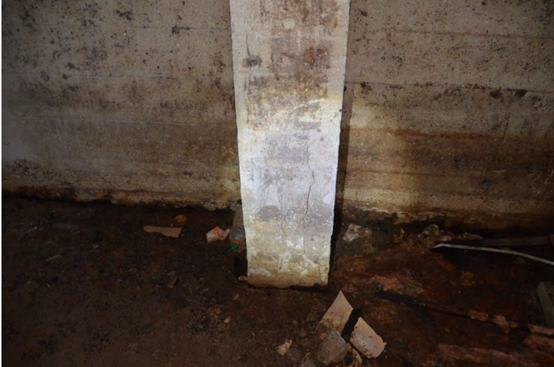
Photo No 03: Concrete Foundation Walls
