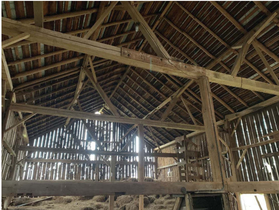
Figure 6.0 - Photo of Existing Barn (Bank Barn) Interior Post and Beam Structure
