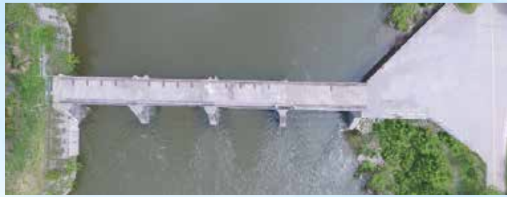
Exhibit 1. Springbank Dam Partial Dam Removal
