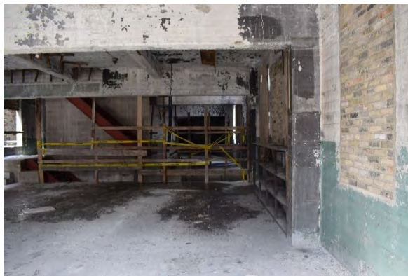
Plate 65: Window openings bricked with buff brick
