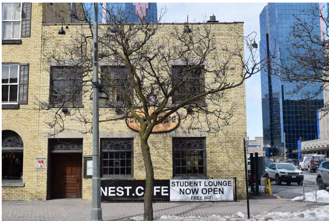
Plate 91: 126 Carling Street, looking north
