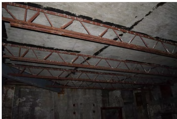
Plate 83: Metal beams in basement and plywood ceiling
