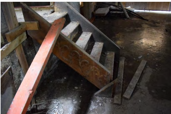
Plate 54: Staircase from Level 2 with scroll detailing
