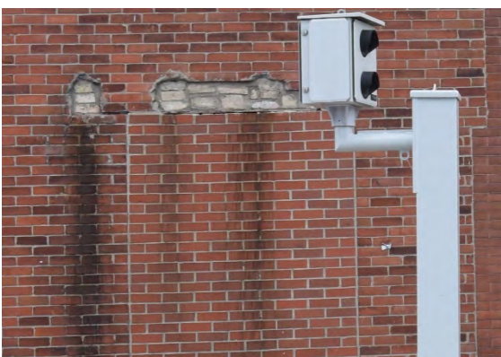
Plate 23: Missing red brick cladding, exposing buff brick
