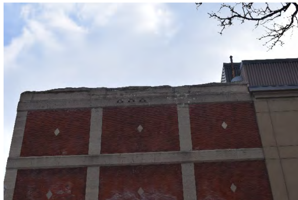
Plate 20: Second and third storey concrete banding and concrete diamonds topped by a concrete parapet, looking south
