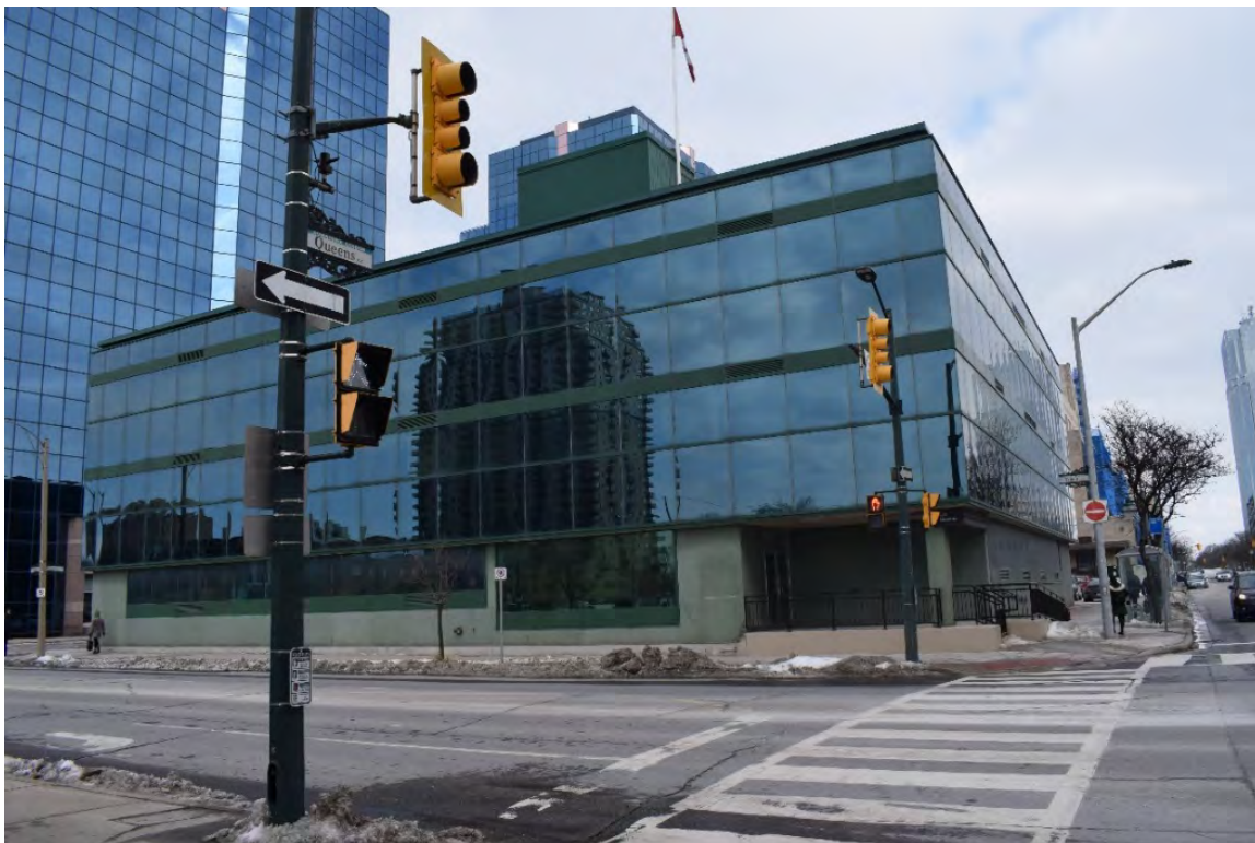
Plate 92: 120 Queens Avenue, looking east
