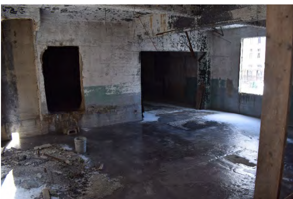
Plate 66: Second storey north section, looking north
