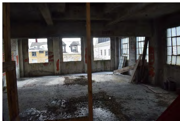
Plate 71: South and west walls, looking south
