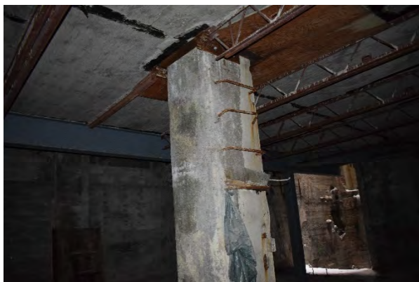
Plate 84: Concrete column and ladder rungs, looking east
