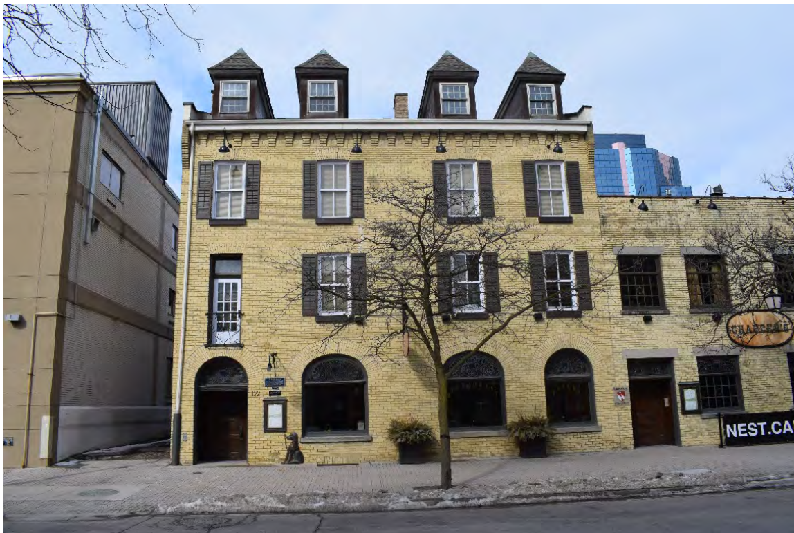
Plate 90: 122 Carling Street, looking north
