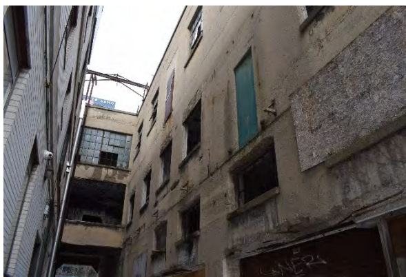
Plate 39: Window openings along alleyway, looking north
