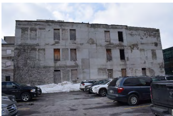
Plate 25: East façade, looking west
