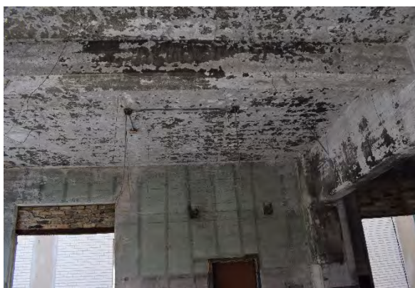
Plate 69: Wiring for light fixtures
