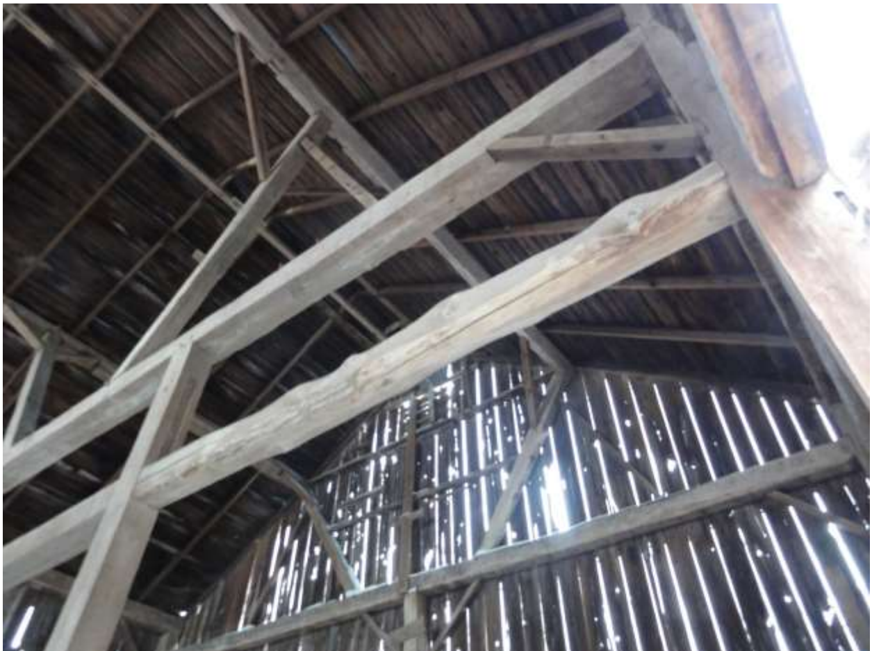
Image 6: View of barn interior illustrating exterior bent, west face (2019-02-14).
