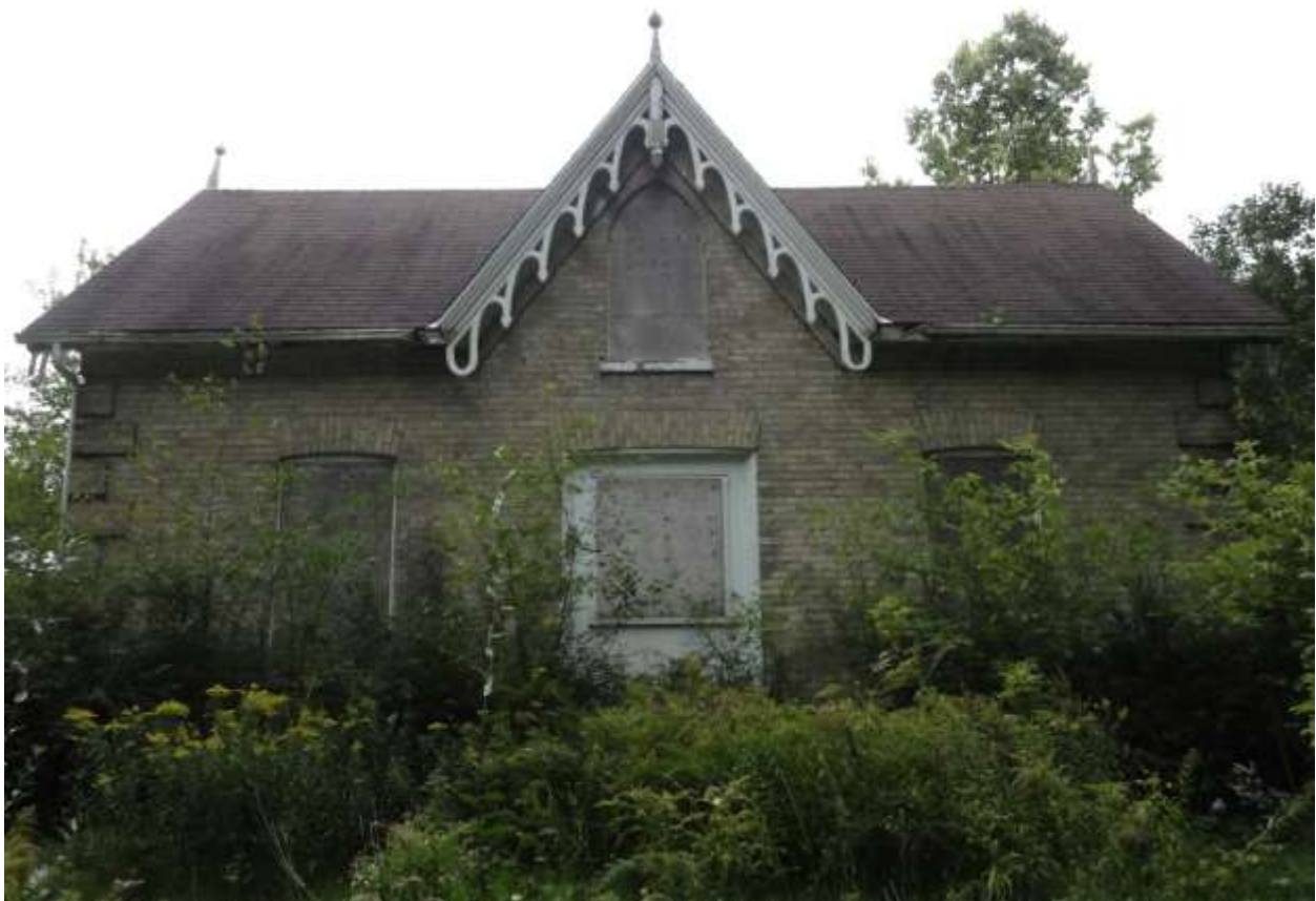
Image 16: View of 1424 Clarke Road, front façade – north facing (2016-09-29).
