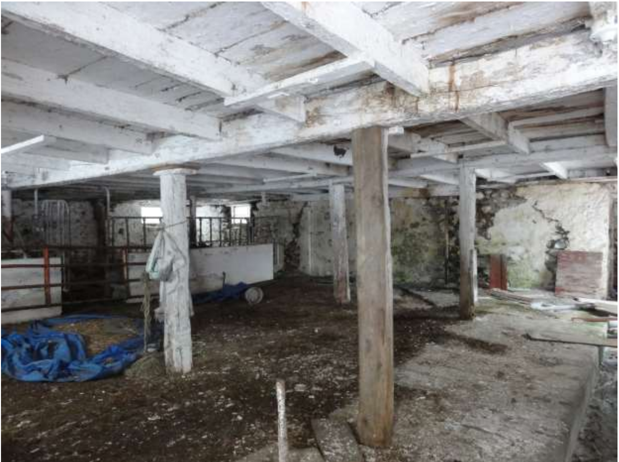
Image 10: View of lower section of barn, stable area (2019-02-14).
