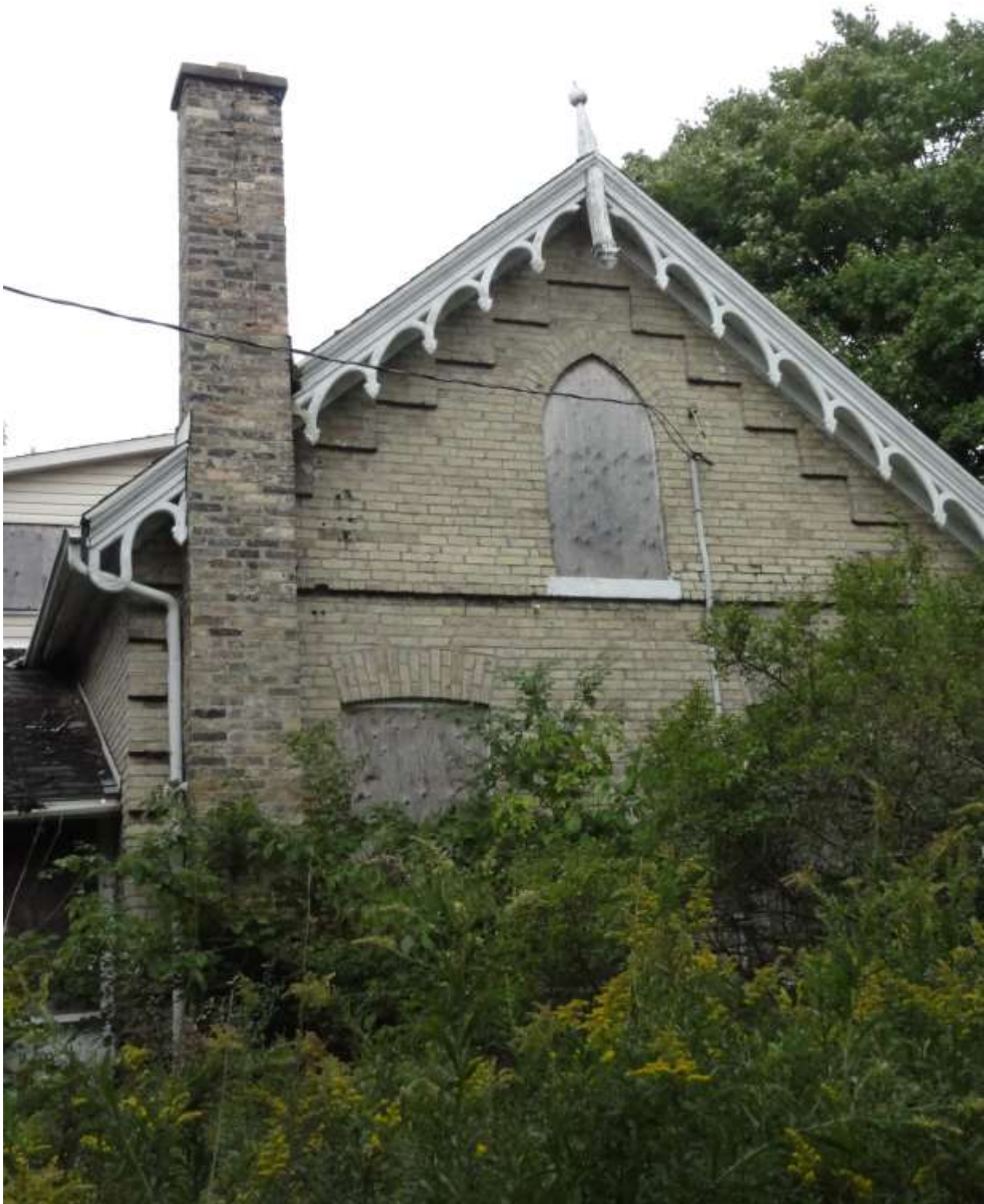
Image 17: View of 1424 Clarke Road, elevation – east facing (2016-09-29).
