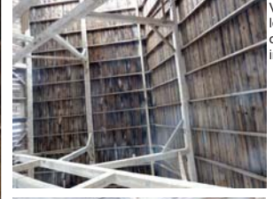
View looking up of barn interior
