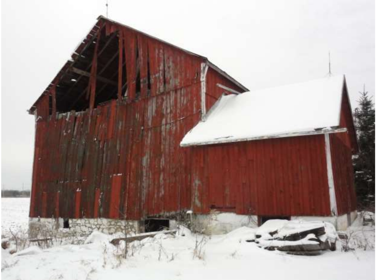
Image 3: View of the barn and addition, east face (2019-02-14).
