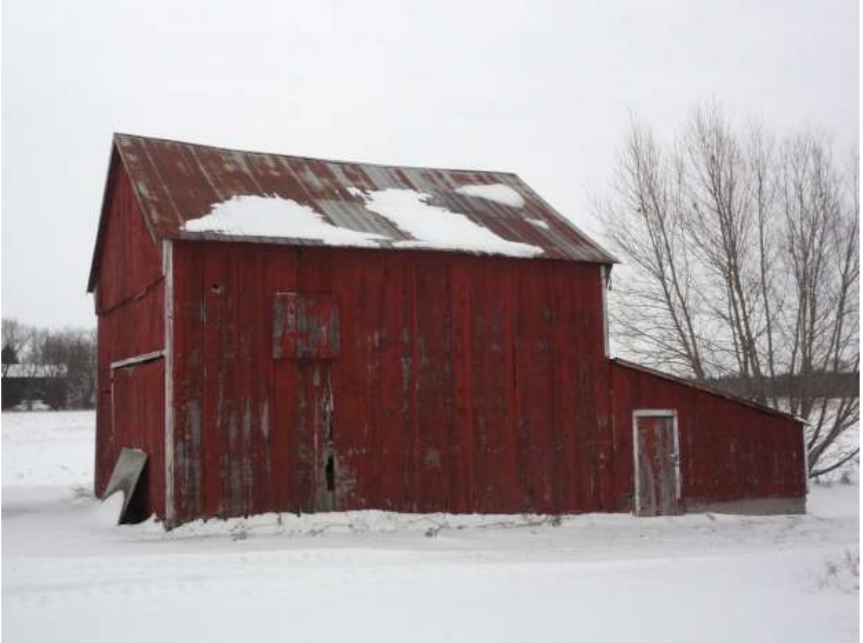
Image 7: View of drive shed (2019-02-14)
