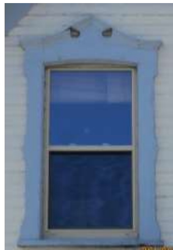
Image 6. Window Trim, 429 William Street, February 2019
